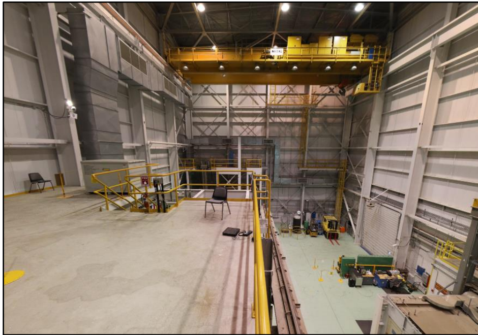
Figure 2.3-4. TREAT Mobile Microreactor Fueling Area
