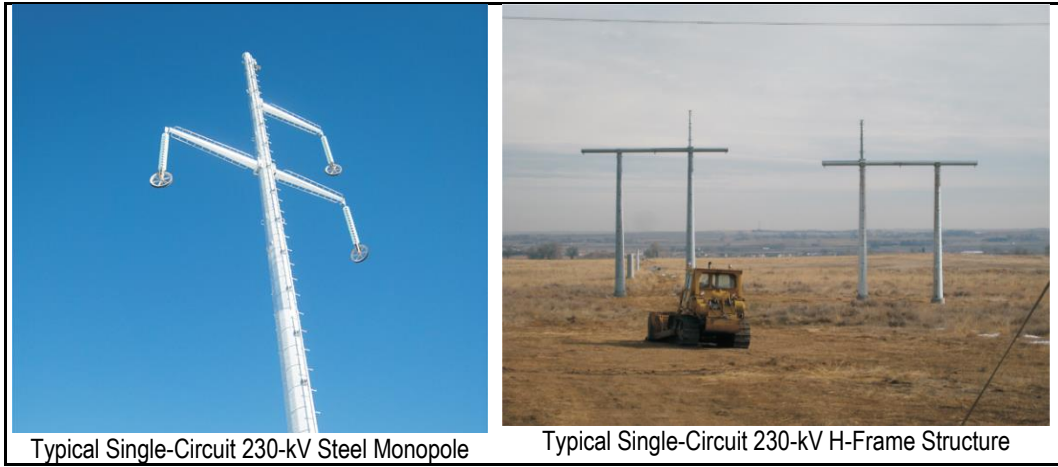
Figure 2-2 Typical Transmission Line Structures
