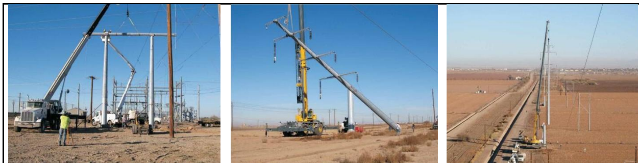
Figure 2-5 Typical Construction of Transmission Line Structures
