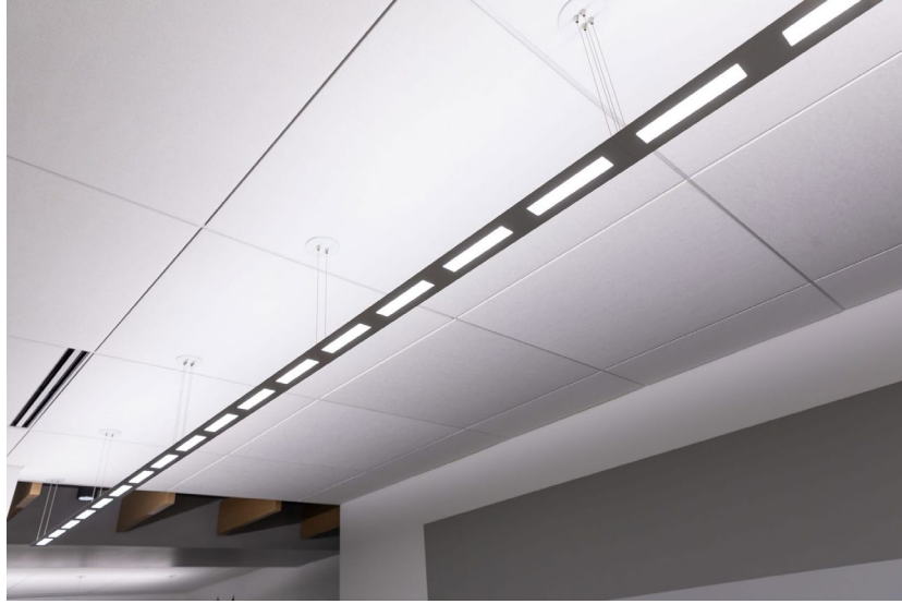
Figure 2.12 Example of white OLED panels integrated into a linear light fixture. [12]
