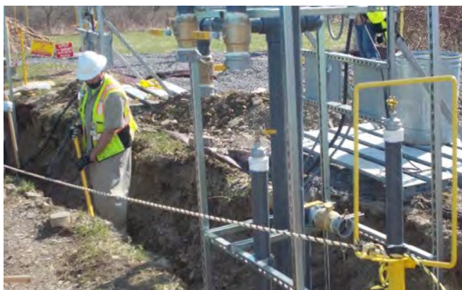
Crews install a robust water management system in preparation for MPPB demolition.
