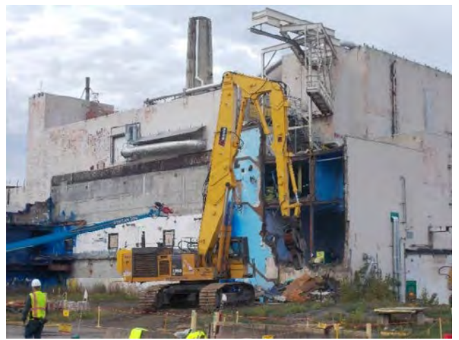
A large excavator is used to remove the west wall for continued deactivation work inside the Acid Recovery Cell.
