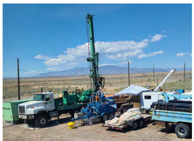
Crews drill a new well near Test Area North at the INL Site.
