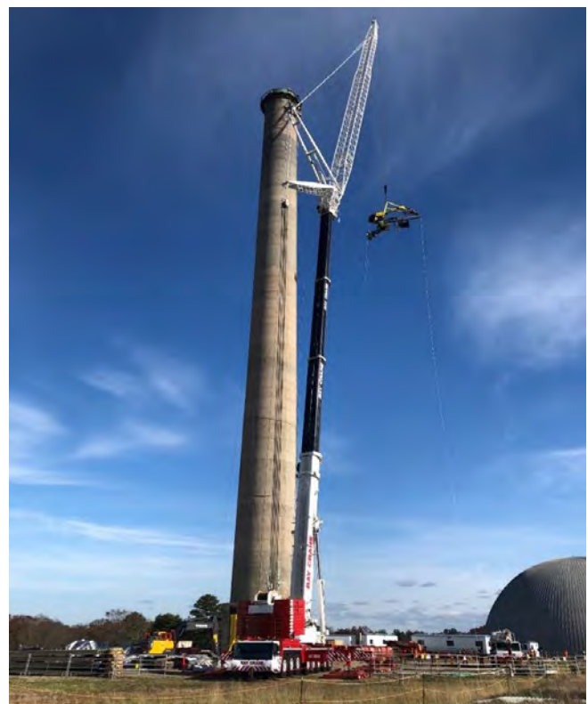
A patented concrete chimney demolition system called the MANTIS is being lifted by crews to the top of the exhaust stack.
