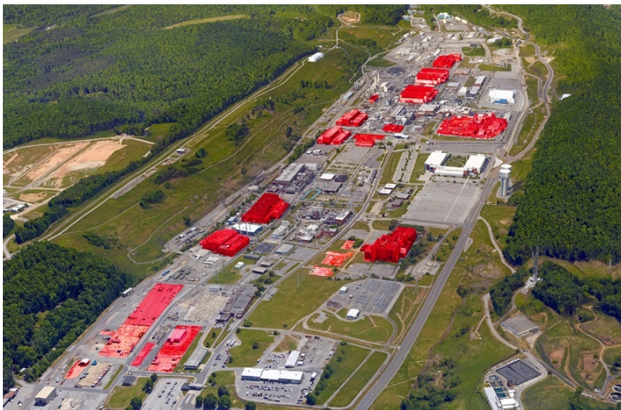
Facilities to address at Y-12
