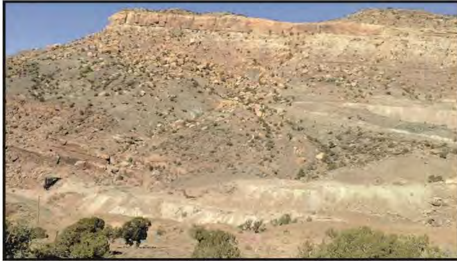
Figure 9: North overview of the Burro Tunnel. The tunnel portal and its ore bin are at far lower left and are largely original. The waste rock bench extending to the right from the ore bin, in the photo's lower left quarter, predates 1970, and retains its original footprint, profile, and surfaces. The tunnel, ore bin, and pre-1970 bench are contributing, and among the most visible elements from public vantage points. The large waste rock bench extending to the right from photo-center post-dates 1970 and was bulldozed after deposition. It remains uncertain how much of the right bench is original and undisturbed. It can be observed that the flanks appear different in character from all the site's other waste rock dumps. The flanks of the site's other dumps consist of fine material deposited by underground haul vehicles, and later furrowed by erosion. In contrast, the flanks of the right bench are a mix of coarse cobbles and boulders deposited by large construction equipment, rarely used at period mines. Given the uncertainty of origin, difference in content and appearance, and recent age (less than fifty years), the right bench is non-contributing and is proposed for removal in the current sediment control project. All other features fifty years and older at the Burro Tunnel will be left intact.
