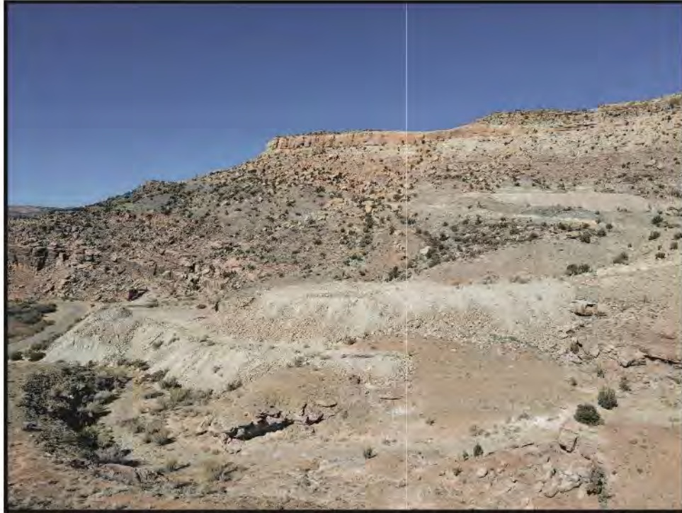
Figure 10: Northwest overview of the Burro Tunnel. The tunnel portal and ore bin are visible at center-left. The waste rock bench also at center-left pre-dates 1970 and is original and contributing. The waste rock bench extending across photo-center post-dates 1970 and is uncertain in origin, possibly reworked with heavy equipment. Note that the flanks are different from the mine's other waste rock dumps, consisting of cobbles and boulders too large for the haul vehicles used when the mine operated. The bench is non-contributing and proposed for removal in the current sediment control project. Note that the left toe of the pre-1970 bench fronts the floor of Burro Gulch, where erosion incised a channel. Storm runoff has calved off portions of the toe, which are to be armored with riprap boulders buried with waste rock for an original appearance.
