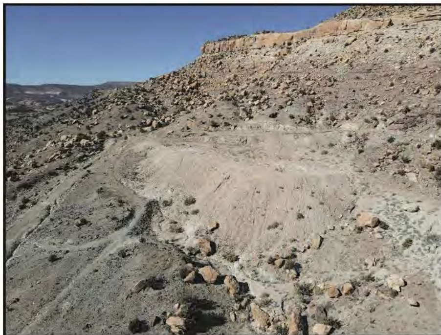
Figure 4: Northwest overview of Burro No. 3 complex, marked by a large waste rock pad. The top-surface was reclaimed decades ago, but the pad still exhibits its original footprint and profile. In a broad sense, the pad is a contributing element of the landscape because from afar, it appears very similar to the original waste rock formation. However, the top-surface is a non-contributing portion because of disruption from reclamation. Relative to the size of the pad and broad scale of the landscape, the reclamation is minor but imposes some cumulative effects. Overall, the pad is a major landscape feature, and will be avoided by the current sediment control project.
