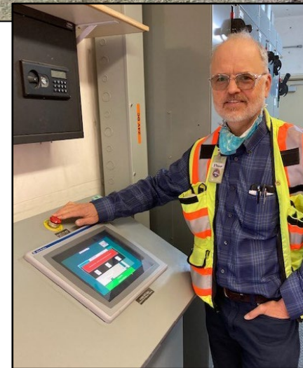
Vapor Vacuum System being shut down to begin OCVZ rebound test
