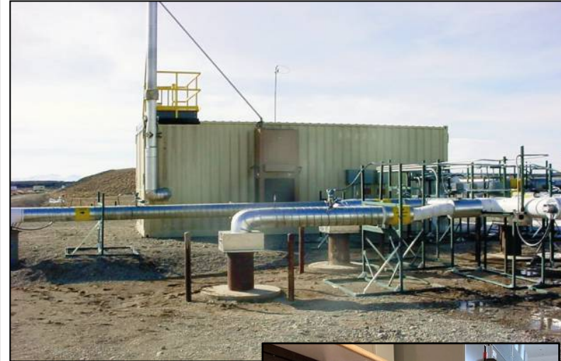
Vapor Vacuum Extraction Treatment System extracts VOCs from the vadose zone beneath the SDA
