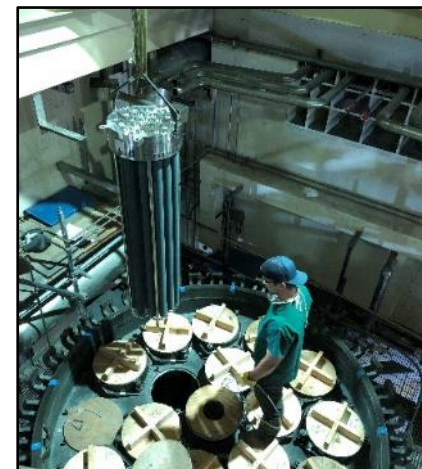
Modified PGF ceramic filter bundles during installation at IWTU
