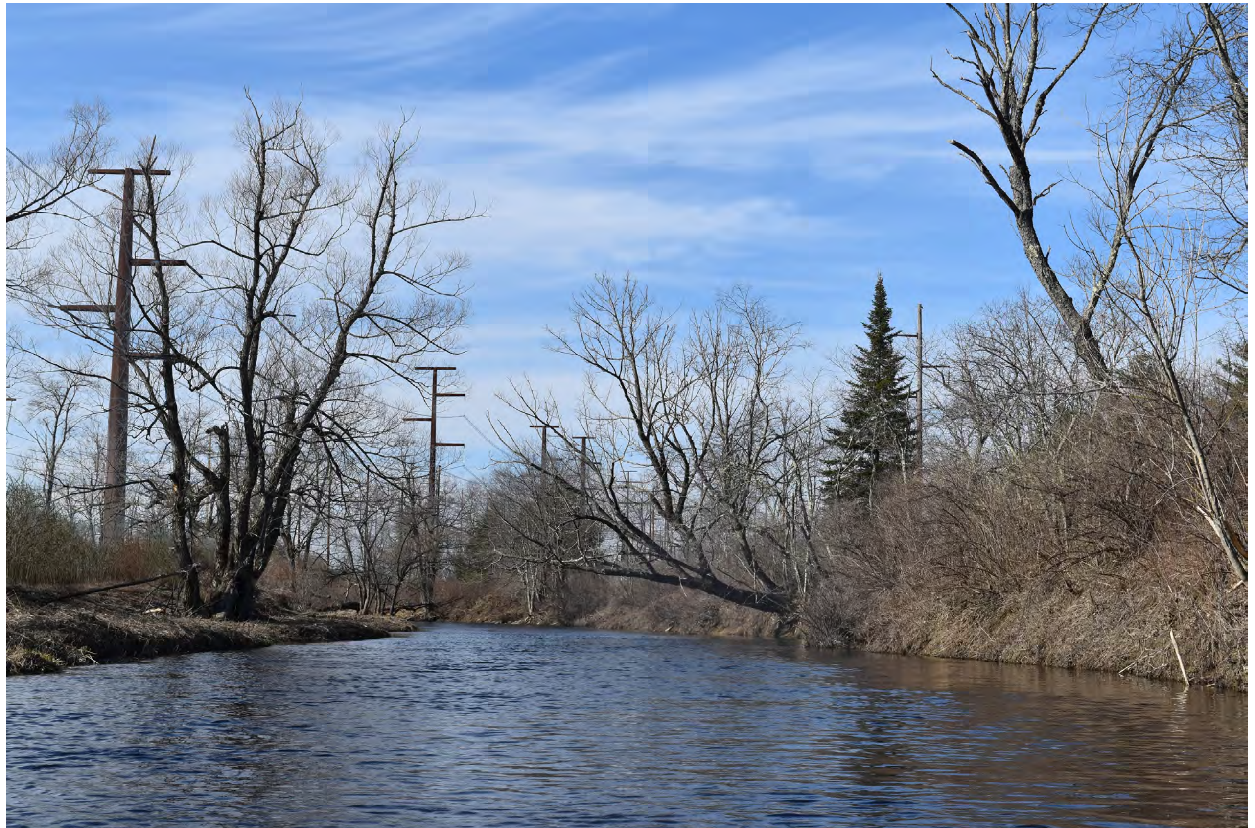
Photosimulation 37D: Normal view looking north from the Sheepscot River in Windsor toward the proposed co-located 345 kV transmission line. Five proposed 345 kV structures and conductors will be visible at distances of 500 to 2,300 feet from this viewpoint. Riparian corridor vegetation will be enhanced with new plantings to contribute to stream bank stability, biofiltration, and visual mitigation.
