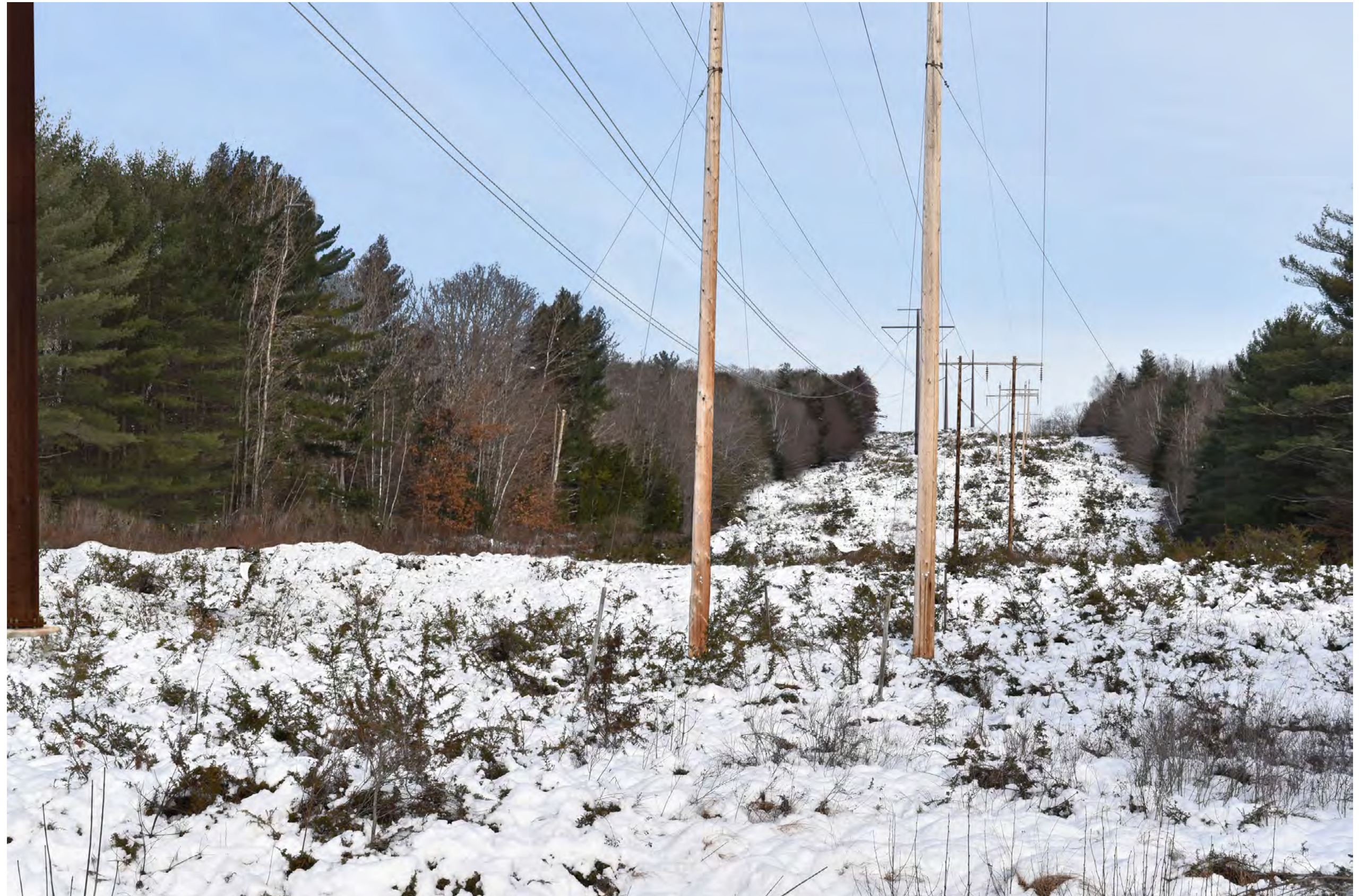
Photosimulation 53A: Normal view looking northeast toward the proposed co-located HVDC transmission line from Route 201 in Moscow. This portion of Route 201 is part of the Old Canada Road National Scenic Byway. The existing 225 ft wide corridor clearing will be widened by 75 ft on the western side (left of corridor in image) to accommodate the proposed HVDC transmission line. Three structures will be visible from this viewpoint.
