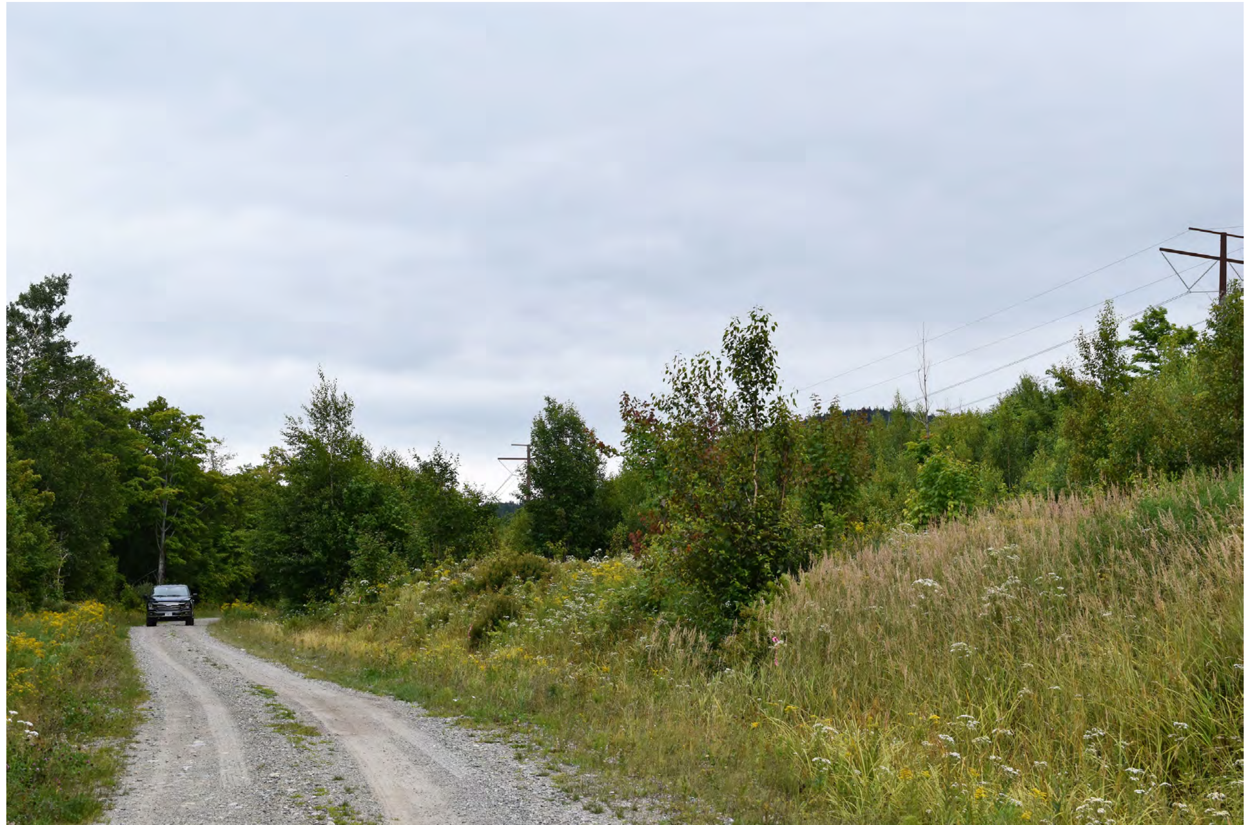
Photosimulation 59A: Normal view looking east from Merrill Strip Road toward the proposed alternative section of the HVDC transmission line in Merrill Strip Township. Two tangent structures (#804 at 104.5 ft and #803 at 111.5 ft), conductors, and shield wires will be visible from this viewpoint. The closest structure (#804) is 610 feet from the viewpoint.
