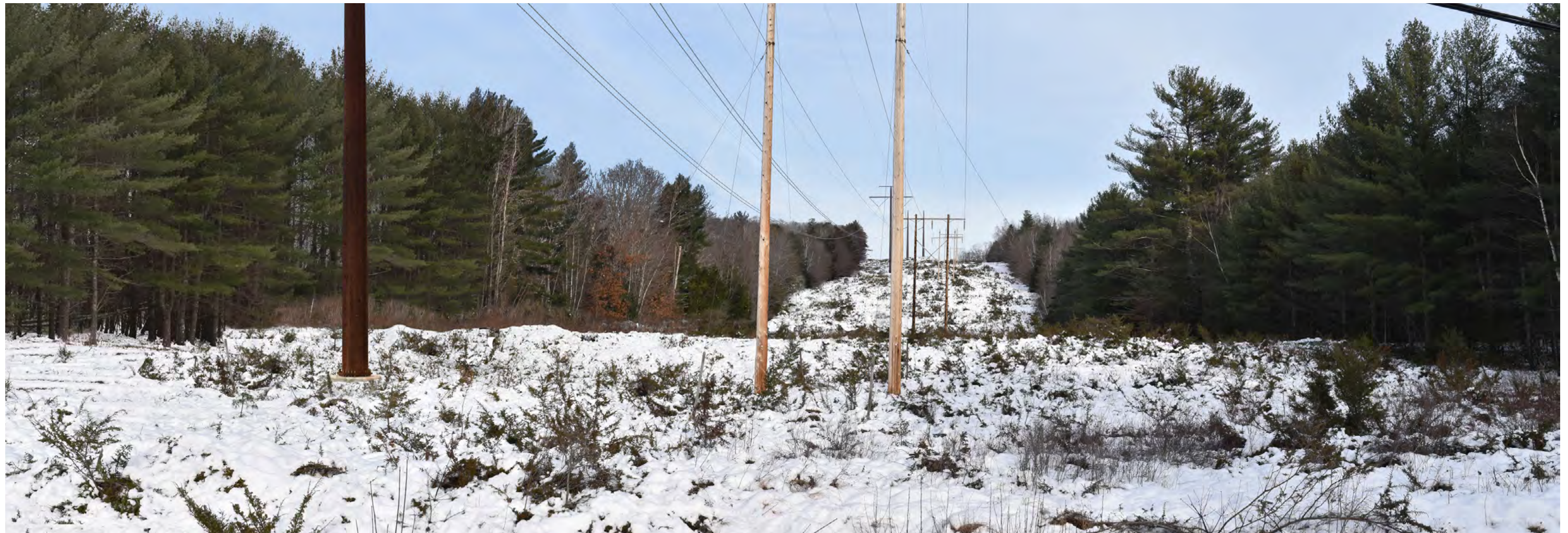
Photosimulation 53: Panoramic view looking from north to east from Route 201 in Moscow toward the proposed co-located HVDC transmission line. This portion of Route 201 is part of the Old Canada Road National Scenic Byway. The existing 225 ft wide corridor clearing will be widened by 75 ft on the western side (left of corridor in image) to accommodate the proposed transmission line. Three structures will be visible from this viewpoint.
