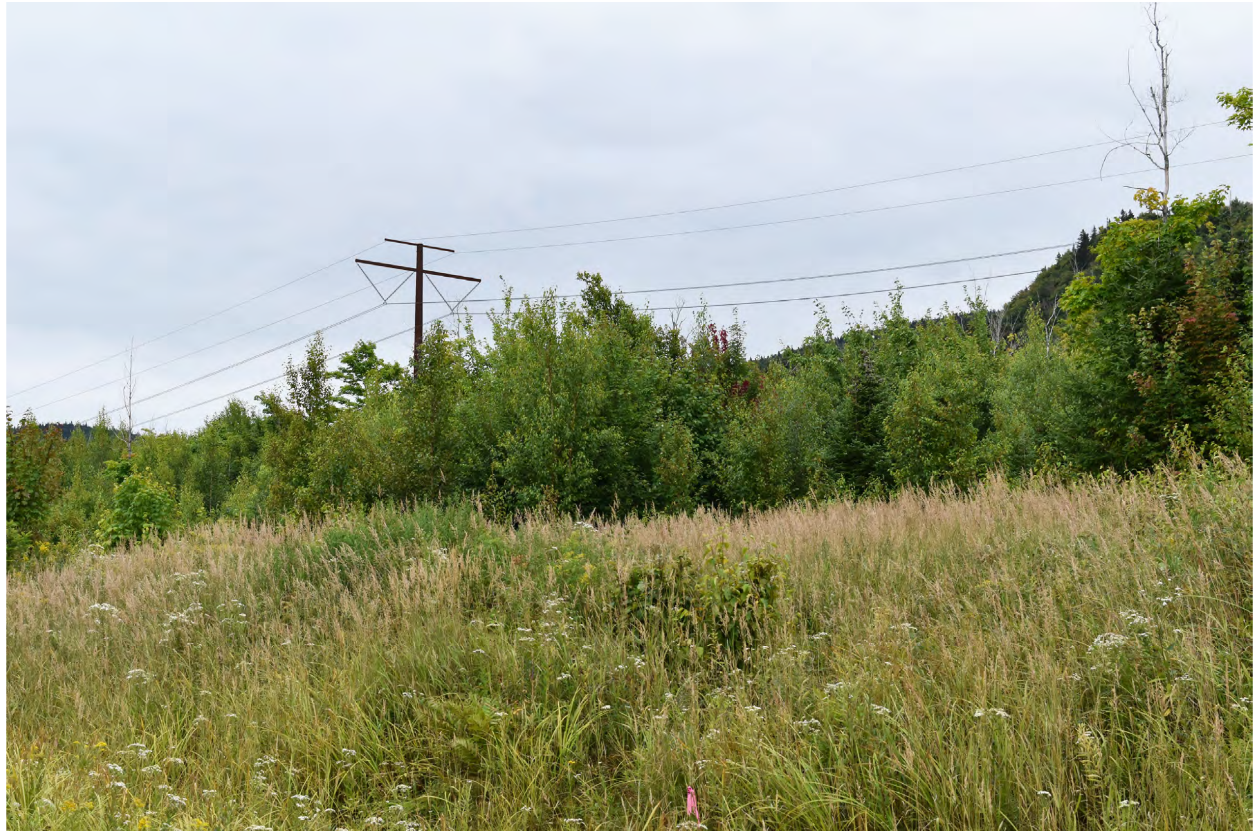
Photosimulation 59B: Normal view looking southeast from Merrill Strip Road toward the proposed alternative section of the HVDC transmission line in Merrill Strip Township. Structure #804 is shown at 104.5 ft in height and located 610 feet from this viewpoint. The conductors and shield wires will be visible.
