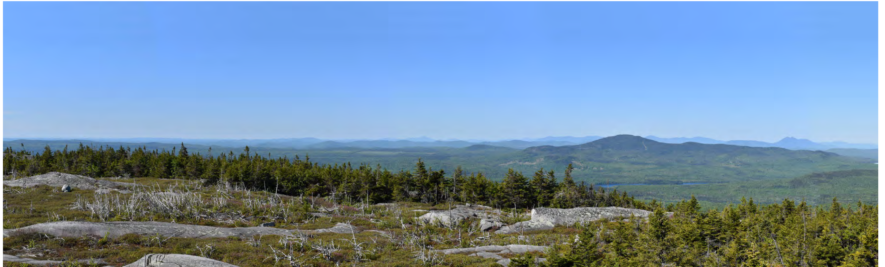
Proposed Conditions: Panoramic view looking from south to west from the summit of Bald Mountain on the Appalachian Trail in Bald Mountain TWP toward the proposed co-located HVDC transmission line. Moxie Mountain is visible on the right side of the image with Baker Pond visible below.
