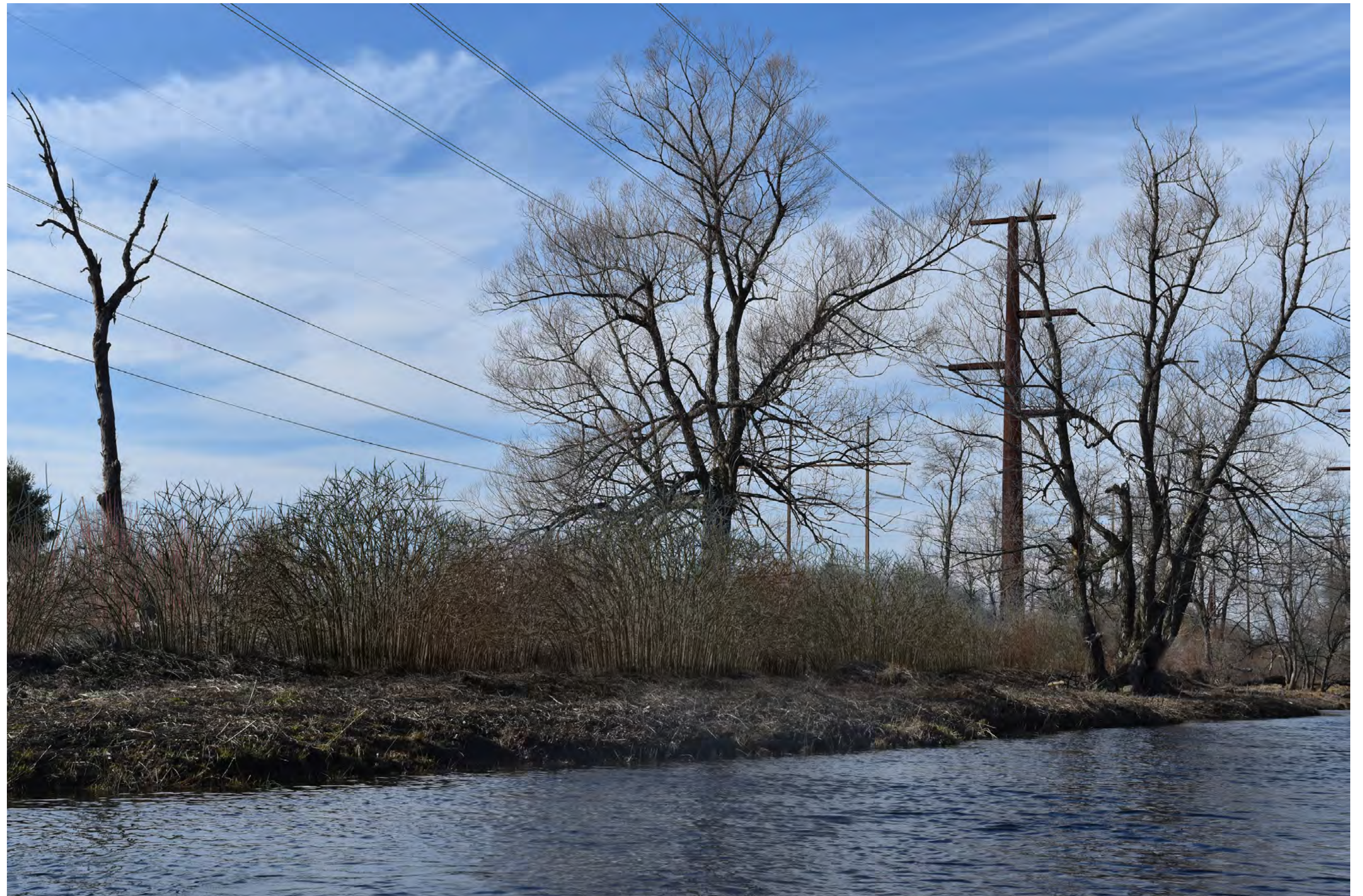
Photosimulation 37A: Normal view looking north from the Sheepscot River in Windsor toward the proposed co-located 345 kV transmission line. Five proposed 345 kV structures and conductors will be visible at distances of 500 to 2,300 feet from this viewpoint. Riparian corridor vegetation will be enhanced with new plantings to contribute to stream bank stability, biofiltration, and visual mitigation.
