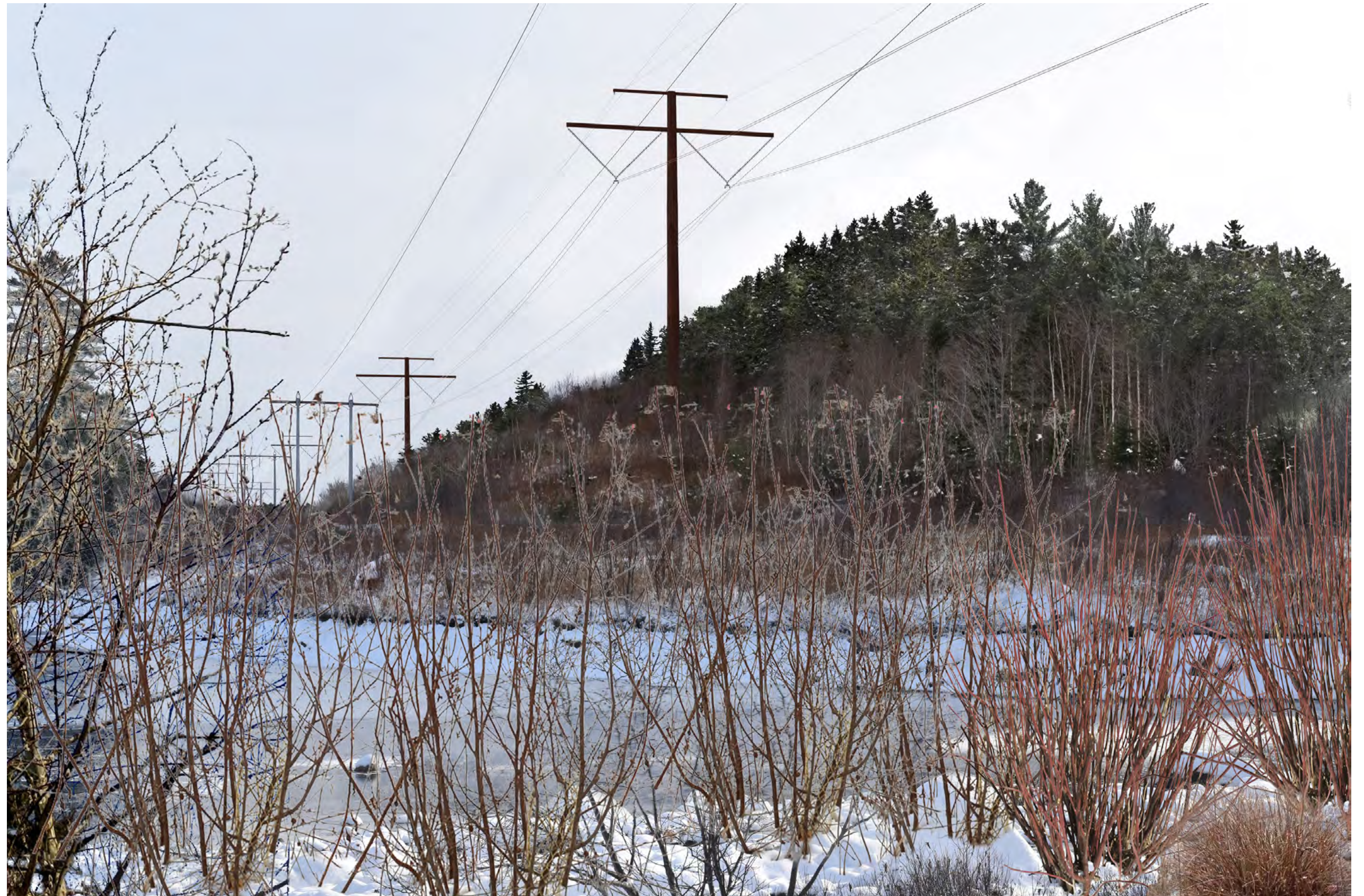
Photosimulation 50A: Normal view looking south on Troutdale Road (private road) looking toward the proposed co-located HVDC transmission line with proposed Joes Hole (Moxie Pond) buffer plantings in the foreground . Over a distance of approximately 4,400' within the vicinity of the Appalachian Trail crossings, tapered vegetation management techniques will be used in both the existing 125' wide transmission line corridor and the proposed 75' widened corridor. Portions of six proposed HVDC structures will be visible from this viewpoint.
