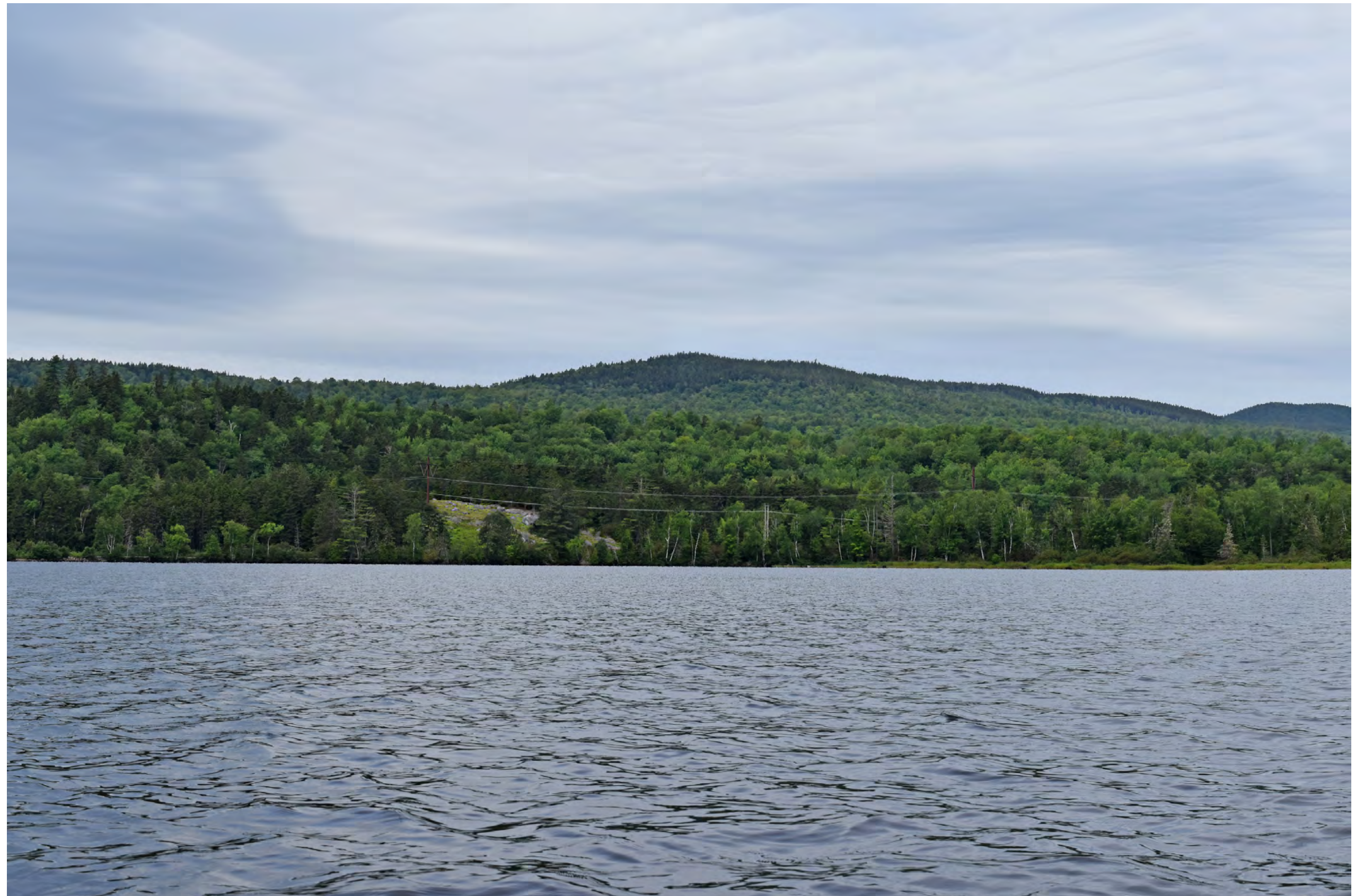
Photosimulation 15A: Normal view looking west from the southern area of Moxie Pond toward the proposed co-located HVDC transmission line. The clearing will be widened by 75' on the western side of the existing 150' wide 115 kv transmission line corridor to accommodate the new HVDC transmission line. One structure and the top of another structure will be visible above the existing transmission line structures and conductors at distances of approximately 2,000 to 2,100 feet.
