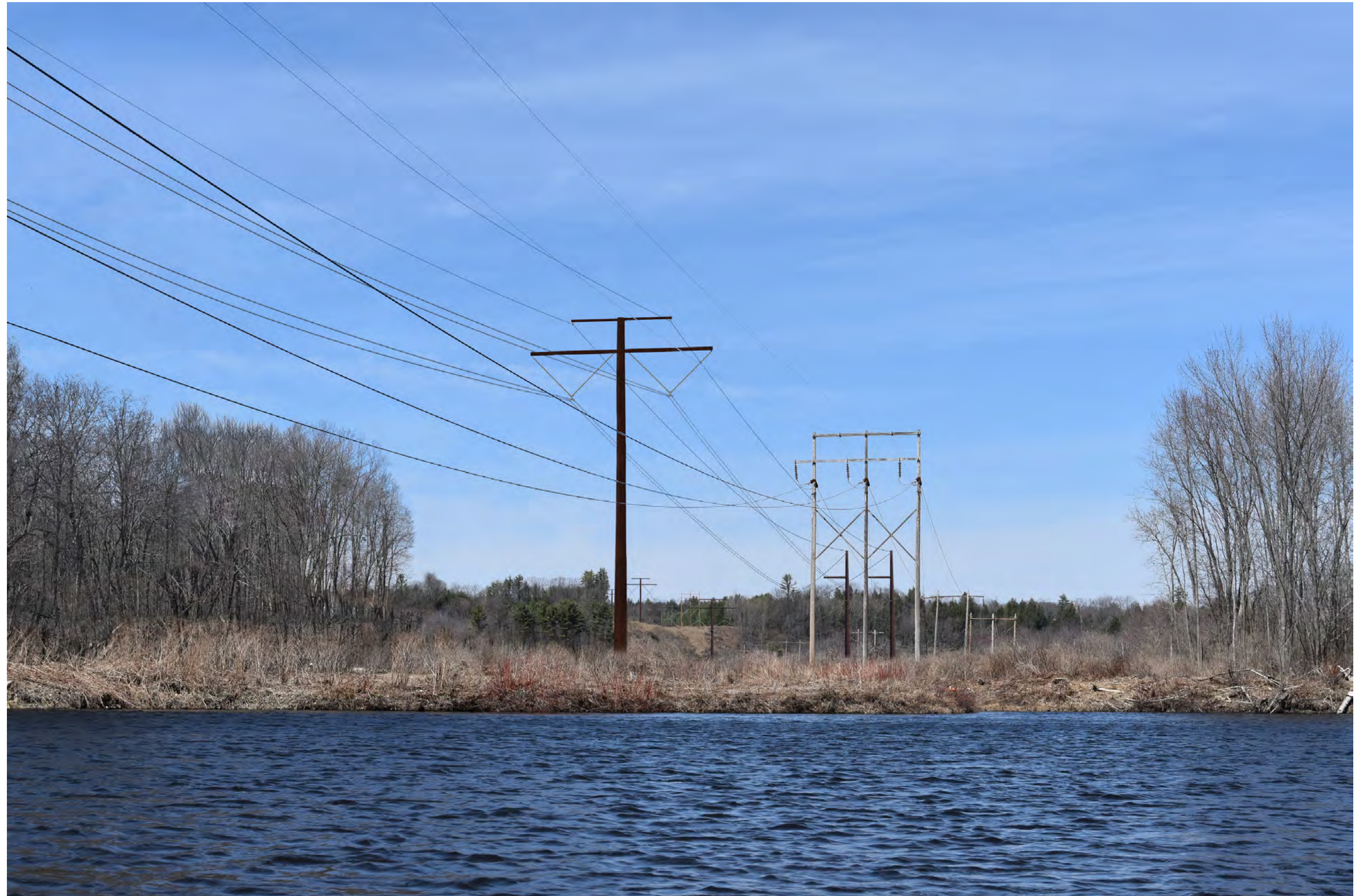
Photosimulation 34: Normal view looking north from the Carrabasset River in Anson toward the proposed co-located HVDC transmission line. The existing 225' wide cleared corridor will be widened by 75' on the western side to accommodate the proposed HVDC transmission line. Five proposed HVDC structures and conductors will be visible at distances of 540 feet to 3,800 feet from this viewpoint.
