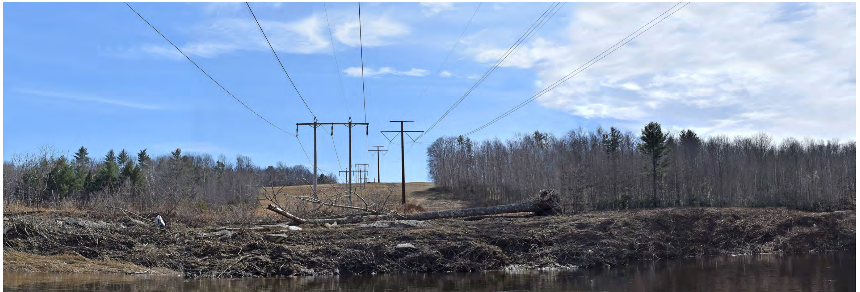
Photosimulation 35: Panoramic view looking south to west from the Sandy River in Farmington toward the proposed co-located HVDC transmission line. The existing 225' wide cleared corridor will be widened by 75' on the western side to accommodate the proposed HVDC transmission line. Three proposed HVDC structures and conductors will be visible at distances of 805 to 2,450 feet from this viewpoint.
