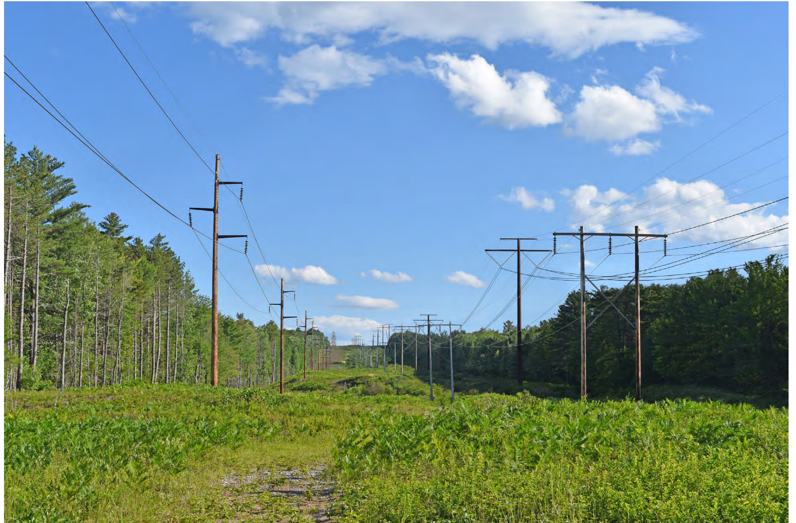
Photosimulation 23A: Normal view looking south from an access road (off Church Hill Road) crossing the existing transmission line within the State Park toward the proposed co-located HVDC transmission line. The existing 225' corridor clearing will be widened by 75' on the western side to accommodate the new transmission line.
