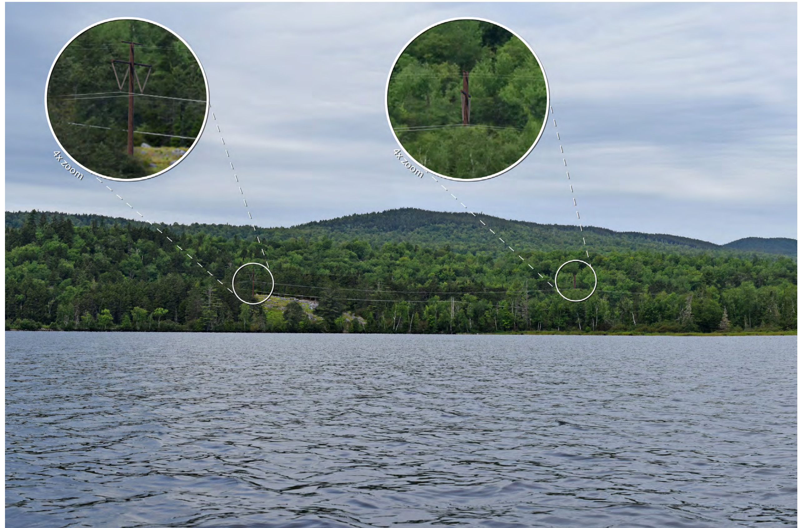
Photosimulation 15A: Normal view looking west from the southern area of Moxie Pond toward the proposed co-located HVDC transmission line. The clearing will be widened by 75' on the western side of the existing 150' wide 115 kv transmission line corridor to accommodate the new HVDC transmission line. One structure and the top of another structure are visible above the existing transmission line structures and conductors at distances of approximately 2,000 to 2,100 feet.
