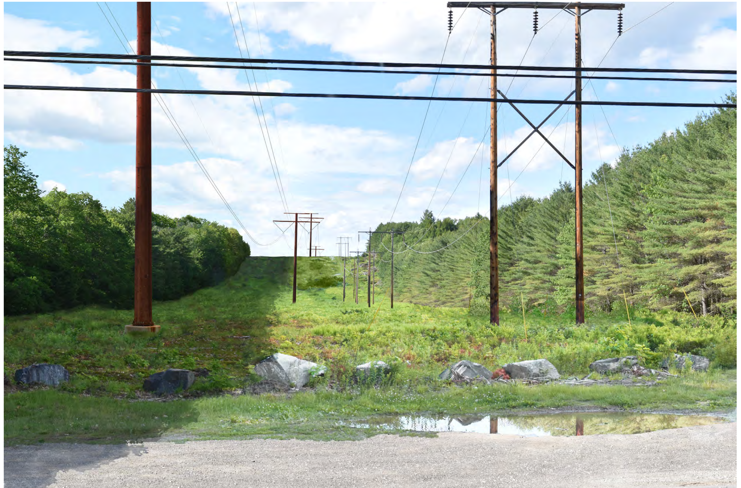
Photosimulation 21A: Normal view looking north from Route 8 (Solon Rd) toward the proposed co-located HVDC transmission line. The existing 150' wide cleared corridor will be widened by 75' on the western side to accommodate the proposed HVDC transmission line. Four of the proposed HVDC structures and conductors will be visible from this viewpoint.
