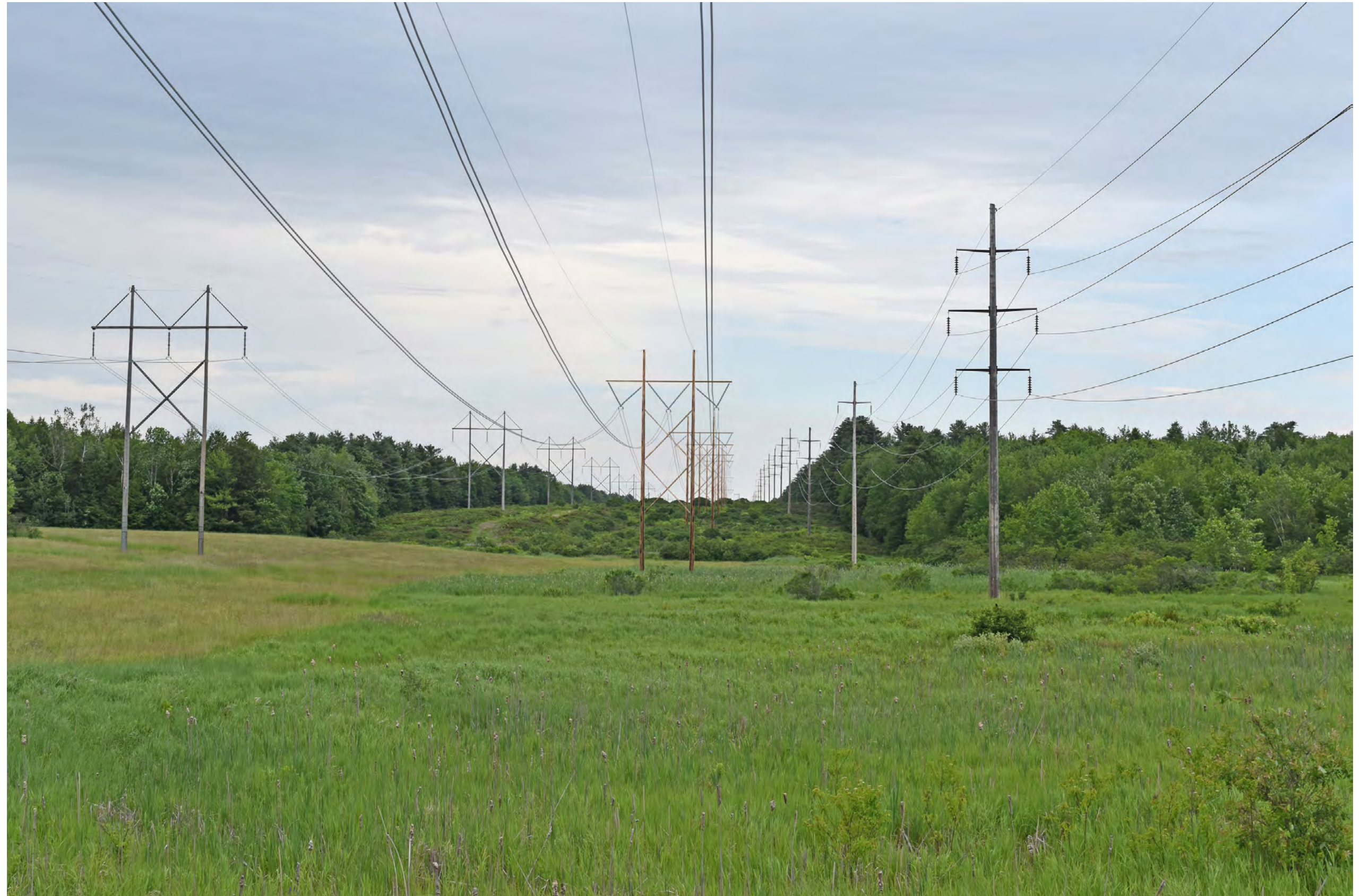
Photosimulation 28A: Normal view looking from north to northeast from Route 27 toward the proposed co-located 345 kV transmission line. The proposed 345 kV transmission line will be located in between the existing 115 kV and 345 kV transmission lines. Seven structures and conductors will be visible from this viewpoint.
