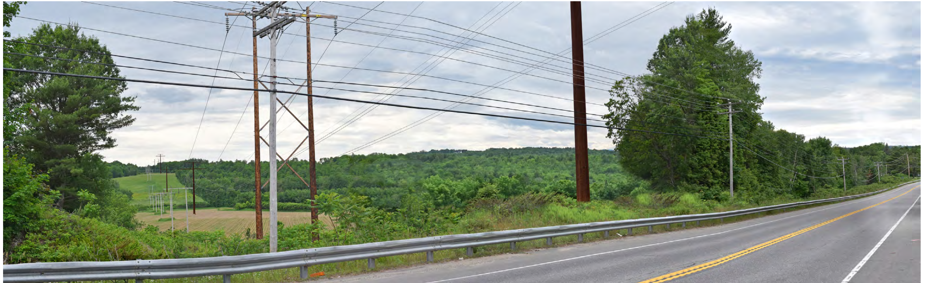
Photosimulation 22: Panoramic view looking from south to west from Route 2 in Farmington toward the proposed co-located HVDC transmission line. The existing 225' wide cleared corridor will be widened by 75' on the western side to accommodate the proposed HVDC transmission line. Six of the proposed HVDC structures and conductors will be visible from this viewpoint. See Appendix B: Study Area photographs for additional images.
