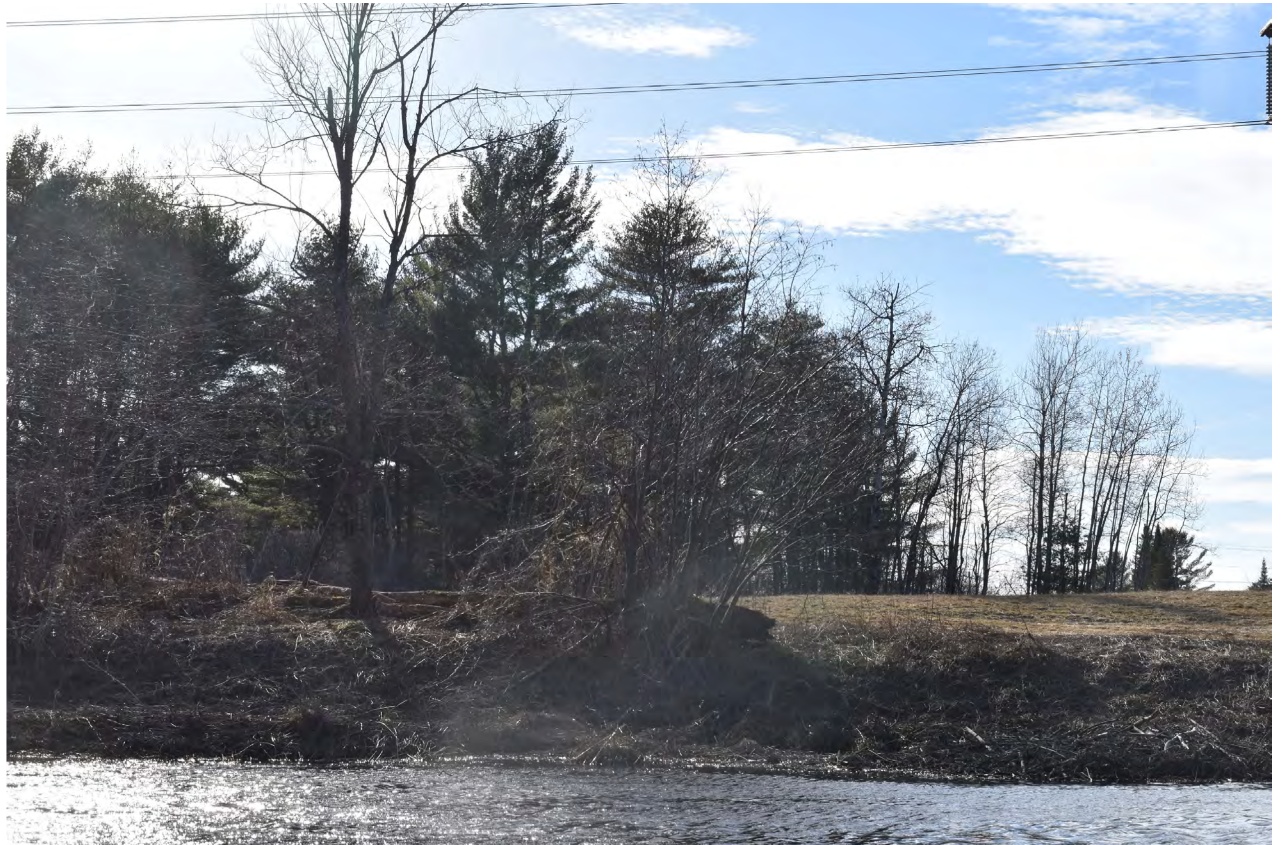
Existing Conditions 36B: Normal view looking west from the West Branch Sheepscot River in Windsor toward the existing 345 kV transmission line.
