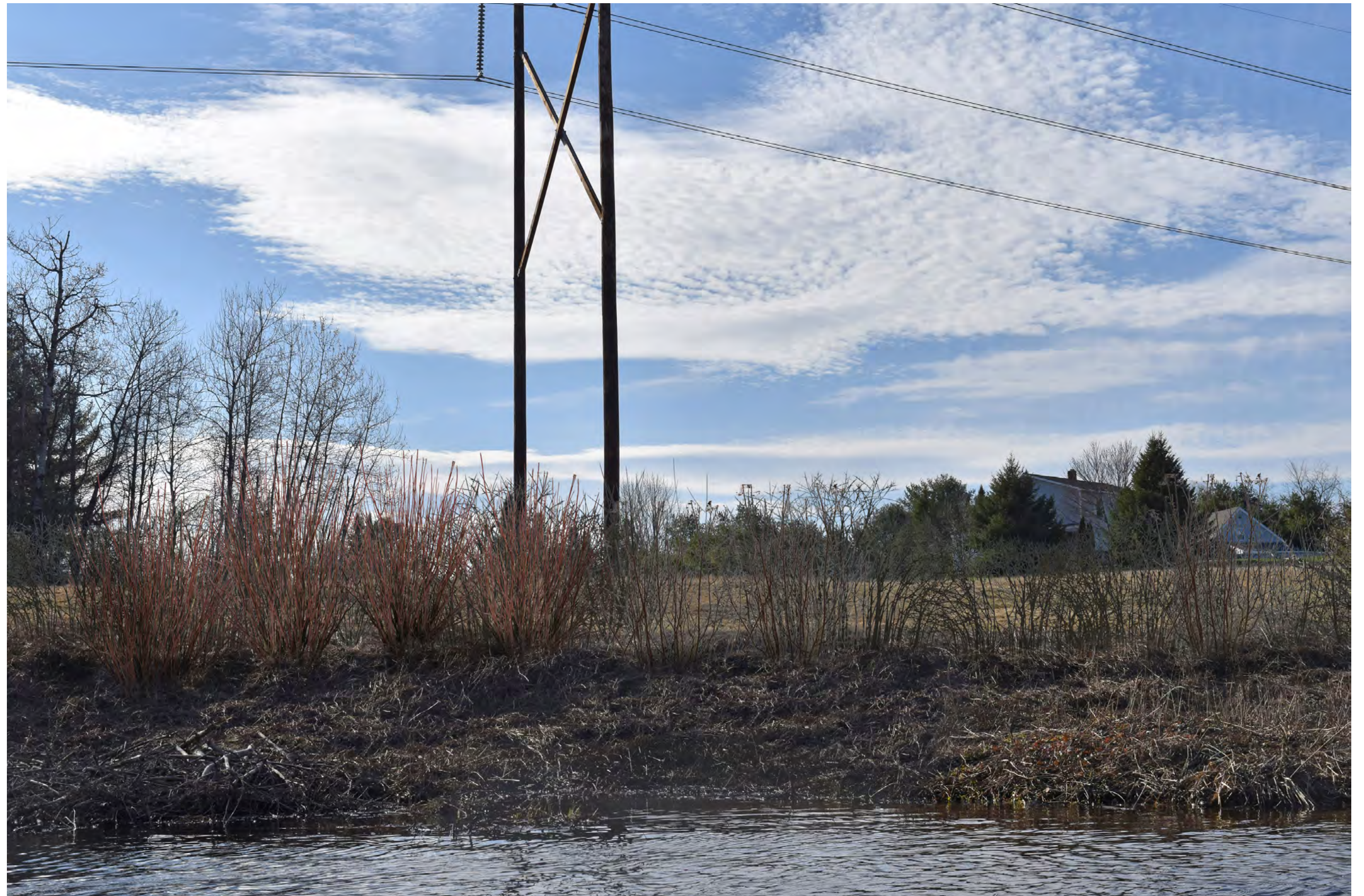
Photosimulation 36A: Normal view looking west from the West Branch Sheepscot River in Windsor toward the proposed co-located 345 kV transmission line. Based on the revised (Rev1) design of the co-located 345 kV transmission line, no proposed structures will be visible when looking in this direction. Riparian corridor vegetation will be enhanced with new plantings to contribute to stream bank stability, biofiltration, and visual mitigation.
