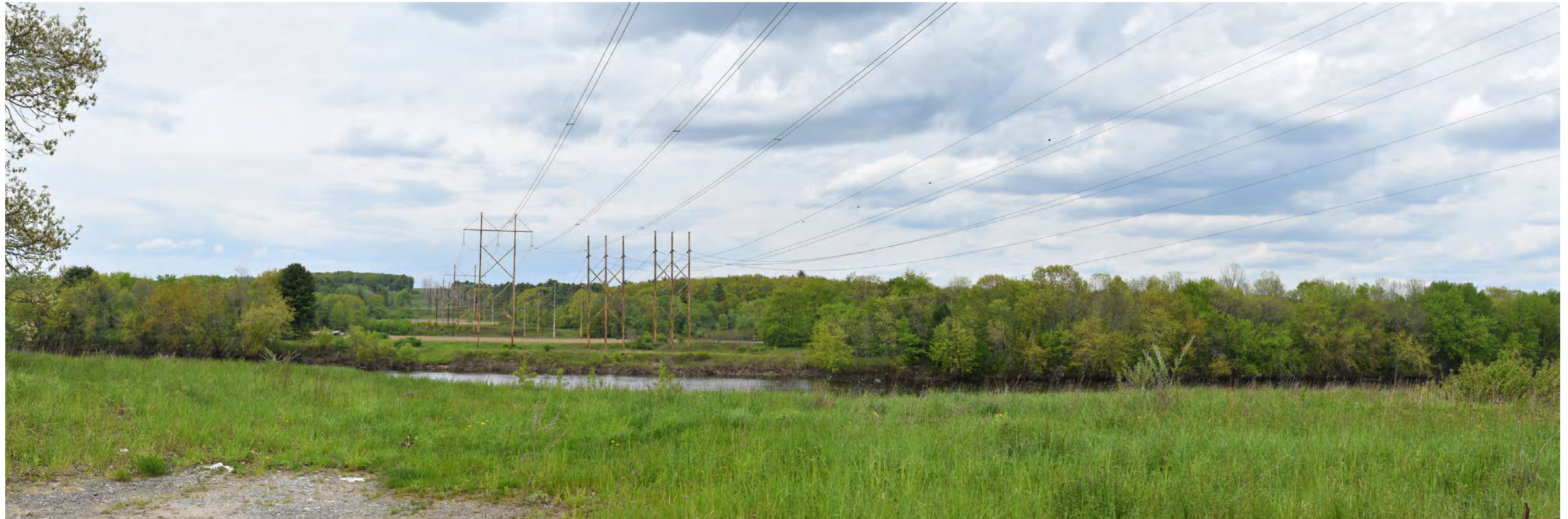
Photosimulation 25: Panoramic view looking from north to northeast from Riverside Drive / Route 136 in Auburn over the Androscoggin River toward the proposed Sections 62 & 64 Rebuild transmission lines. The wood H-frame 115 kV structures will be replaced. The existing single pole structures will be relocated / replaced as necessary. All of the rebuilt structures will be made of wood. No additional tree removal will be required. Approximately 20 new structures will be visible from this viewpoint. See Appendix B: Study Area Photographs for additional images.
