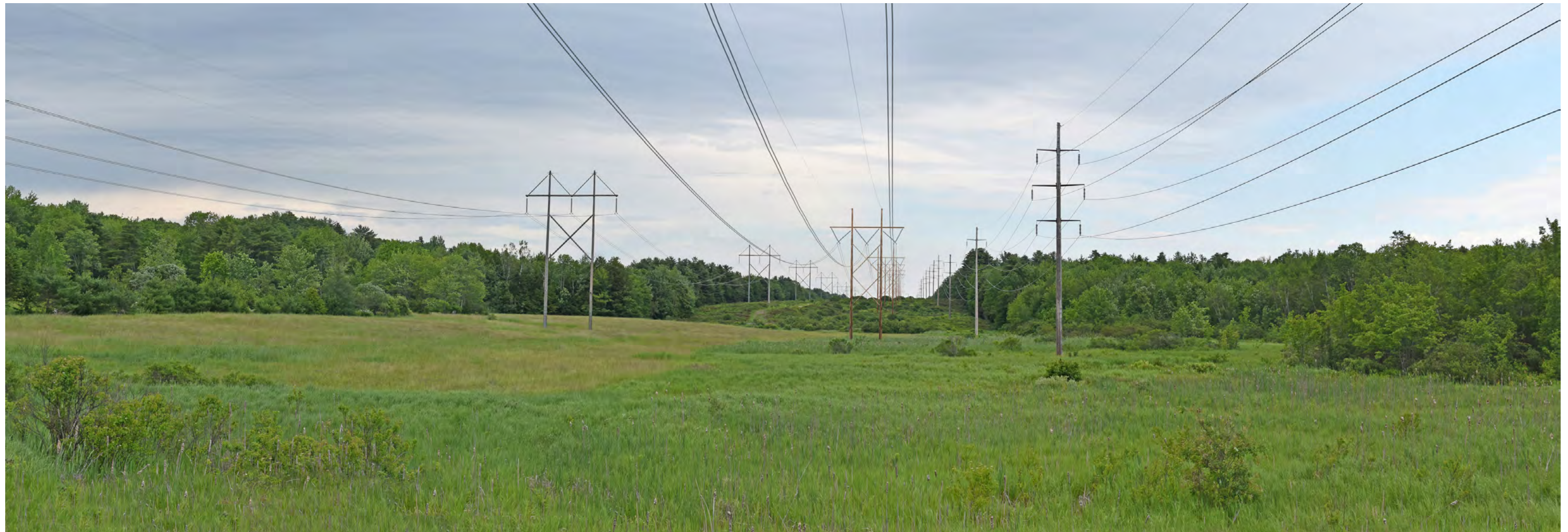
Photosimulation 28: Panoramic view looking from north to northeast from Route 27 toward the proposed co-located 345 kV transmission line. The proposed 345 kV transmission line will be located in between the existing 115 kV and 345 kV transmission lines. A proposed structure will be located directly adjacent to this viewpoint. Seven structures and conductors will be visible from this viewpoint. See Appendix B: Study Area Photographs for additional images.
