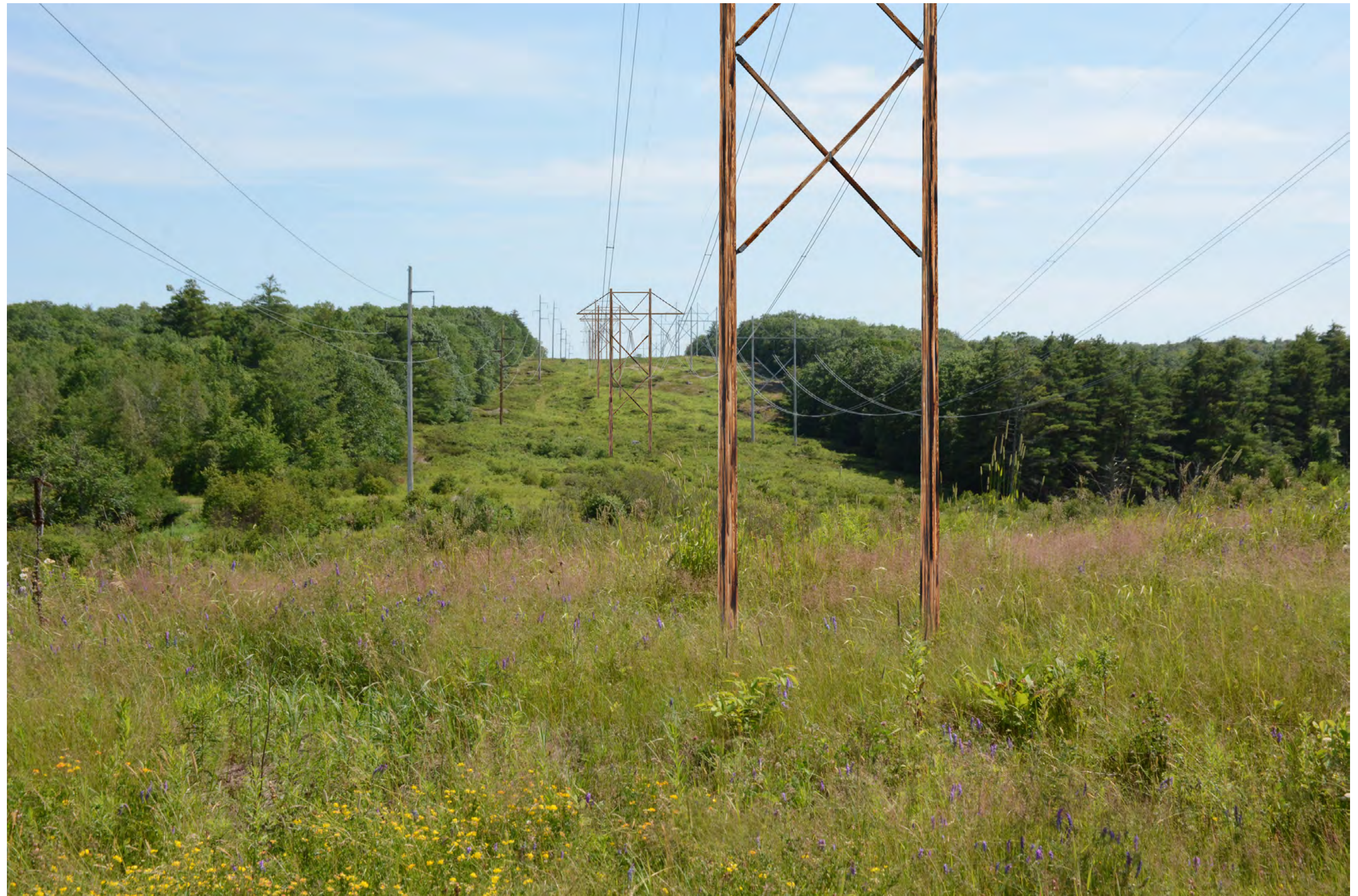
Photosimulation 29A: Normal view looking from southeast to southwest from Route 194 toward the proposed co-located 345 kV transmission line. Seven structures and conductors will be visible from this viewpoint. The proposed 345 kV transmission line will be located in between the existing 115 kV and 345 kV transmission lines.
