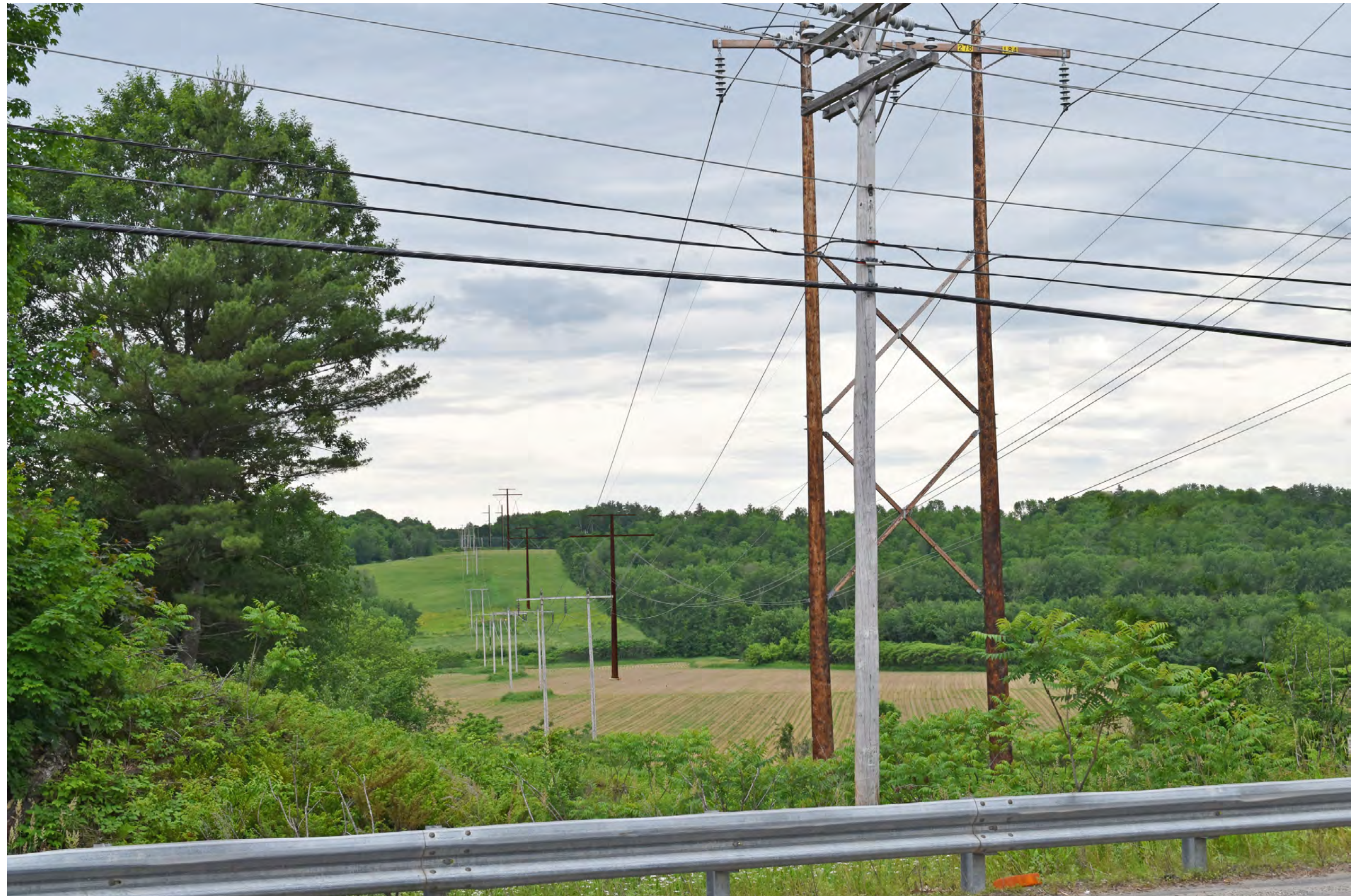
Photosimulation 22A: Normal view looking from southwest from Route 2 toward the proposed co-located HVDC transmission line. The existing 225' wide cleared corridor will be widened by 75' on the western side to accommodate the new HVDC transmission line. Five of the proposed HVDC structures and conductors will be visible from this viewpoint.
