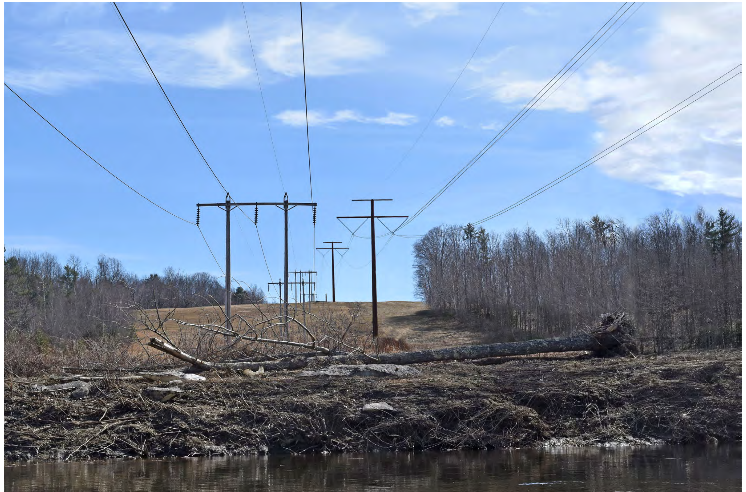
Photosimulation 35B: Normal view looking south from the Sandy River in Farmington toward the proposed co-located HVDC kV transmission line. The existing 225' wide cleared corridor will be widened by 75' on the western side to accommodate the proposed HVDC transmission line. Three proposed HVDC structures and conductors will be visible at distances of 805 to 2,450 feet away from this viewpoint.
