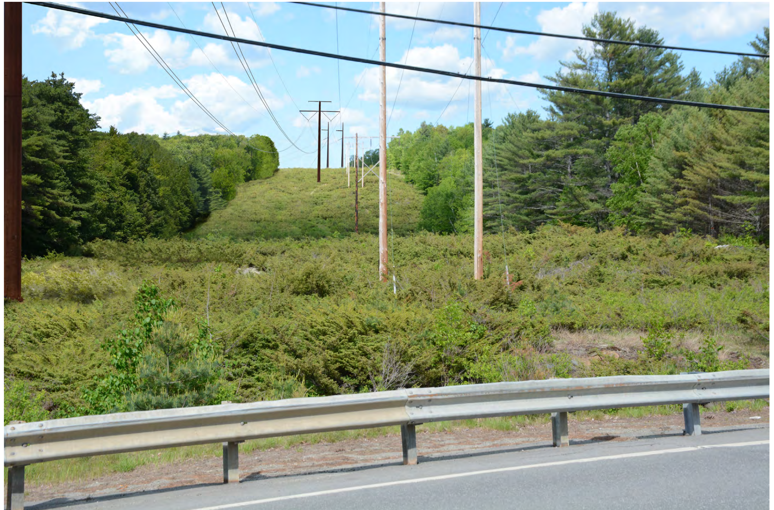
Photosimulation 19A: Normal view looking east from Route 201 in Moscow toward the proposed co-located HVDC transmission line. This portion of Route 201 is part of the Old Canada Road National Scenic Byway. The existing 225' wide corridor clearing will be widened by 75' on the western side (left of corridor in image) to accommodate the proposed HVDC transmission line. Three structures will be visible from this viewpoint.
