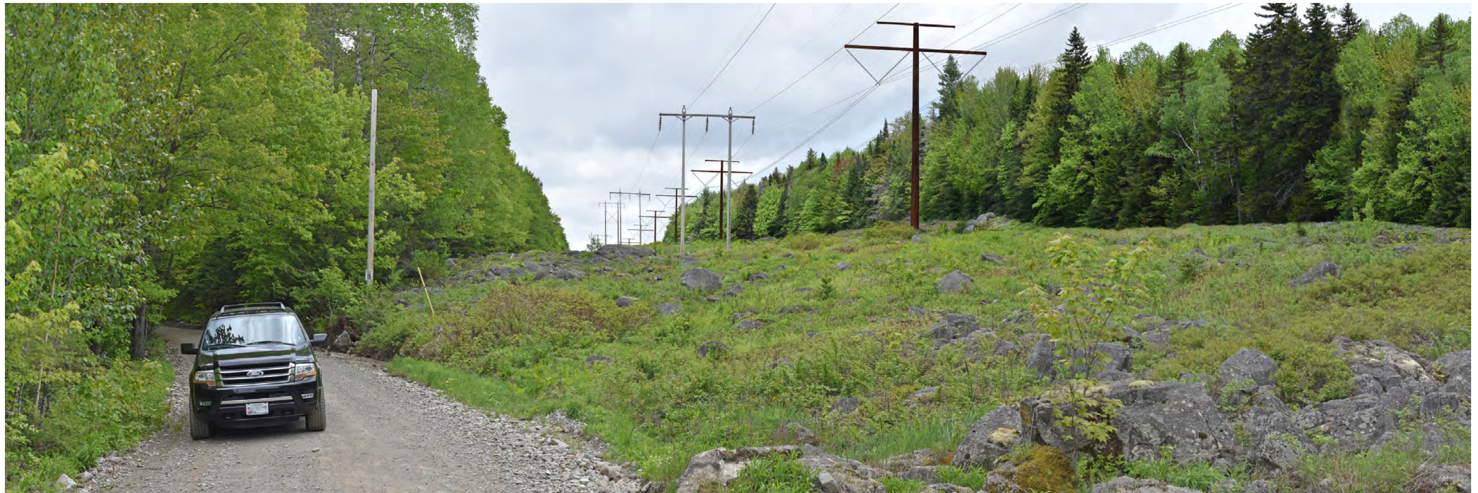
Photosimulation 18: Panoramic view looking southeast to south from Troutdale Road in The Forks Plt. toward the proposed co-located HVDC transmission line. Troutdale Road is located within the existing 115 kV transmission line corridor for approximately 1,000 feet. The existing 150' wide corridor clearing will be widened by 75' on the western side to accommodate the new transmission line. Two HVDC transmission structures will be visible looking to the southeast, and four looking to the northwest. See Appendix B: Study Area Photographs for additional images.
