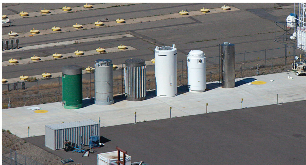
Dry storage casks at the Idaho Nuclear Technology and Engineering Center at INL.
