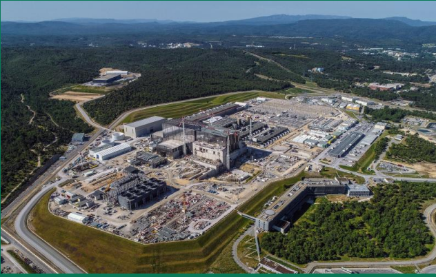
International Thermonuclear Experimental Reactor (ITER) site, May 2020
