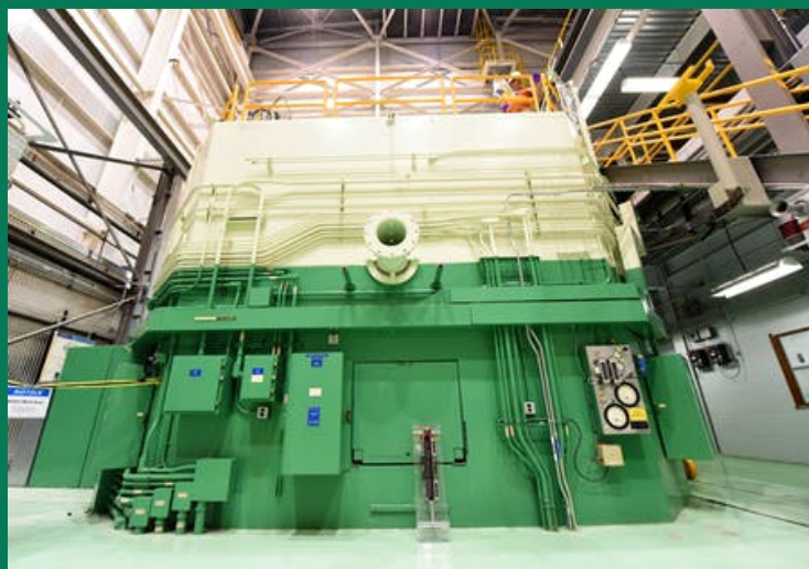
Idaho National Laboratory's TREAT provides transient testing of nuclear fuels and materials.
