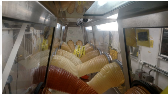
Exhibit 3. Manipulator repair glovebox refurbishment - interior view.
