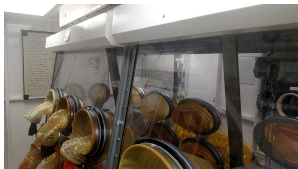
Exhibit 4. Manipulator repair glovebox refurbishment - exterior.
