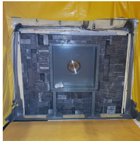
Exhibit 7. Small cask transfer installation – inside tent.
