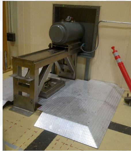
Exhibit 6. Small cask transfer station installation – installed.
