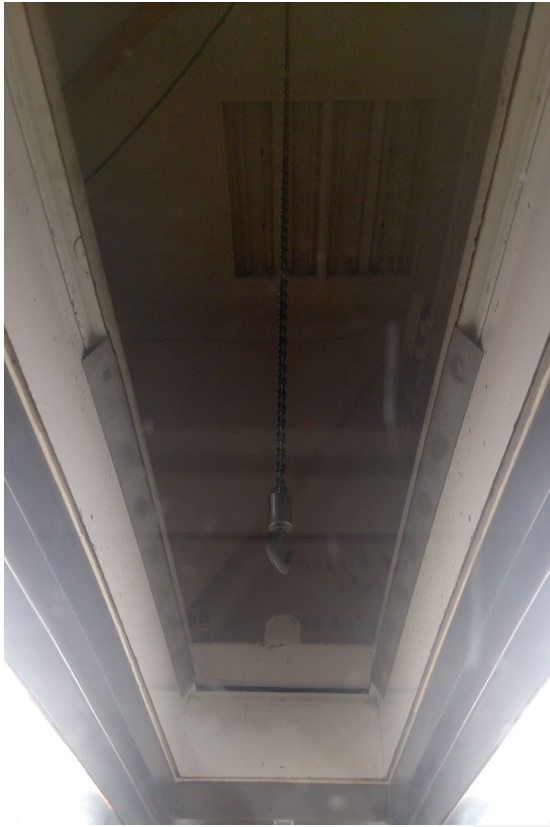
Exhibit 5. Manipulator repair glovebox refurbishment - roof opening.
