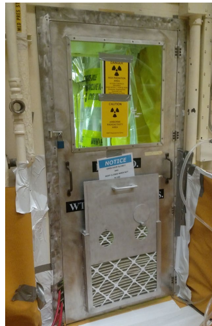
Exhibit 2. Decon Cell – temporary door configuration.
