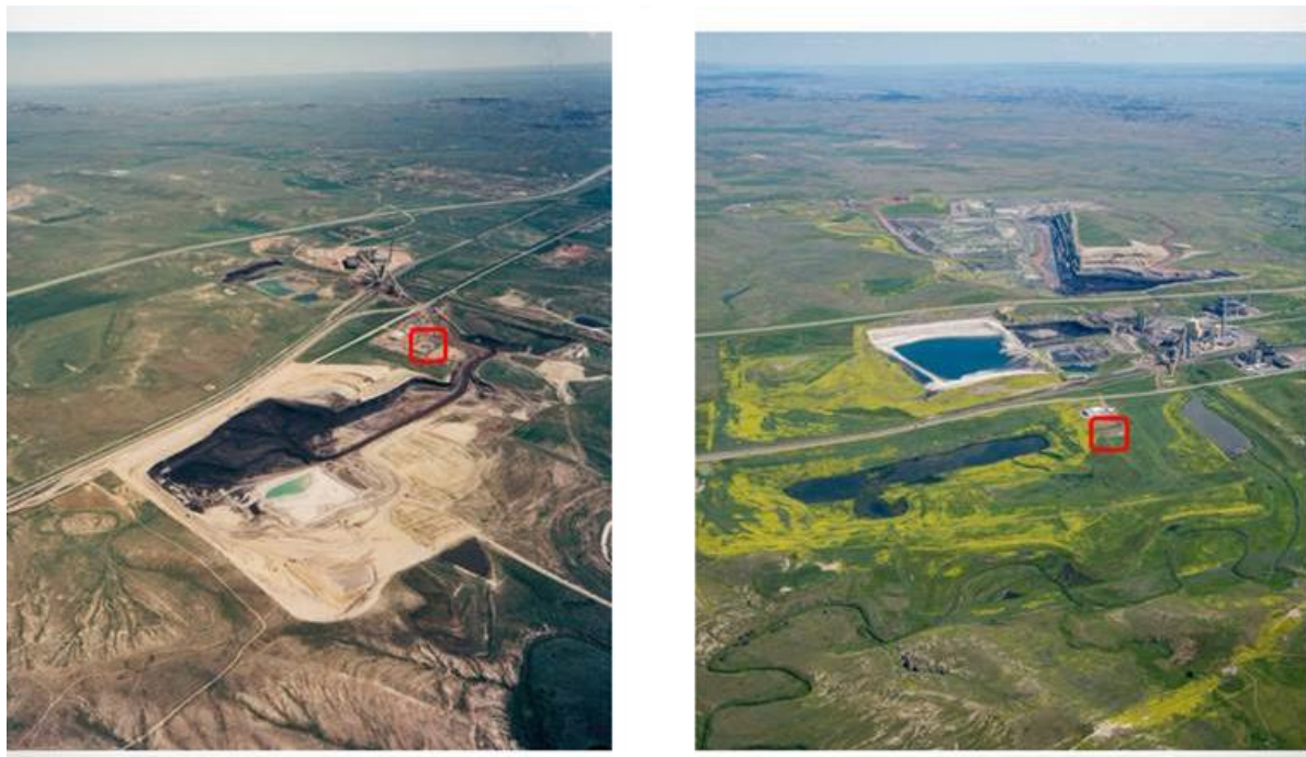
Figure 2 Mining in the South Pit Wyodak Mine and South Pit Reclamation
