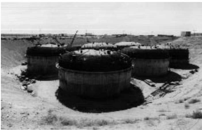
As a result of analyses conducted during the NEPA process, DOE decided not to construct six new high-level waste tanks similar to these shown under construction at Hanford during the 1970's, saving over $400 million.
