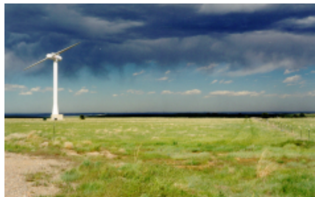
The site-wide EA evaluated the impacts of adding more test turbines like this one at the site.
