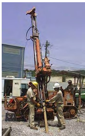
Workers obtain a soil core sample in the Field Research Center contaminated area.
