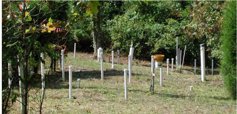
The background (uncontaminated) area of the Field Research Center contains groundwater-monitoring wellheads.
