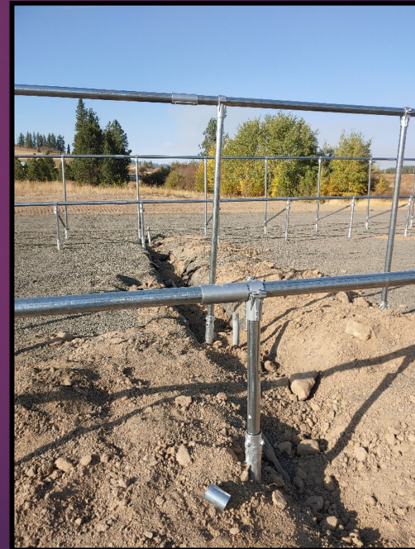
Installing the racking
