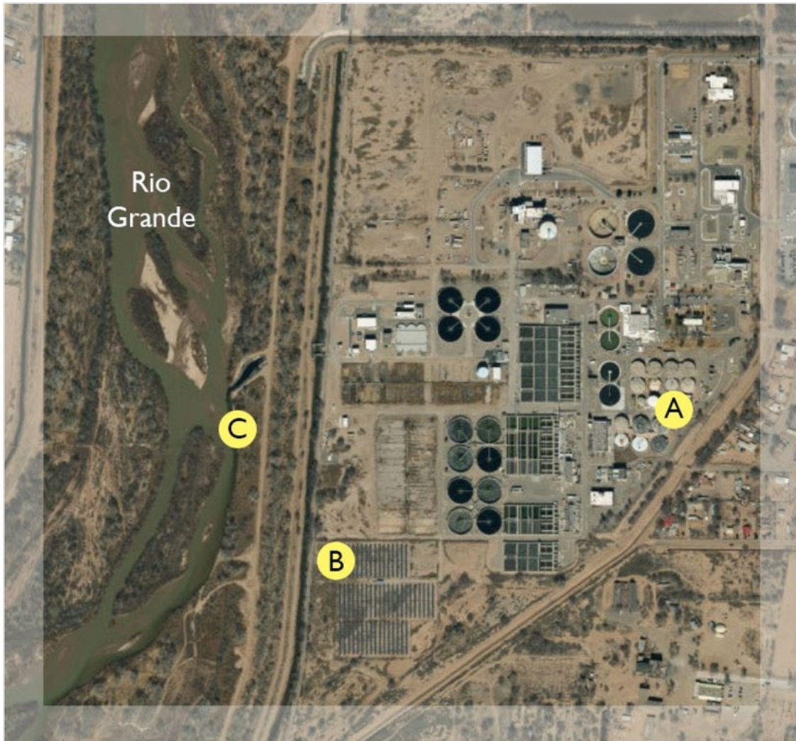
Figure 2. Albuquerque water treatment facility
