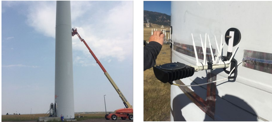
Dim UV-light source installed at Flatirons Campus. By B. Straw (left) & D. Swartz (right).
