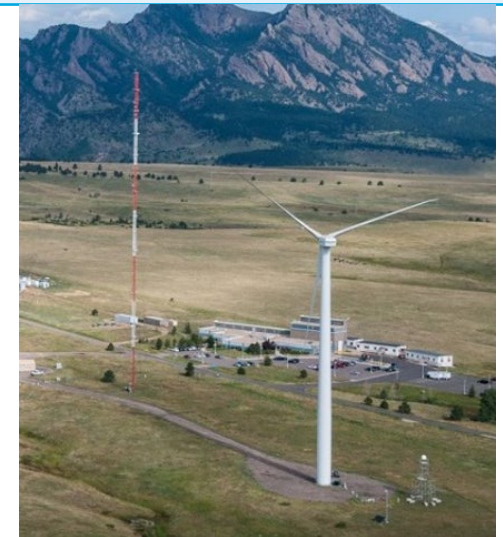
DOE 1.5 MW wind turbine used for aeroacoustics research, NREL Flatirons Campus
