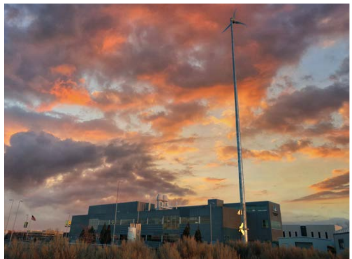
This distributed wind turbine, which supplies backup power to the Center for Advanced Energy Studies at Idaho National Laboratory (INL), is an example of a system that could use the lab's resilience metrics and framework to evaluate the benefits of distributed wind. Photo by J. Gentle, INL
