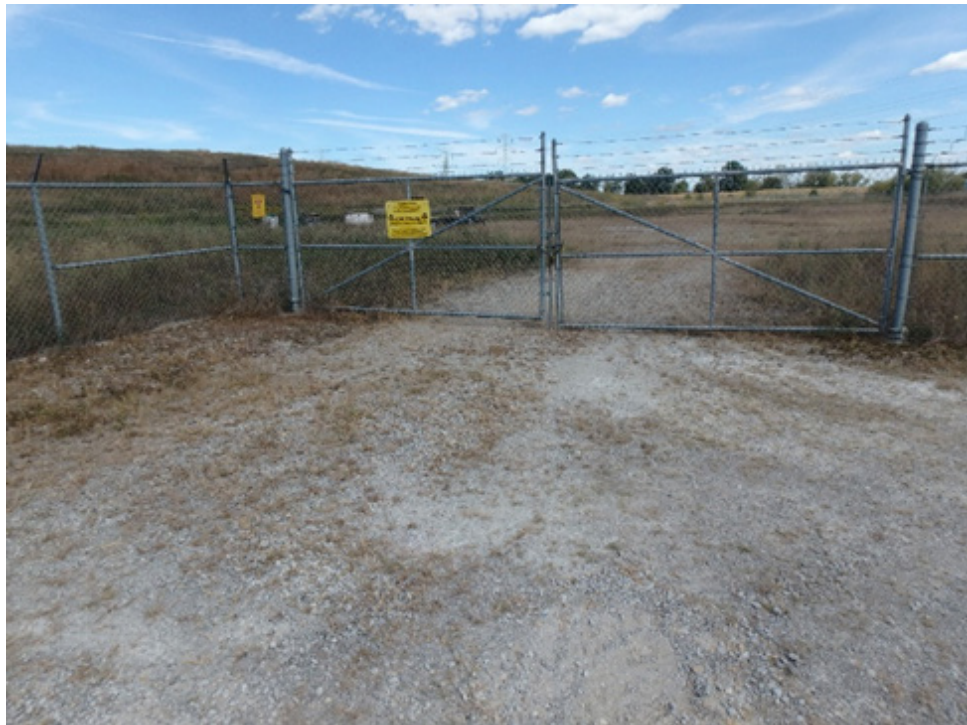
OSDF South Gate, North-Northeast Perspective
