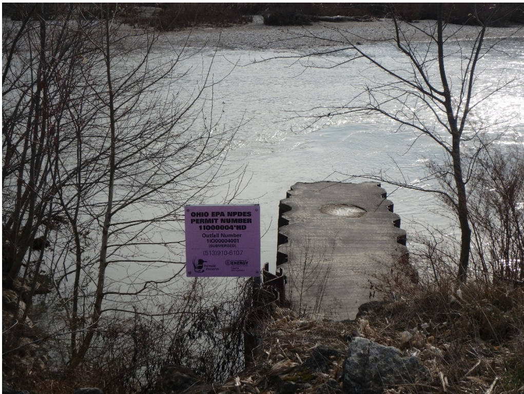
Effluent Discharge at the Great Miami River, NPDES Location PF4001
