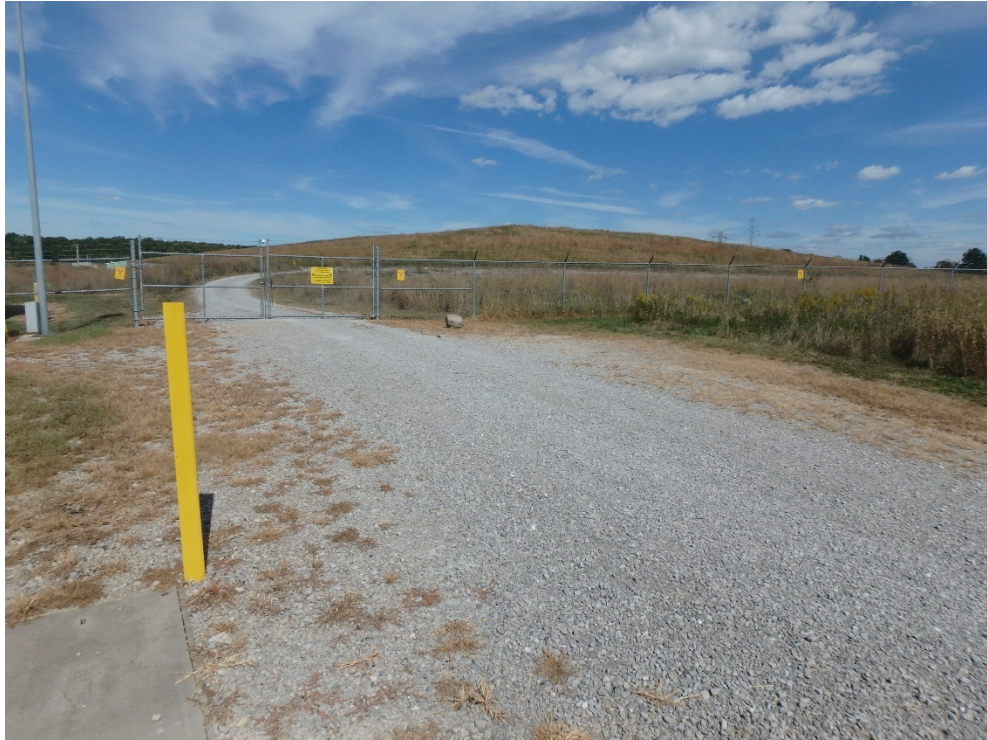
OSDF Southwest Gate, North-Northeast Perspective
