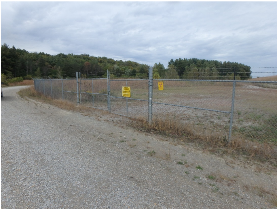
OSDF Northwest Gate, North-Northeast Perspective
