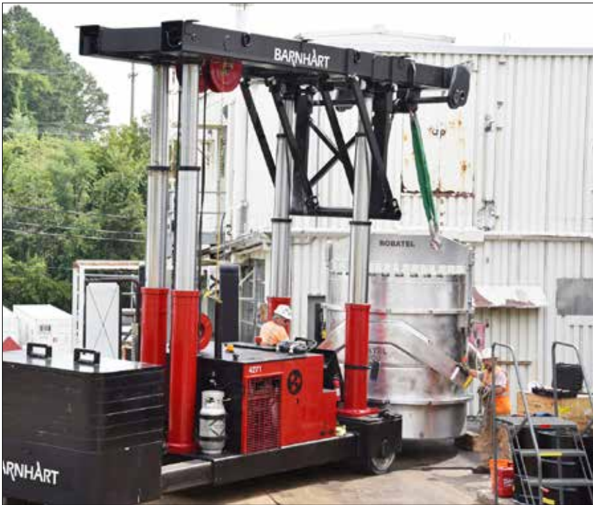
To safely remove radioactive material from the Building 3010 reactor pool, workers lowered a large waste transfer liner into the pool and safely placed irradiated materials into the secure container. (above)
