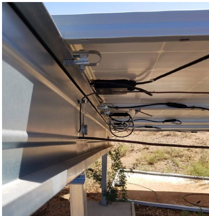
Figure 31. Use of clamping devices on structural elements
