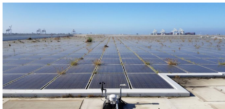
Figure 45. A similar array design provides no access for maintenance and is susceptible to wind lift
