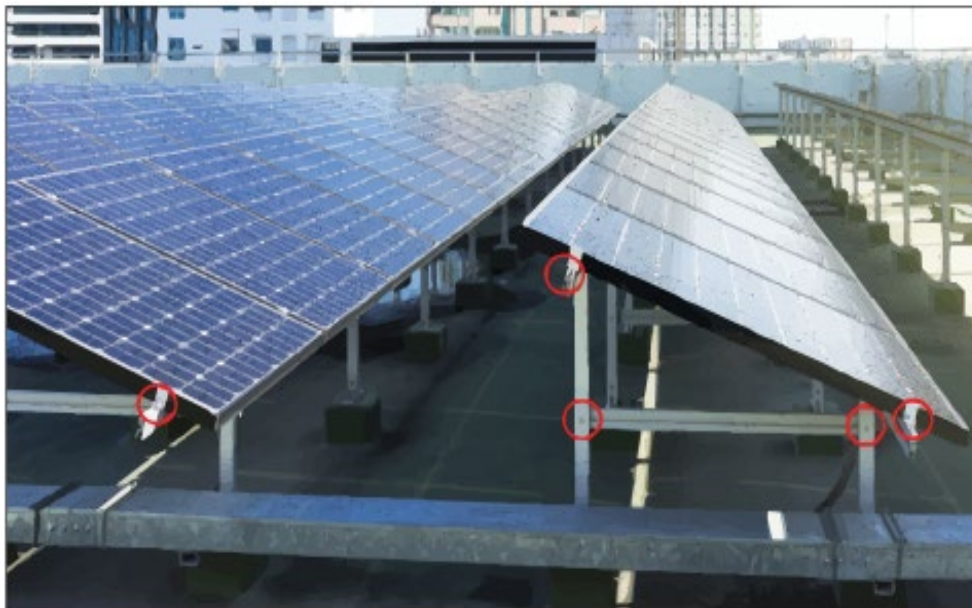
Figure 14. Bolted joints highlighted in red circles
