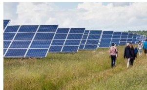
Figure 142. Pollinator plantings around a PV system
