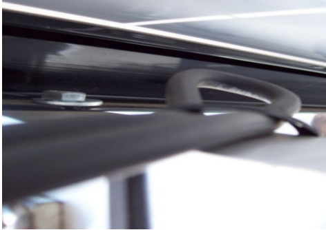
Figure 68. PV wire bent at tight radius
