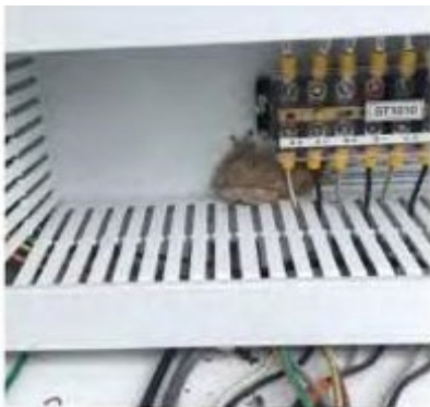
Figure 77. A frog nesting in an electrical enclosure post-flood
