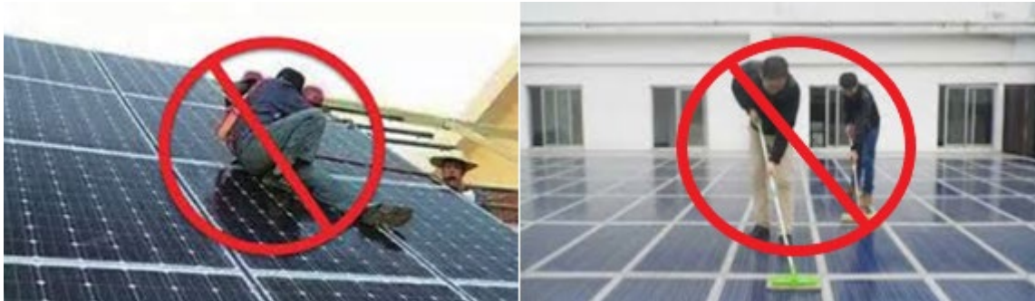
Figure 12. Never walk or lean on a module, as damage can occur
