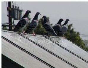
Figure 116. Animal nests must be removed from the array
