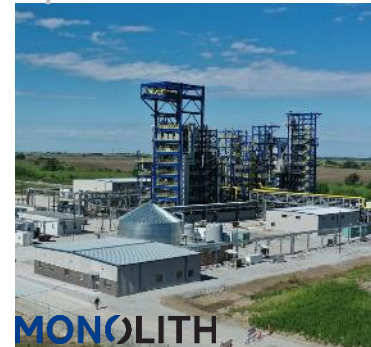
Olive Creek I (OC1), Nebraska Commissioned: 2020
