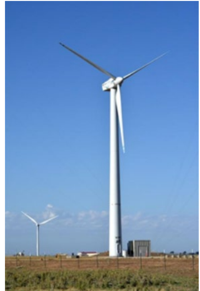
SWiFT Turbine with NRT Rotor Installed
