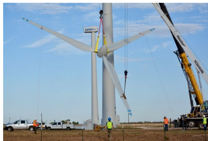
NRT Rotor Installation
