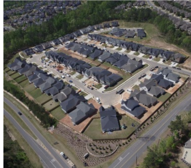
Reynolds Landing Neighborhood, Photo Courtesy: Alabama Power
