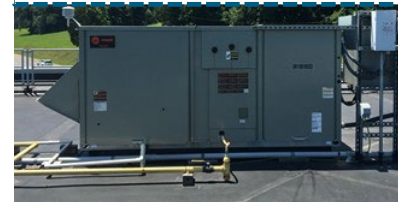
Multi-zone HVAC - RTU with VAV Reheating
