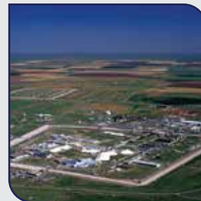
Y-12 National Security Complex
