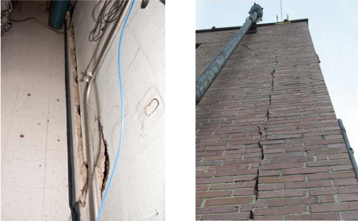
Figure 1-4. Bulging Wall in Room 270 of Building 9202 (left) and Cracked Brick Façade on the West Wall of Building 9202 (right)
