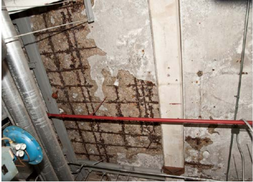
Figure 1-6. Spalling Ceiling of Fan Room 1
