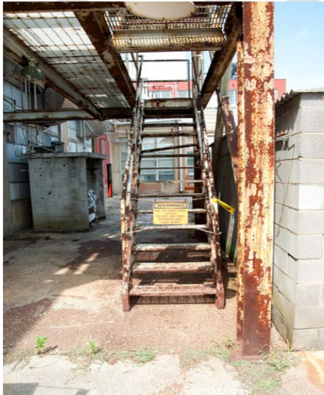
Figure 1-7. Unsafe and Unusable Emergency Stairs
