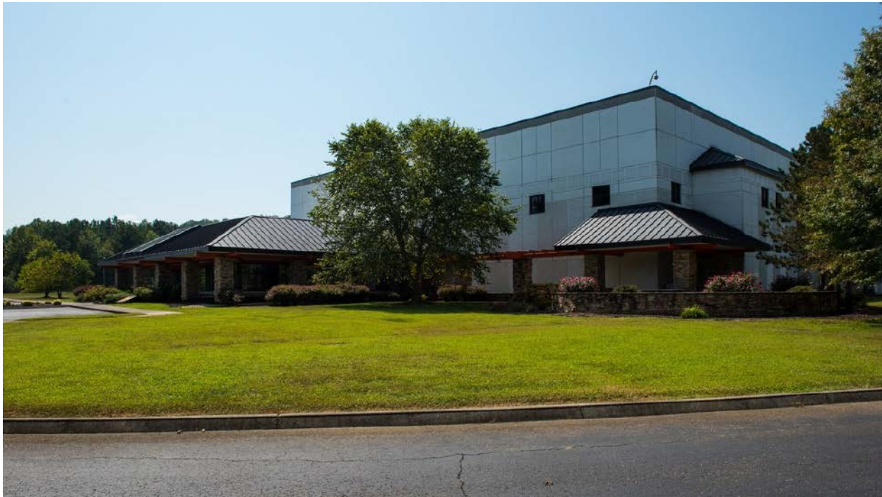
Figure 1-3. Facility Proposed for Acquisition at 103 Palladium Way, Oak Ridge, Tennessee
