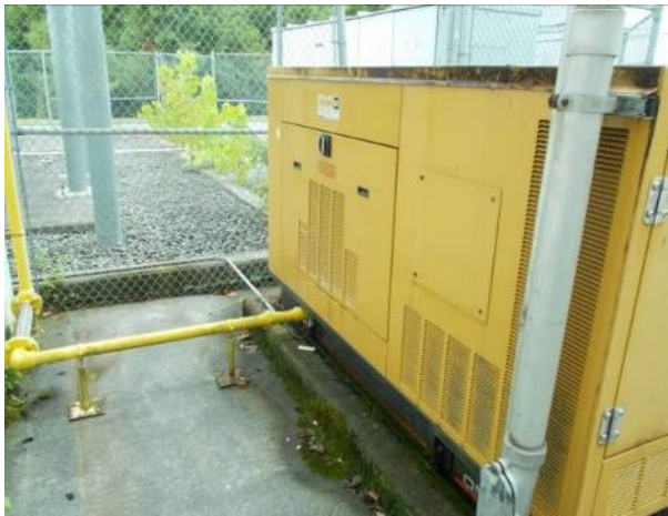
Figure 3-27. Emergency Generator
