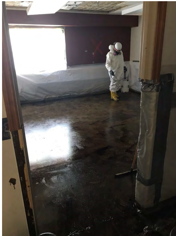
Photo 32. Administration Building, Third Floor: Floor Tile/Mastic Removal in Full Containment
