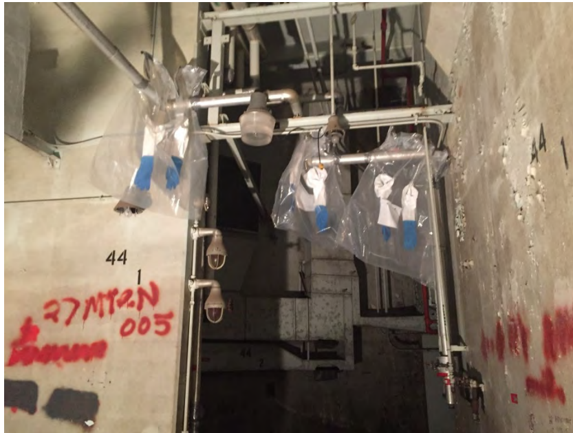
Photo 19. Reactor Building, Level 56, Before Abatement
