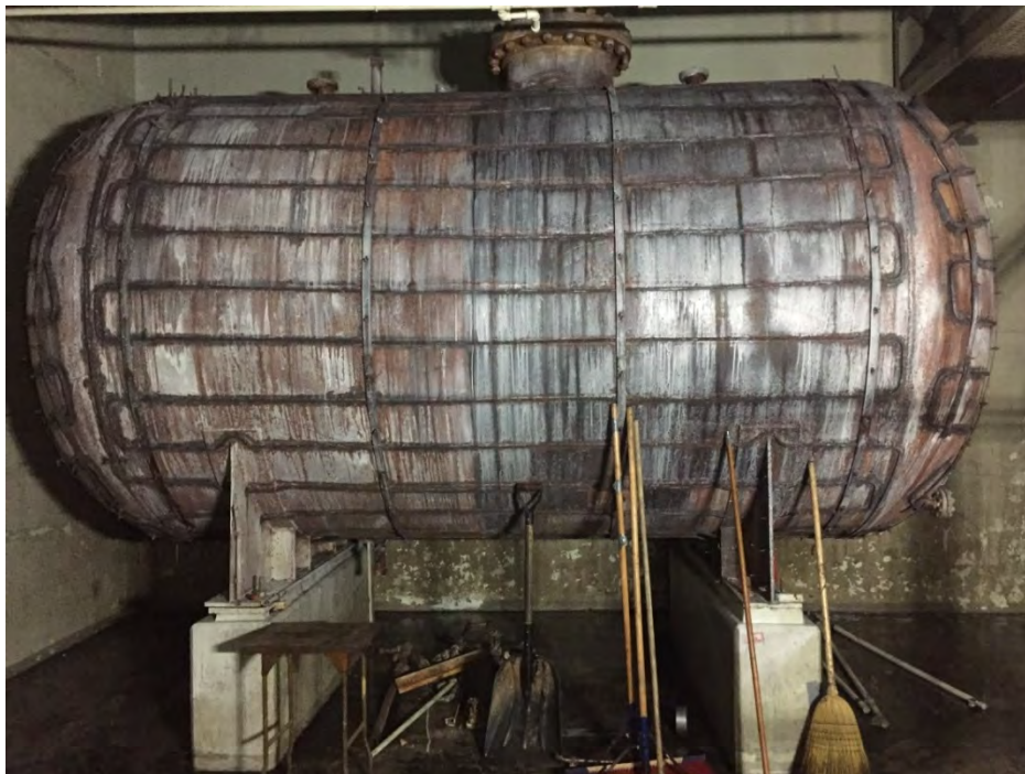
Photo 16. Administration Building, Basement, Large Chemical Tank, After Abatement
