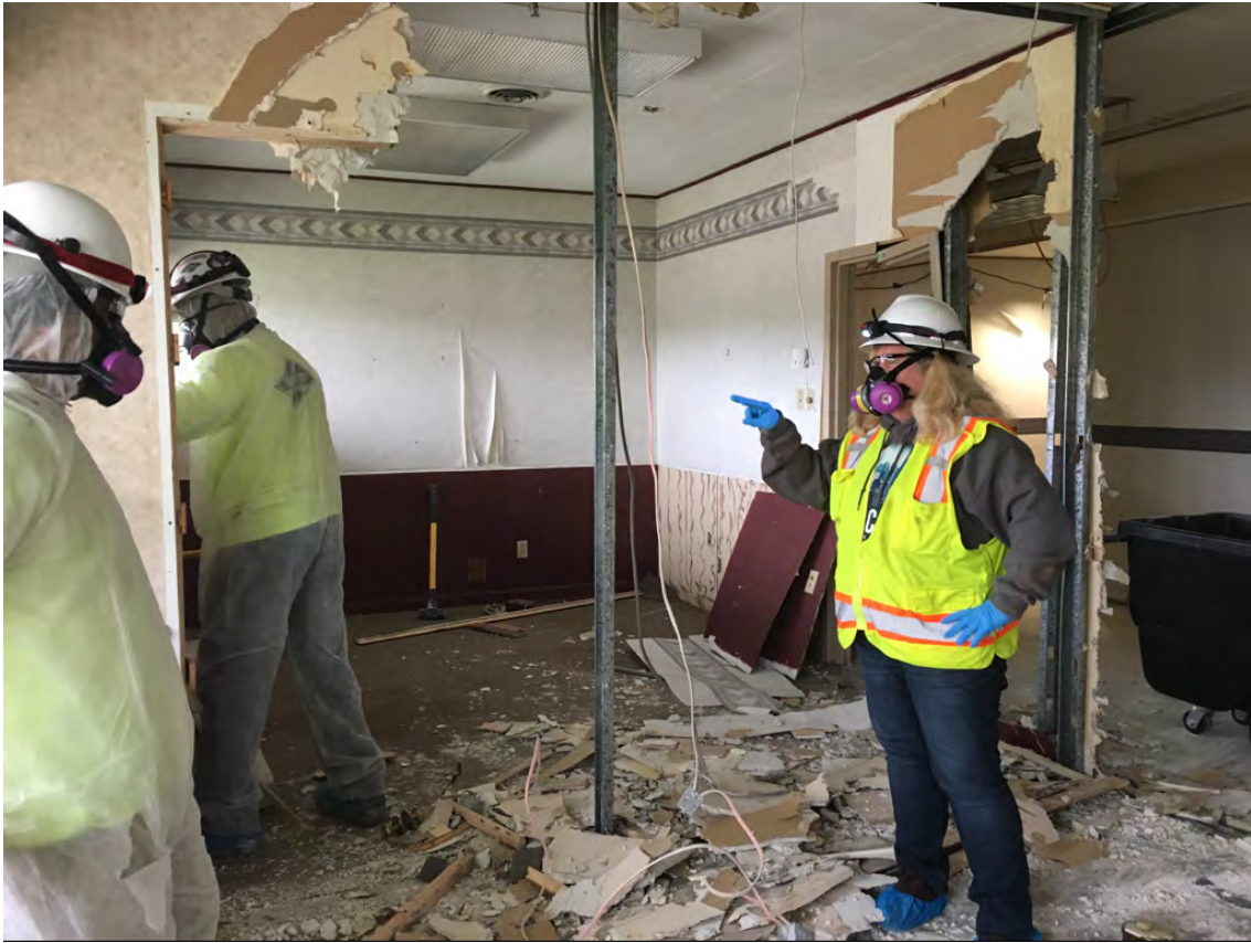
Photo 4. Administration Building, First Floor Office Area, Demolition
