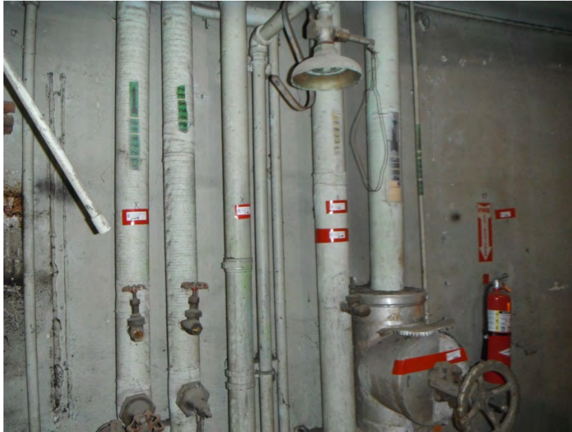
Photo 17. Reactor Building, Level 100, Before Abatement
