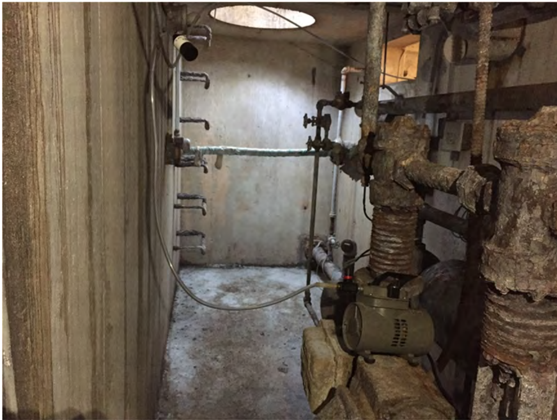
Photo 24. North Vault Final Condition, After Abatement
