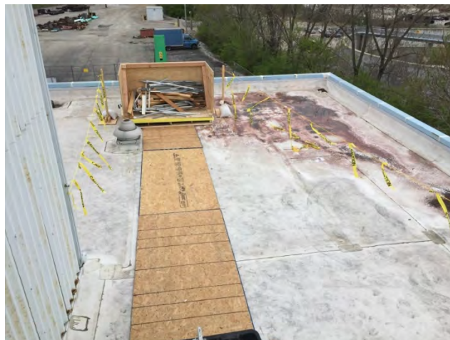
Photo 7. Waste Loadout Area on the Administration Building Roof
