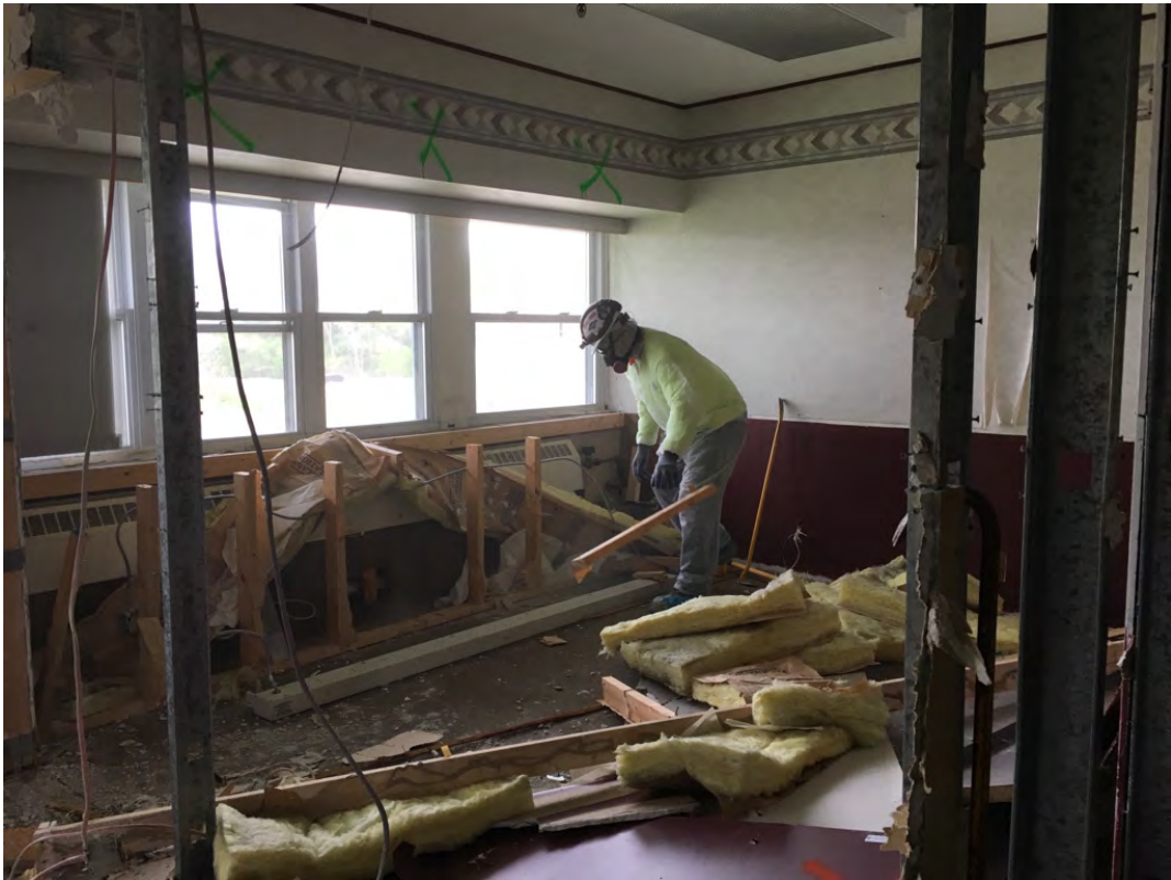
Photo 3. Administration Building, First Floor Office Area, Selective Demolition
