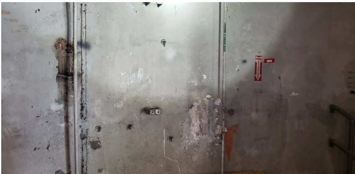
Photo 18. Reactor Building, Level 100, After Abatement
