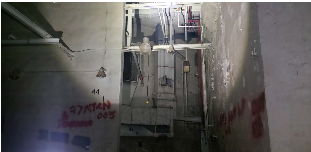
Photo 20. Reactor Building, Level 56, After Abatement
