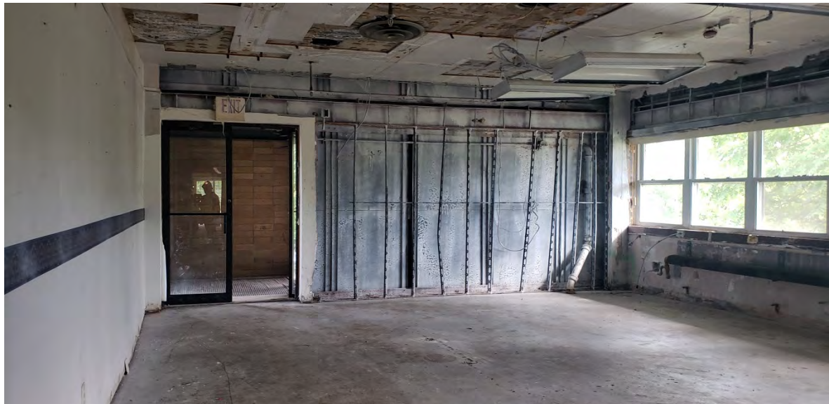
Photo 10. Piqua Administration Building, First Floor Office Area, After Abatement
