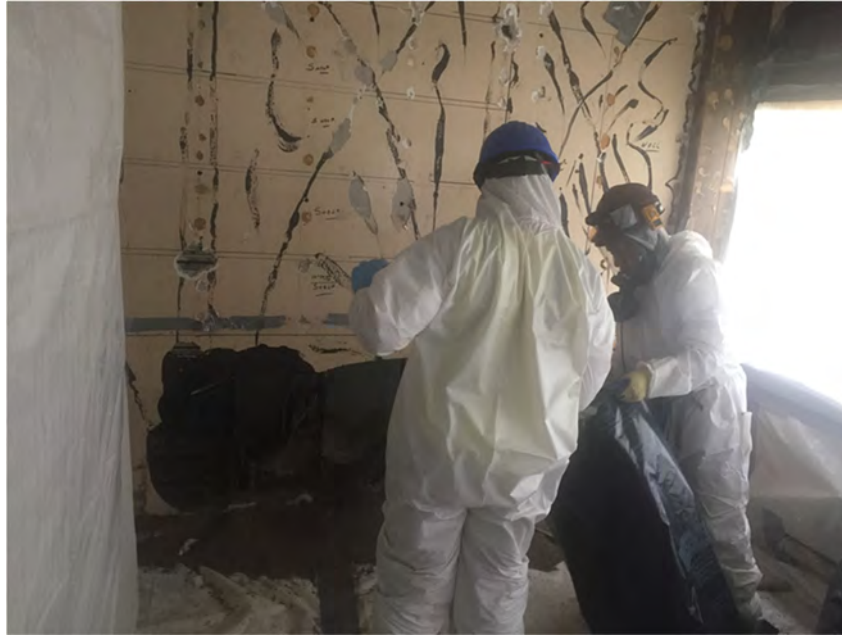
Photo 8. Asbestos Workers Removing Vermiculite for Disposal
