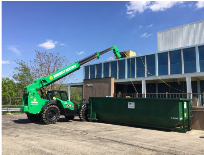
Photo 6. Using a Telehandler to Move the Waste Box
