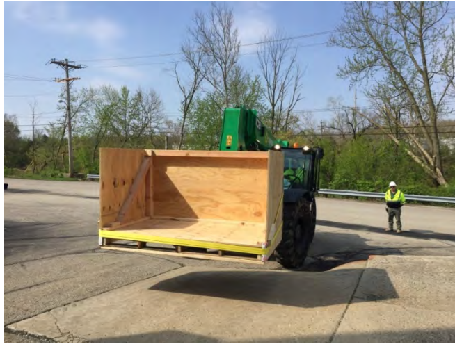
Photo 5. Waste Box for Debris from the Administration Building
