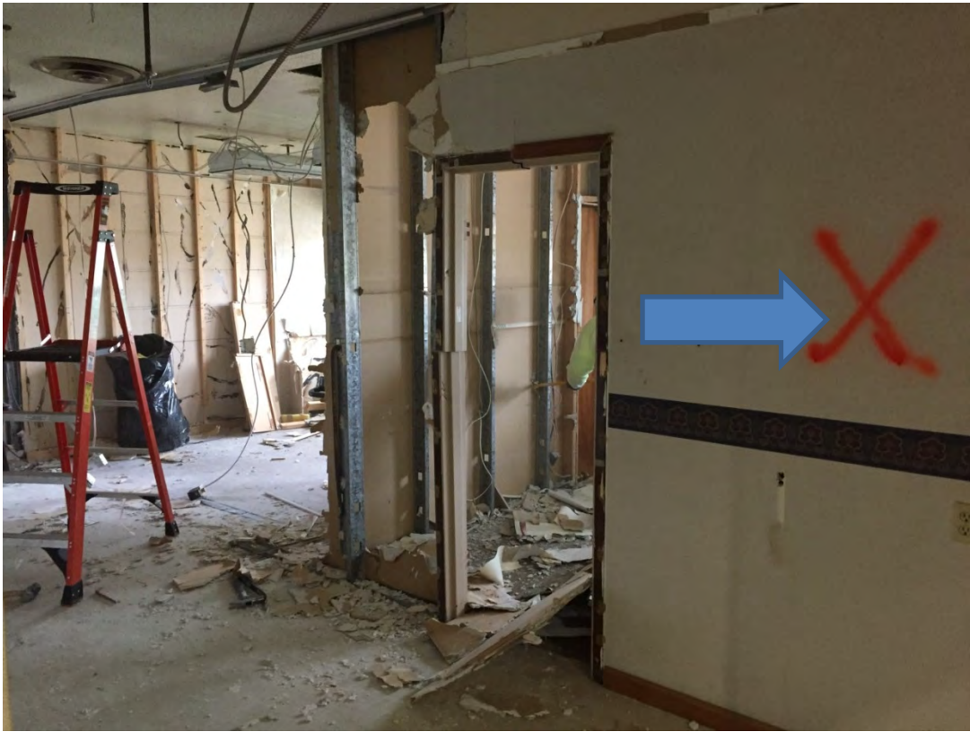
Photo 2. Administration Building, First Floor Office Area, Wall Marked for Selective Demolition
