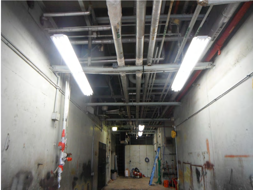
Photo 13. Piqua Administration Building, Basement Level Hallway, Before Abatement
