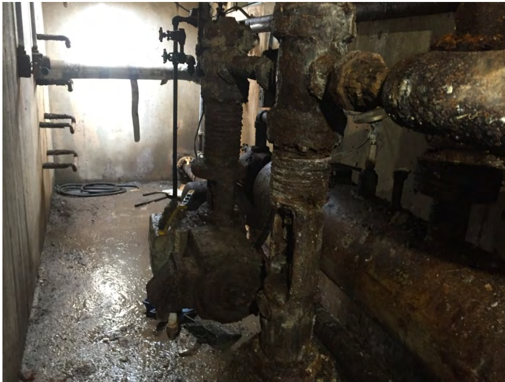
Photo 23. North Vault After Pumping and Before Abatement
