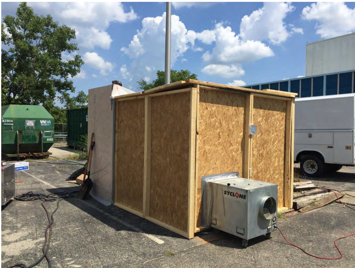
Photo 21. Entry to the Below-Grade Utility Vaults
