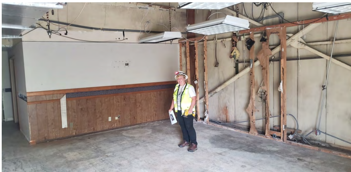
Photo 12. Piqua Administration Building, Conference Room, After Abatement
