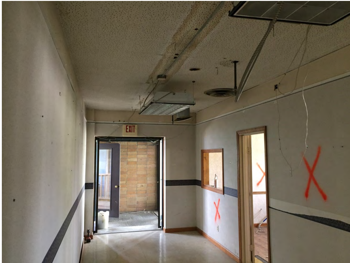
Photo 9. Piqua Administration Building, First Floor Office Area, Before Abatement
