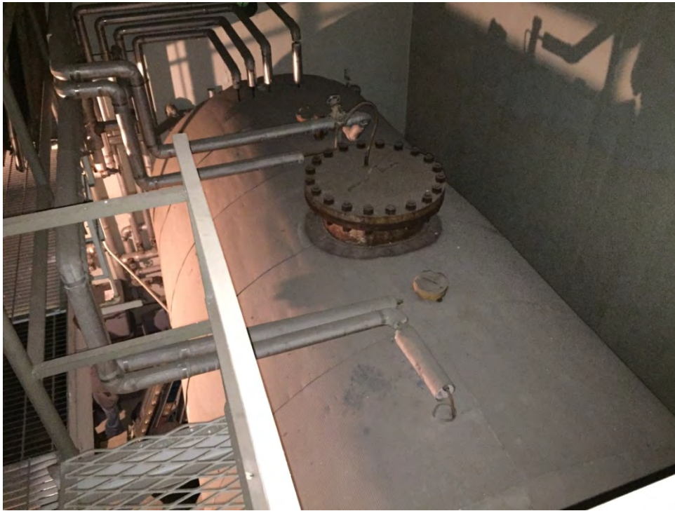
Photo 15. Administration Building, Basement, Large Chemical Tank Before Abatement
