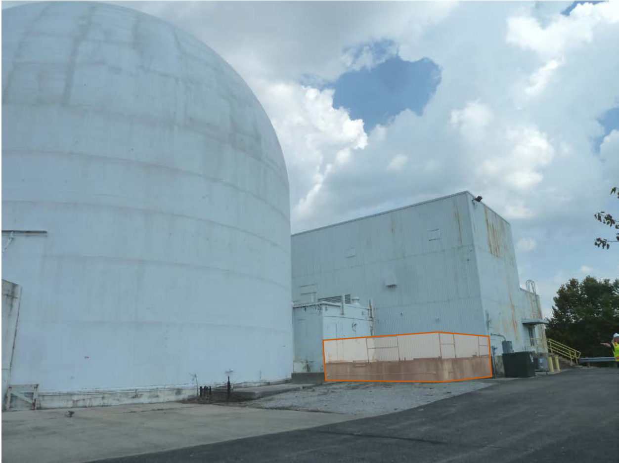
Photo 7. Steel containment dome above the belowground entombment in left of frame. Administration building shown in right of frame. Building between the containment dome and the administration building is an outdoor locker previously used for chemical storage. The concrete pad adjacent to the outdoor locker (indicated with orange outline and tint) may contain PCBs due to previous storage of equipment and fuels.
