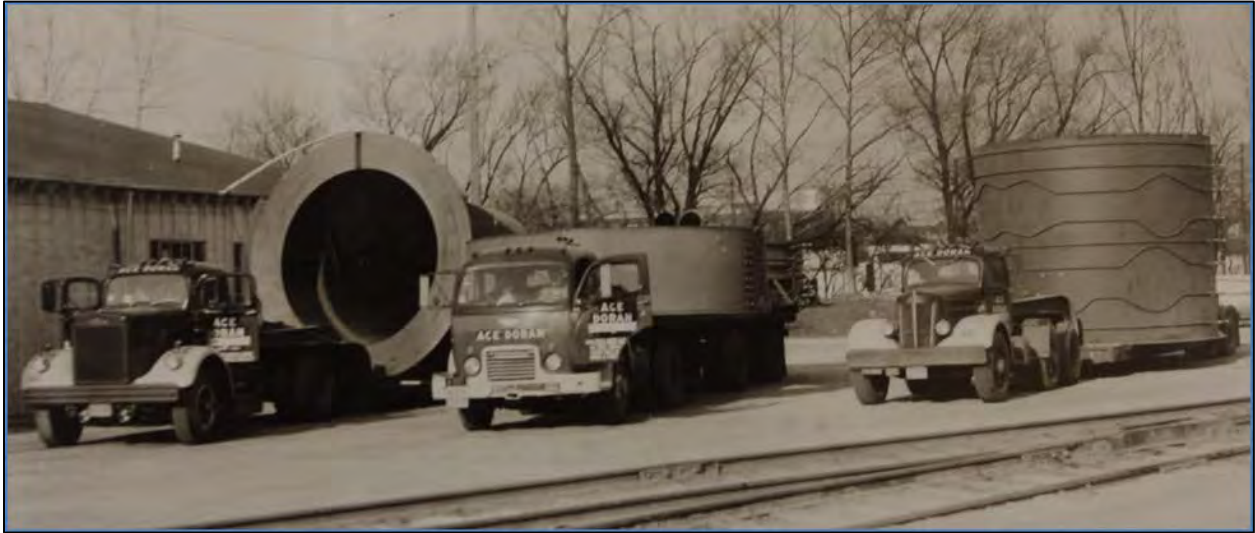
Figure 7. Delivery of the Reactor Vessel.
