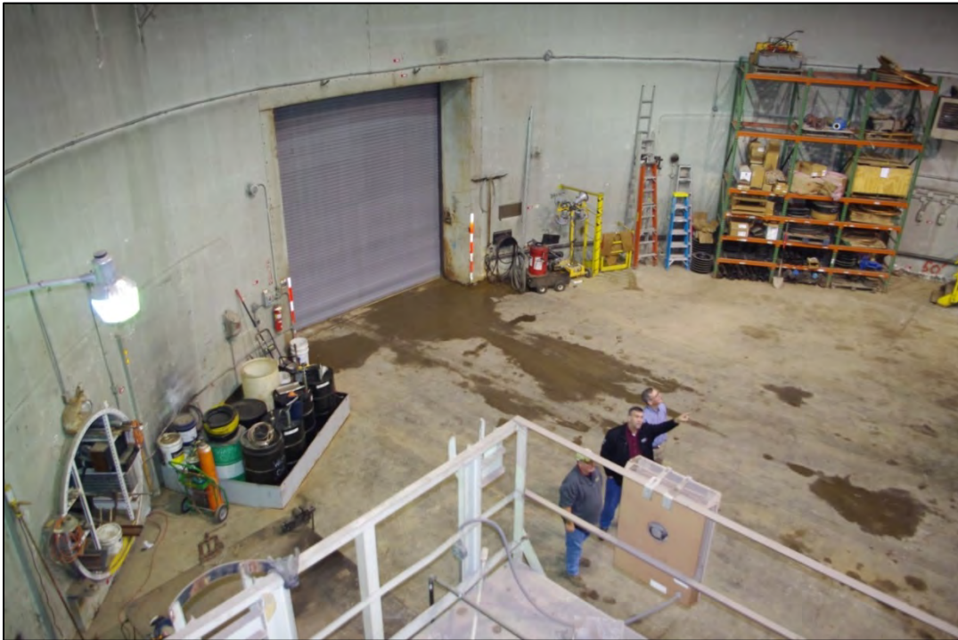
Figure 25. Piqua Reactor Building, Detail View Inside the Concrete Reactor Containment Dome. The reactor was covered by a waterproof membrane and an additional layer of cement after it was defueled during reactor decommissioning.
