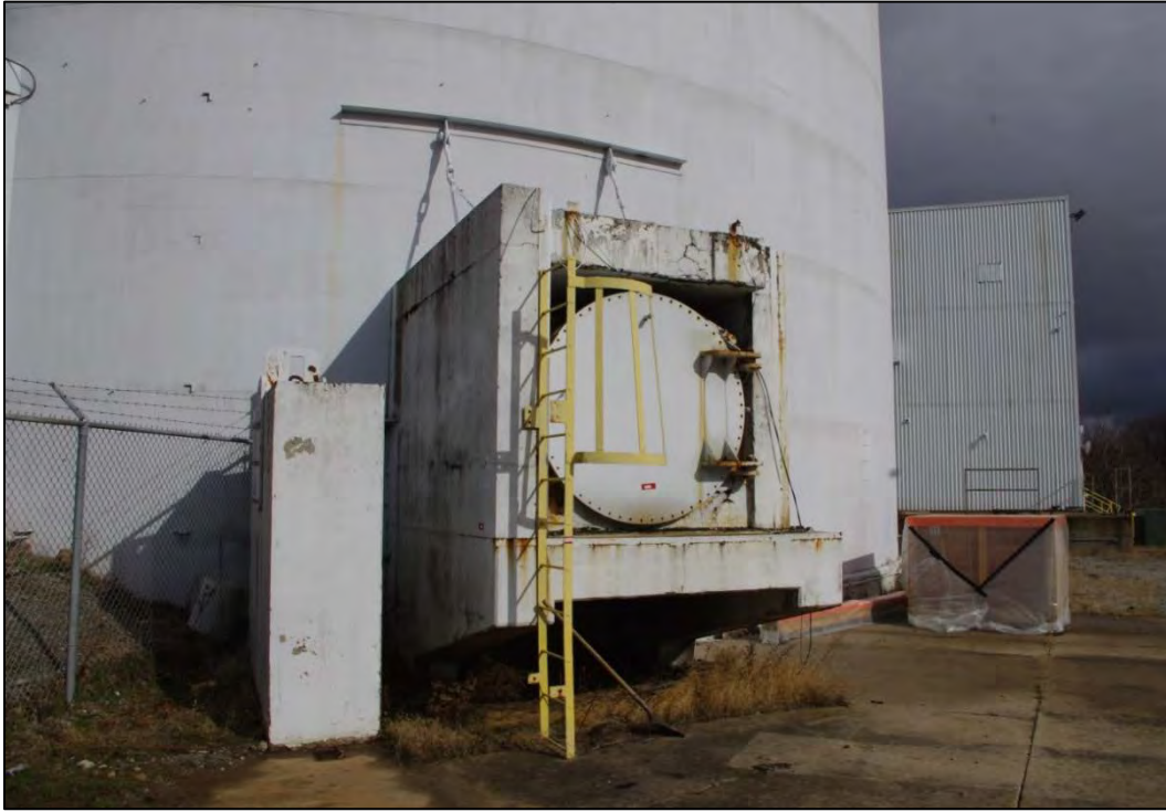
Figure 21. Piqua Reactor Building, Current View.
