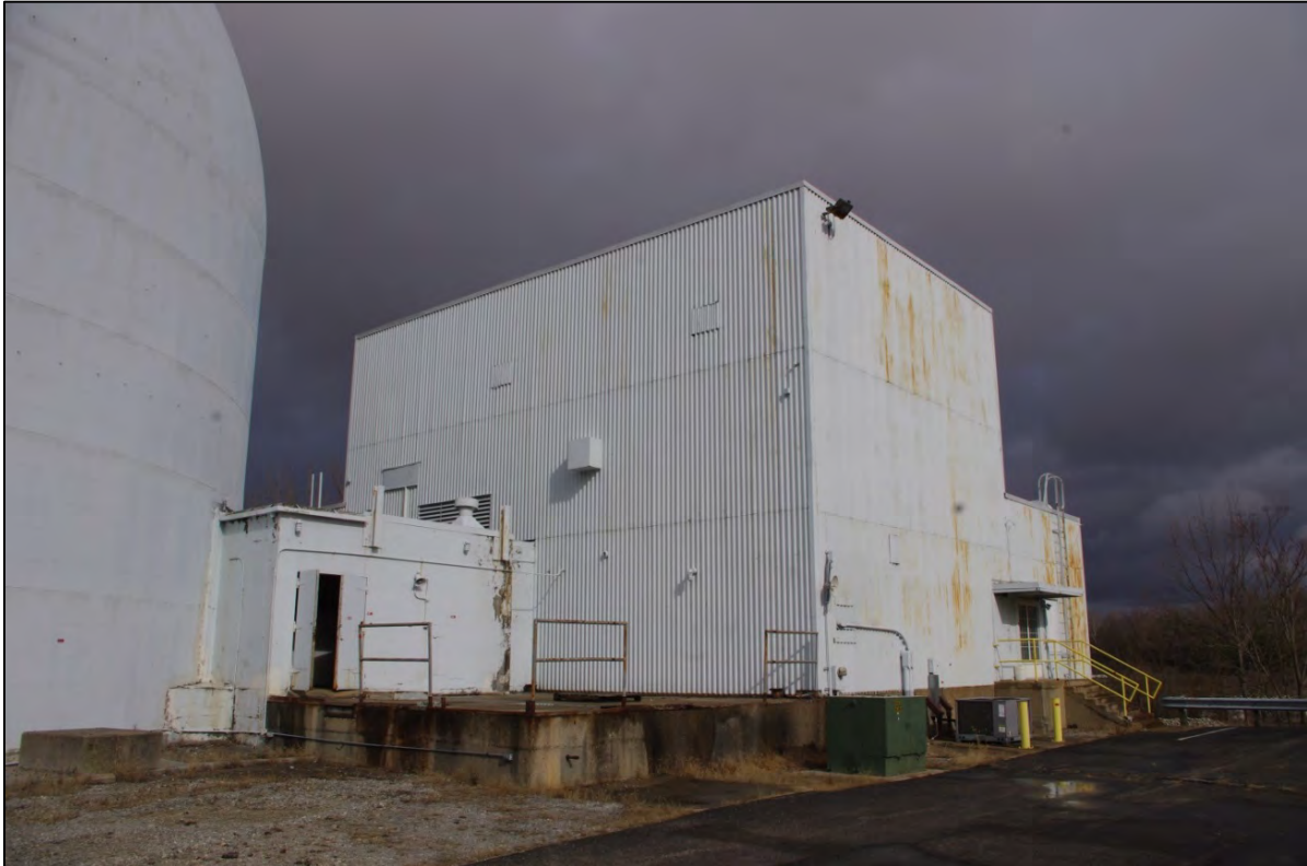
Figure 18. Piqua Reactor Building, Current View, Looking Northeast.
