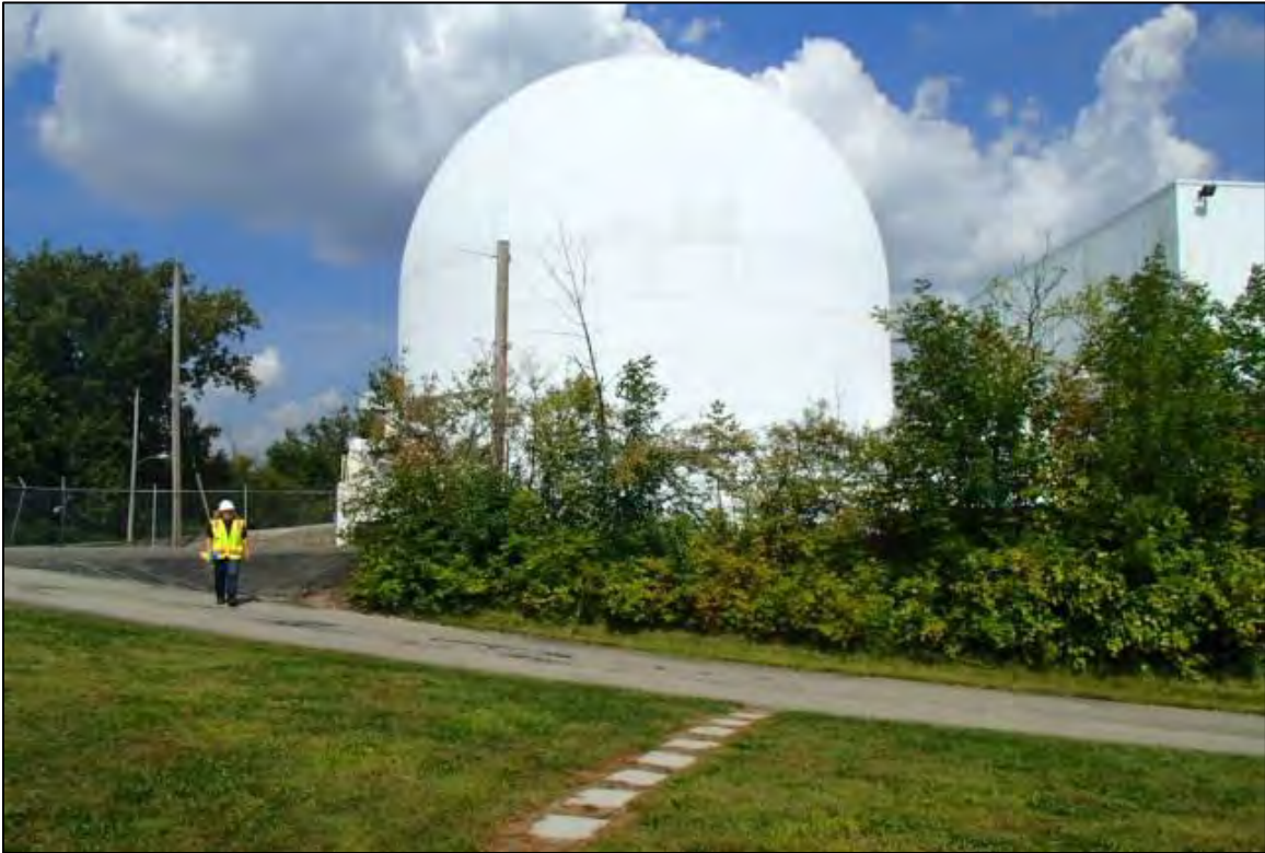
Figure 7: View showing leveled, graded area along southern edge of the APE and sloped terrain immediately to the south, facing north.
