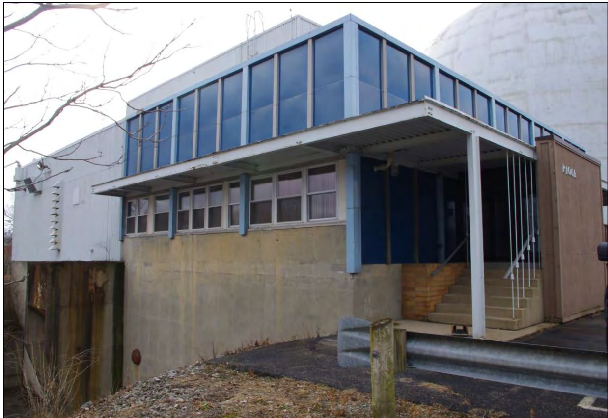
Figure 16. Piqua Reactor Building, Current View, Looking Southwest.
