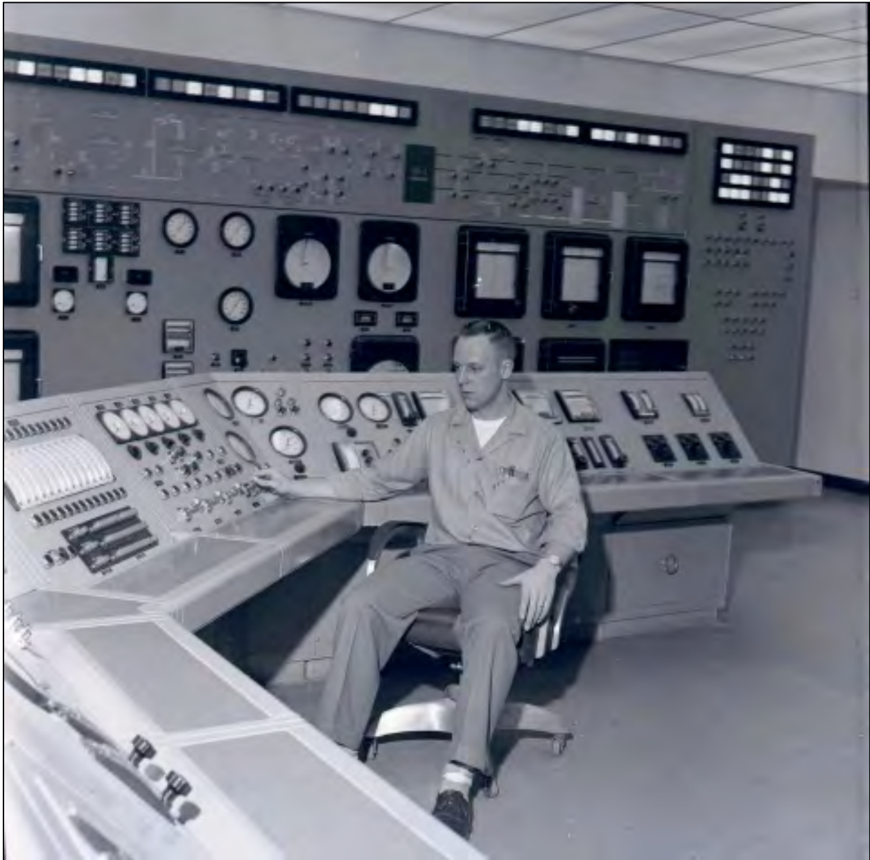
Figure 9. Piqua Reactor Building Control Room, Circa 1962.
