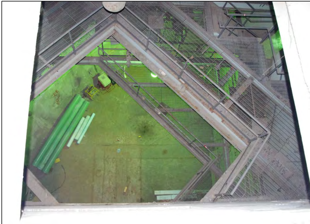
Figure 26. Piqua Reactor Building, Detail Inside the Concrete Containment Dome. The height of the interior space is well illustrated.
