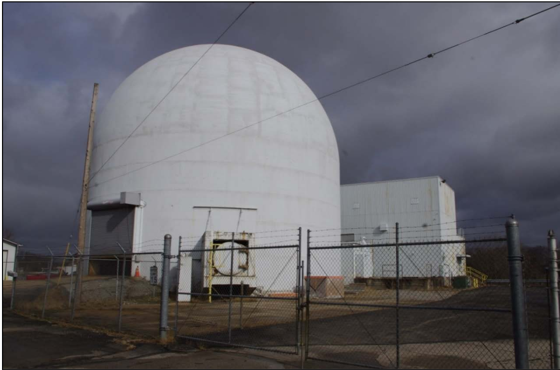
Figure 19. Piqua Reactor Building, Current View, Looking Northeast. The truck access door was cut into the reactor containment dome as part of the reactor deactivation process. The reactor containment dome now provides storage space.
