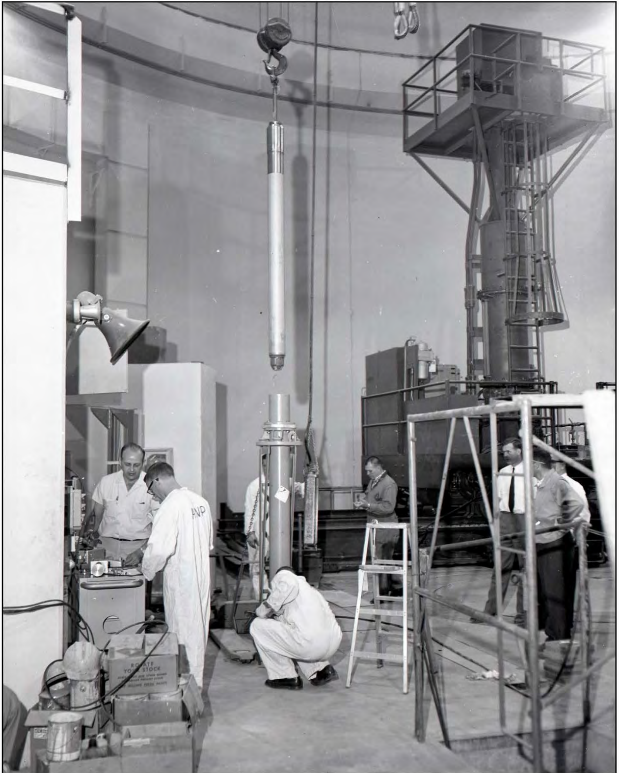
Figure 12. Piqua Reactor Building, Interior Detail Photograph. A fuel rod is being inserted, circa 1962.
