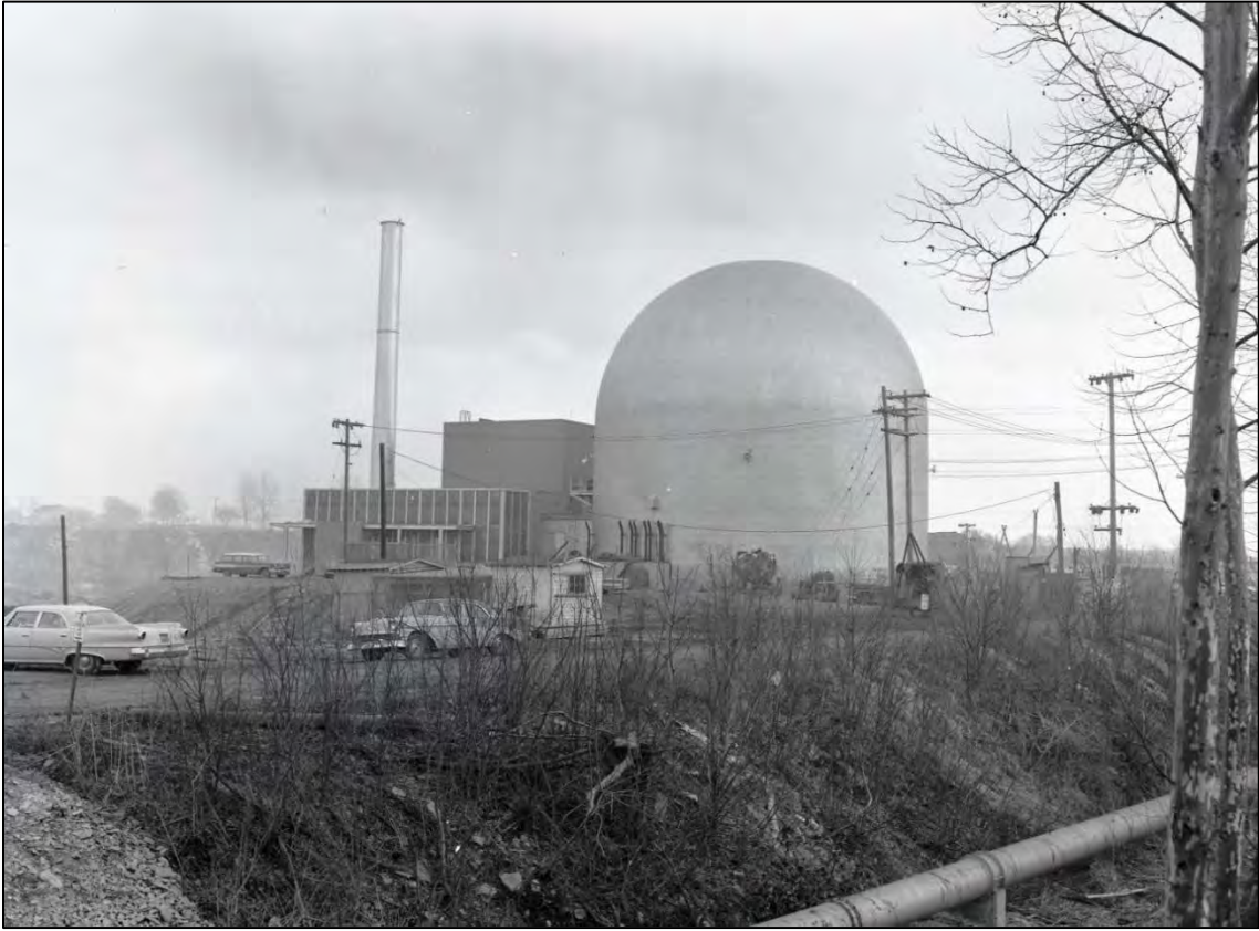
Figure 13. Piqua Reactor Building Looking Southeast, Circa 1962.
