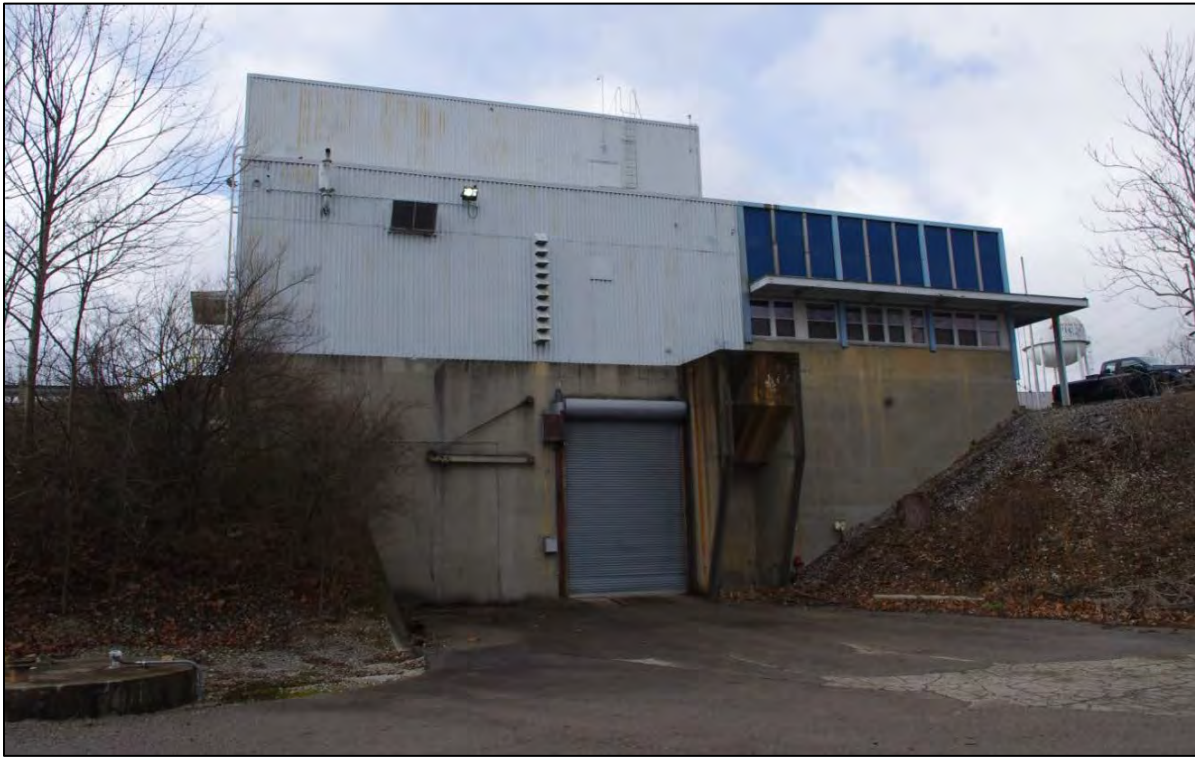
Figure 17. Piqua Reactor Building, Current View, Looking West.
