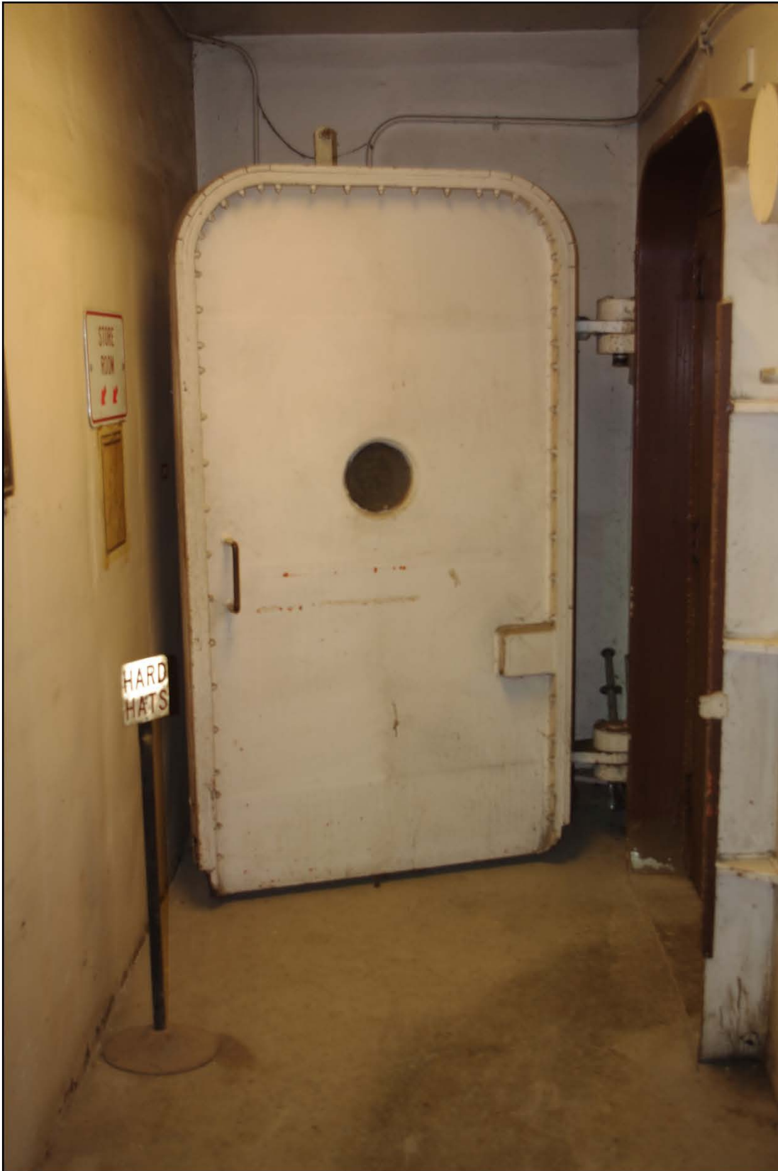
Figure 27. Piqua Reactor Building, Door Detail.
