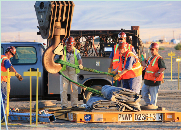
Photo: Crane and rigging crew at the Hanford Site
