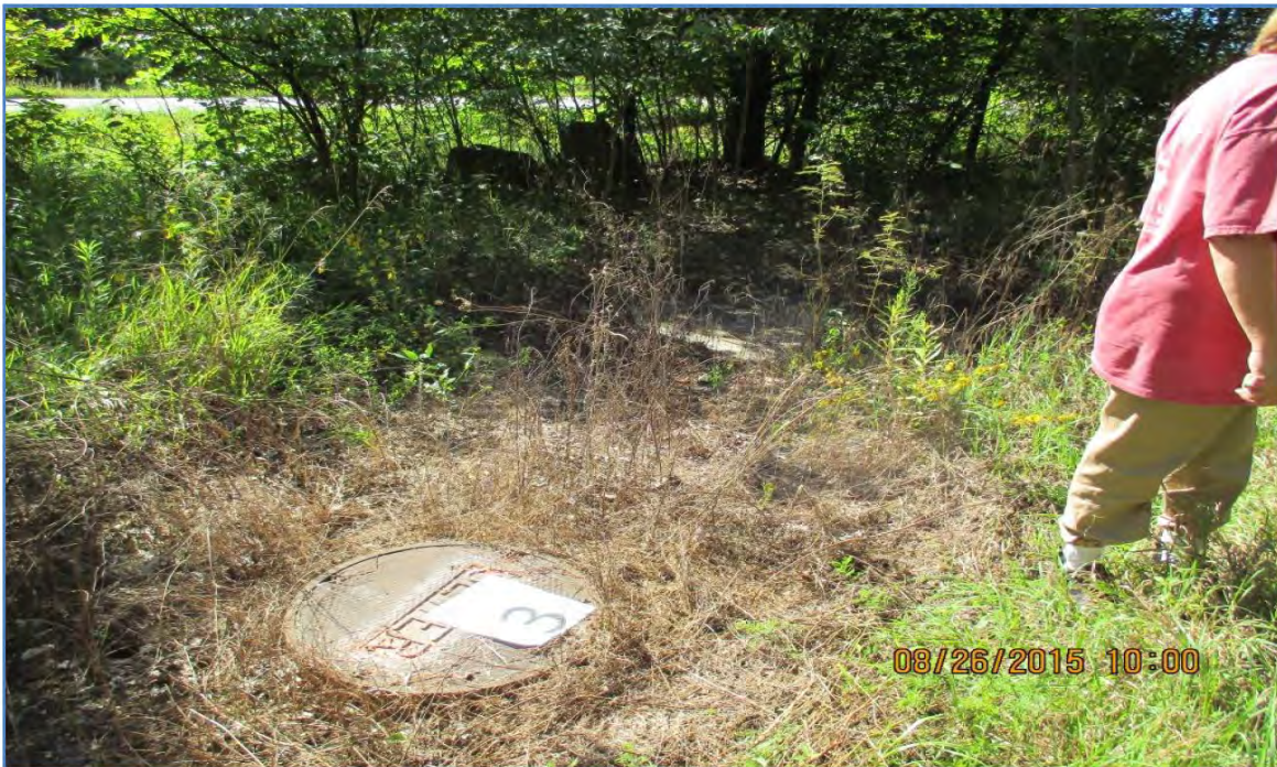
Manhole 3: Near Highway 94
