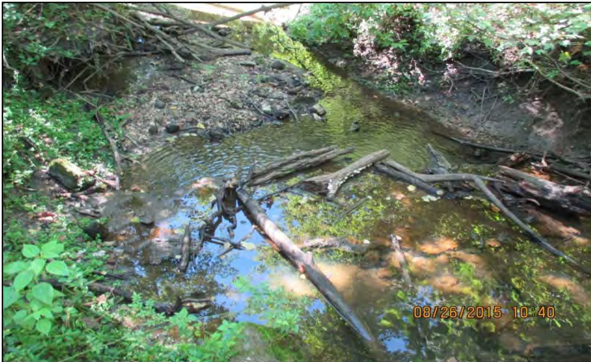
Pipeline crossing under small creek
