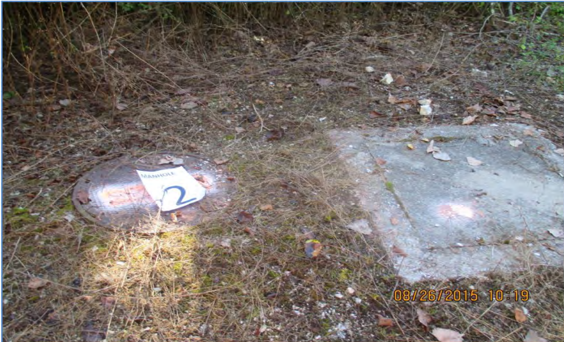
Manhole 2: Near Old Railroad Line
