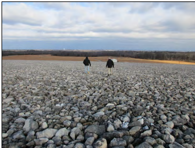
Photo 3: Disposal Cell Inspection
