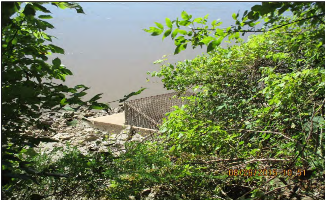
Discharge Outfall Structure at Missouri River
