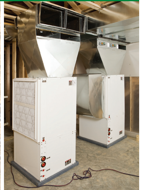
Geothermal heat pump systems, consisting of the heat exchanger (left) and the heat pump (right), heat and cool a home by transferring heat to and from the earth.
