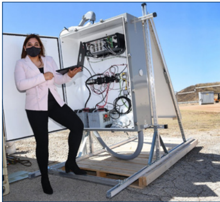
Dr. Ventura with one of the seismo-acoustic sensors deployed for the DNN R&D project at Pantex.
