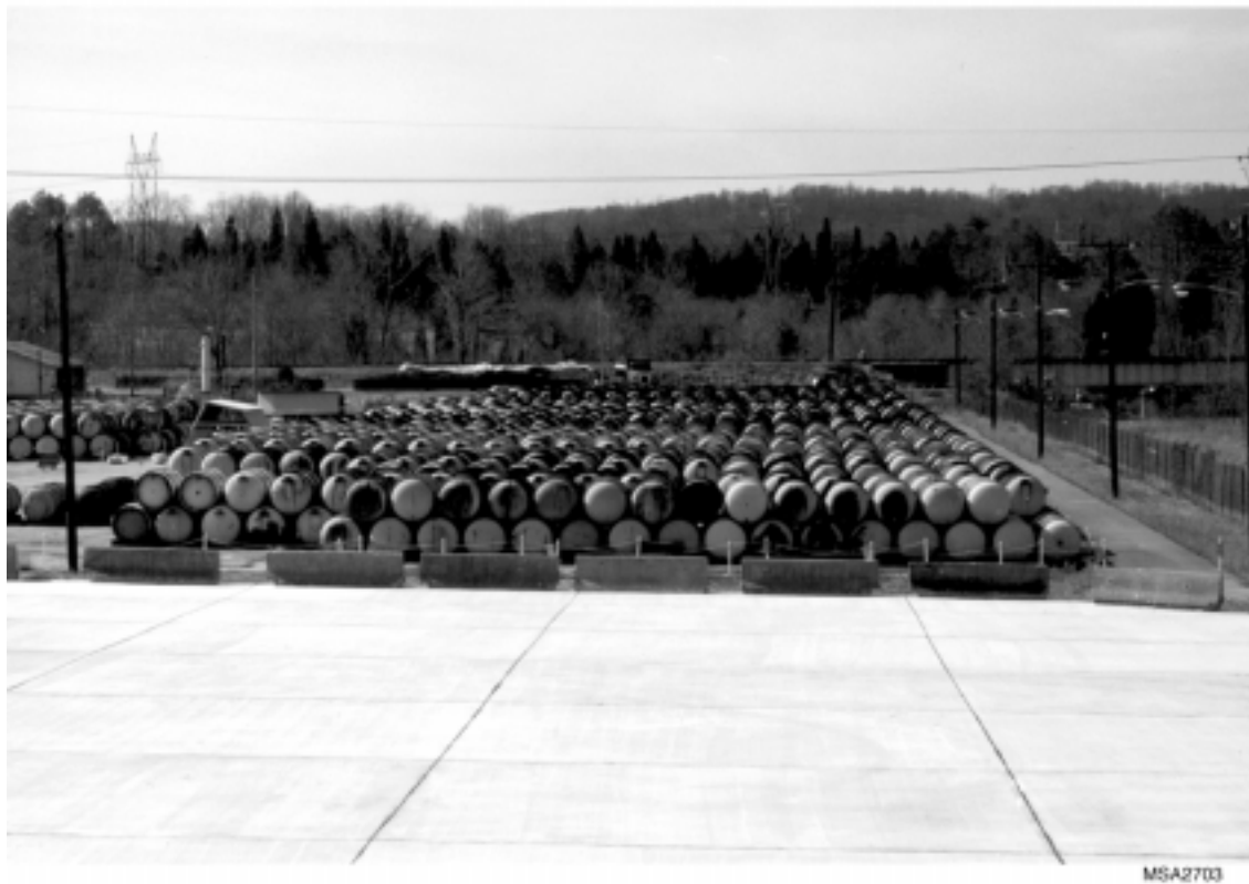
FIGURE S.2 Depleted UF 6 Cylinders in Storage Yards
