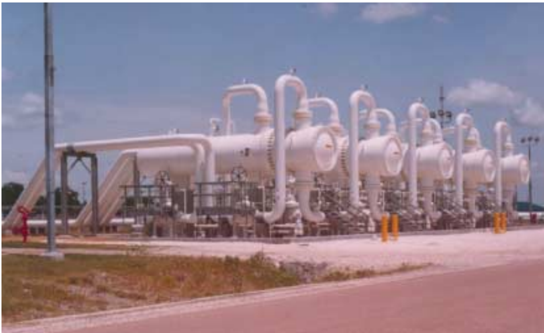
Life Extension: New Heat Exchangers at Big Hill Cool the Oil During Drawdown
