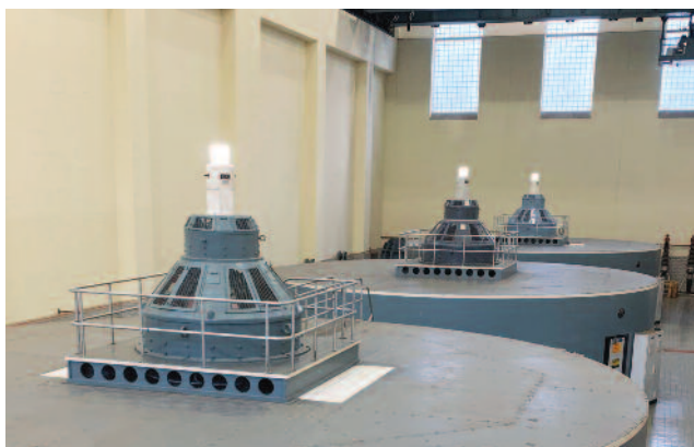
Rehabilitation was completed on the second of three generators at Center Hill powerplant. Downstream dissolved oxygen testing of the two operational aerated turbines in September 2020 yielded a 5 milligrams/liter sustained environmental improvement.
