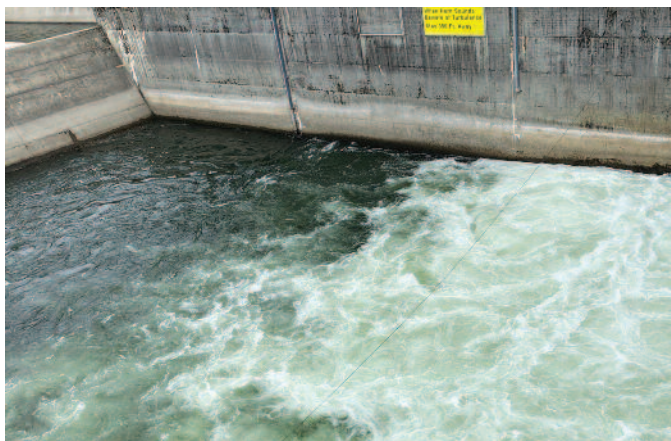
Rehabilitation was completed on the second of three generators at Center Hill powerplant. Downstream dissolved oxygen testing of the two operational aerated turbines in September 2020 yielded a 5 milligrams/liter sustained environmental improvement.
