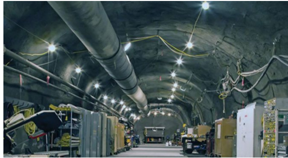
Tunnel at the U1a Complex
