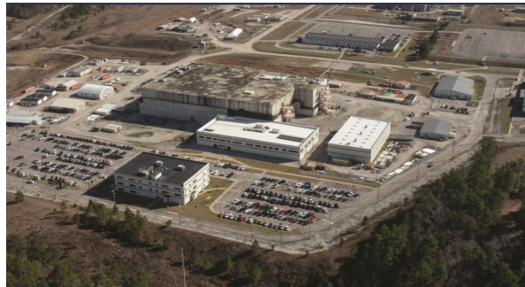
Site of future Plutonium Pit Production Facility at SRS “Final Environmental Impact Statement for Plutonium Pit Production at the Savannah River Site in South Carolina”, NNSA, 2020
