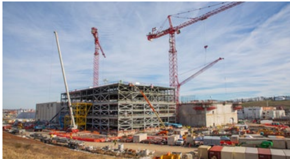
The Uranium Processing Facility at Y-12 progresses toward its 2025 completion date
