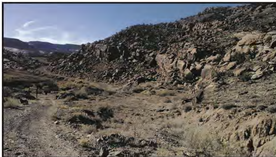
Figure 11: View west across the Burro Tunnel's pre-1970 waste rock bench. The tunnel portal is in the sandstone ledge at upper right. Note the deep erosion channel emerging from lower right and crossing the bench's surface to photo-center, where it drops over the bench shoulder. Not only has heavy erosion incised gullies, but also washed away much of the original top-surface. Given the damage and lack of originality, the top-surface is a non-contributing portion of the bench. For the sediment control project, the gully is to be lined with riprap boulders submerged in fine waste rock for stability. Most of the riprap will appear similar to the existing channel walls, while storm runoff might expose boulder faces in the gully floor.
