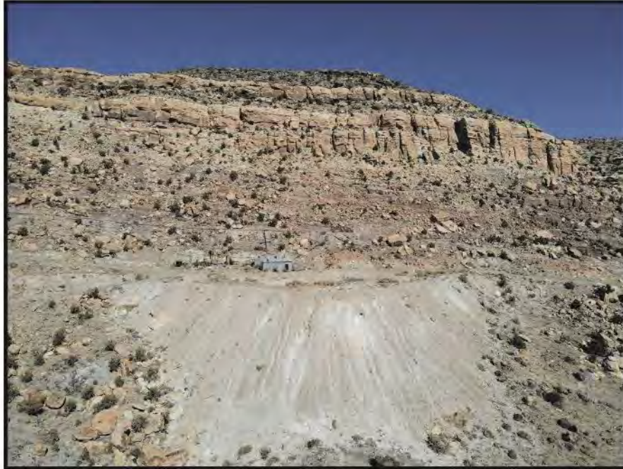
Figure 7: North overview of Burro No.5, including its surface plant on an original pad of waste rock. The pad is a major landscape feature, and the entire complex is contributing.
