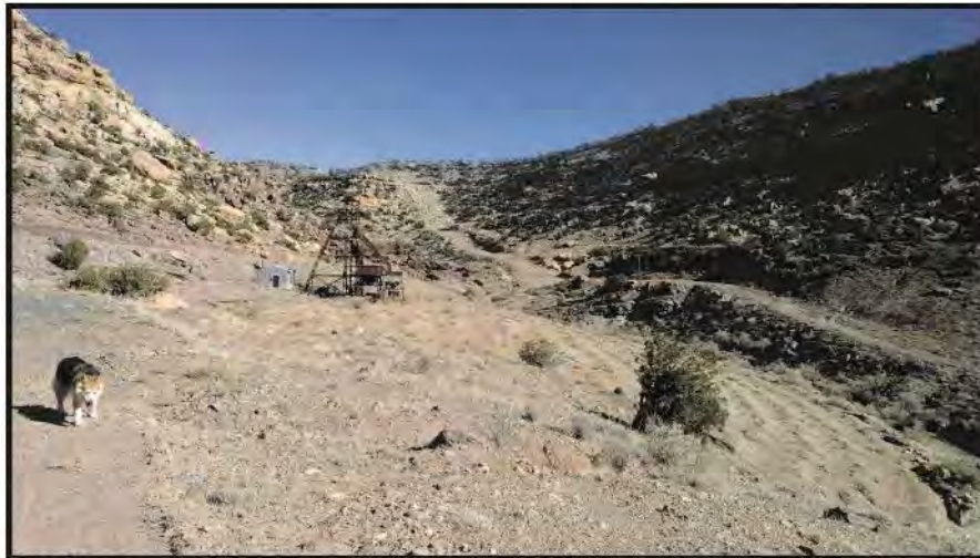
Figure 8: East overview of Burro No.7, with well-preserved headframe, hoist house, and ore bins. The waste rock dump has been partially reclaimed with divots but approximates its original footprint and profile. The entire complex, including the dump, is contributing, and will be avoided by the current sediment control project.
