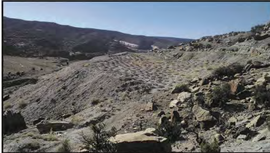
Figure 5: View southwest across Burro No.3's waste rock pad. The top-surface was divoted for reclamation decades ago and is a non-contributing portion due to loss of originality. But overall, the pad is a contributing element of the landscape because it retains its original footprint and profile, and from afar, appears similar to how it did when the mine operated.
