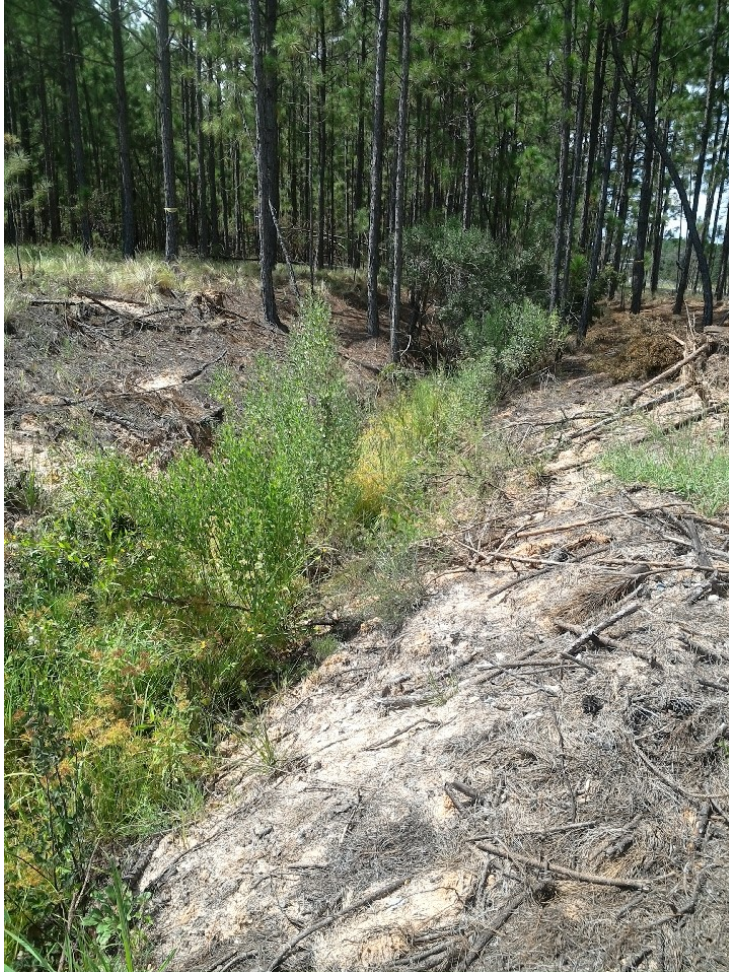
Wet Ditch East End Looking West
