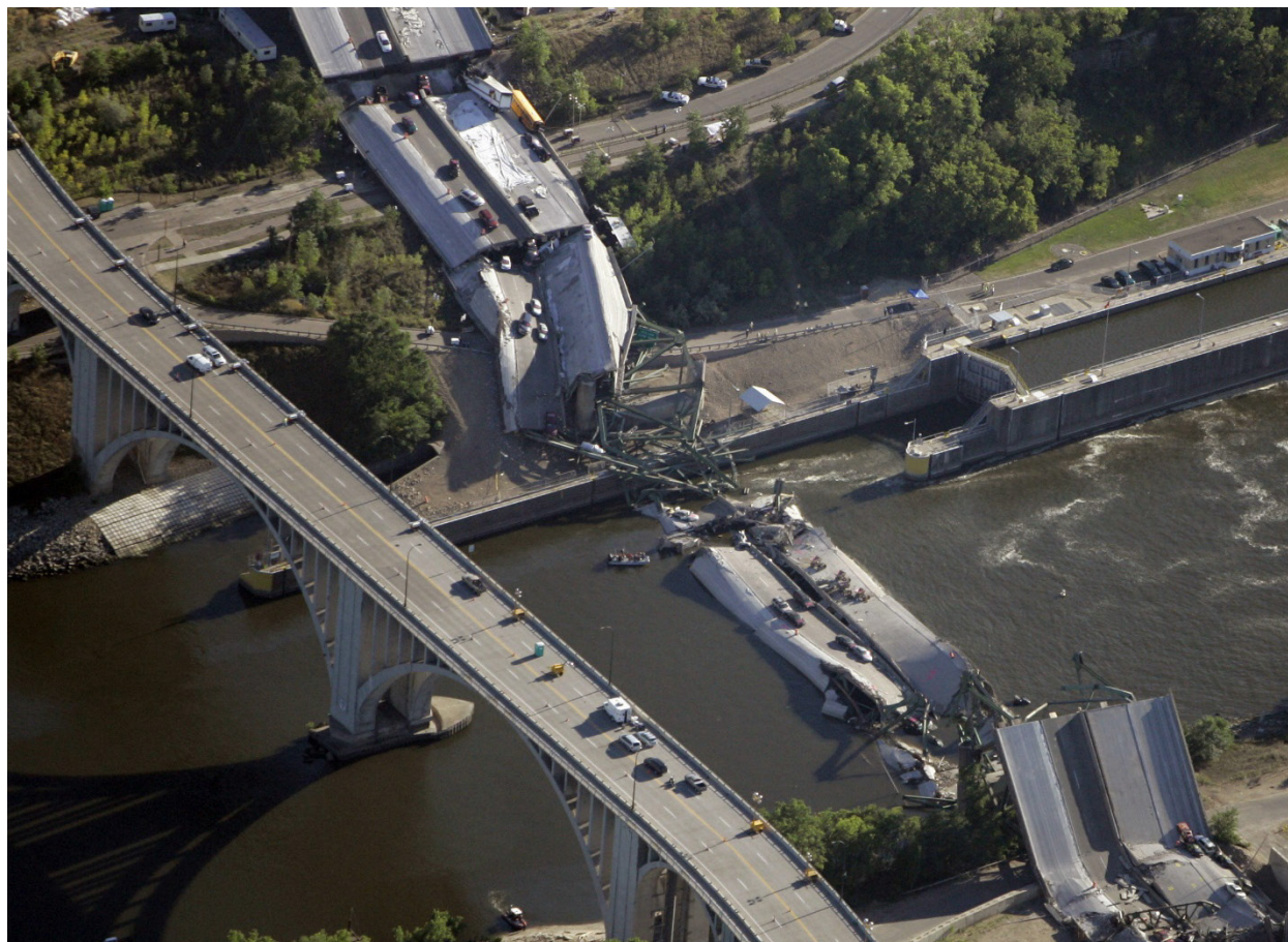
Figure 4. Minneapolis bridge collapse in 2007 8
