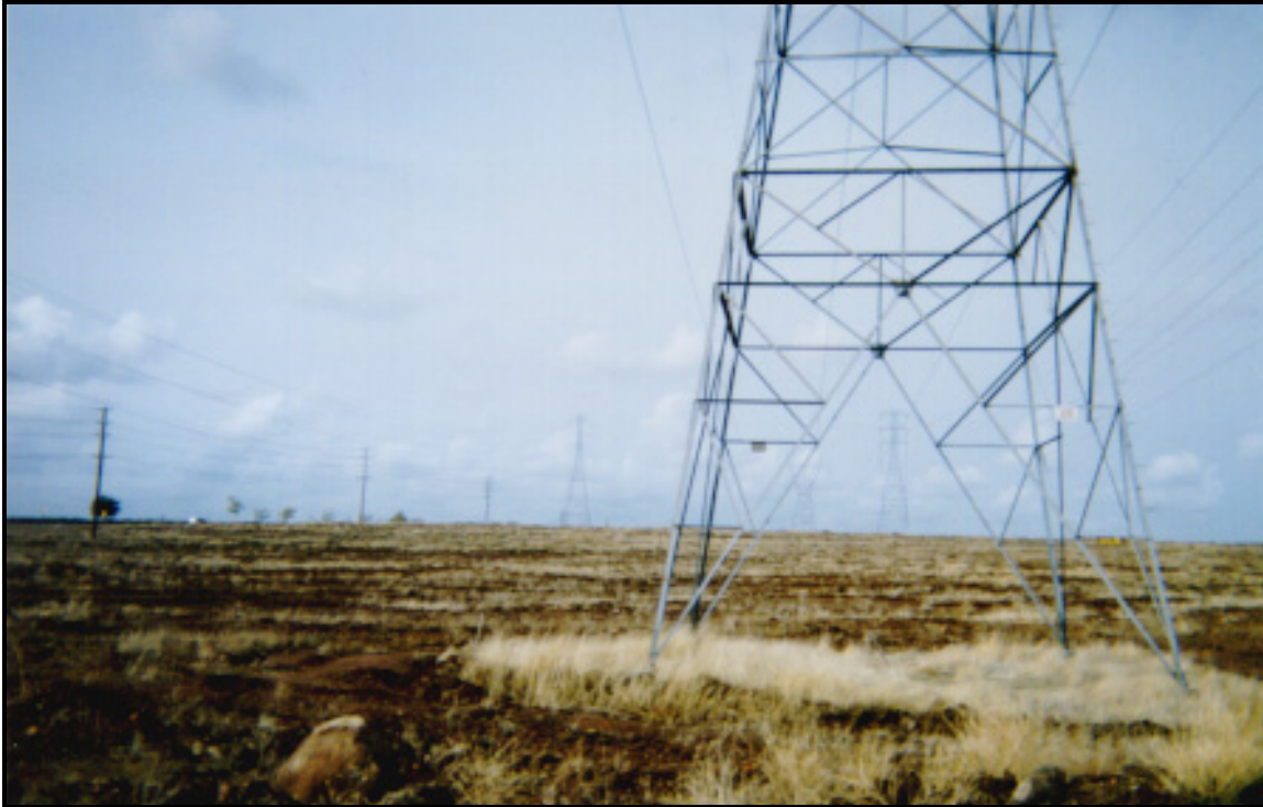
Figure 3-1. Example of Untilled Agricultural Land under Tower
