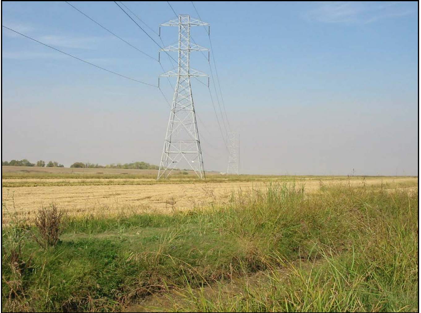
Figure 1-3. Example of Double-Circuit Tower
