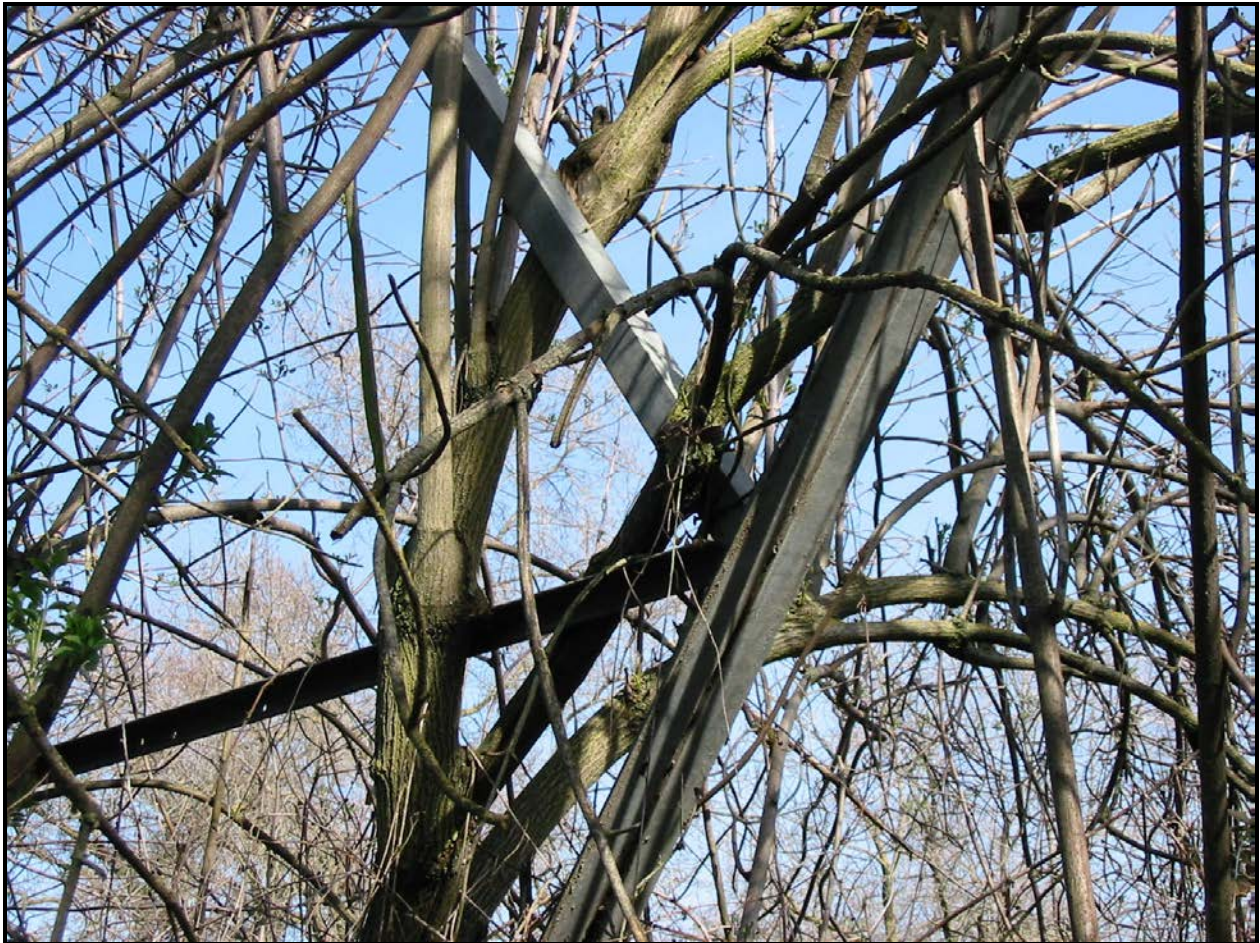
Figure 3-2. Elderberry Causing Stress to Tower 9/4, Elverta-Hurley Transmission Line
