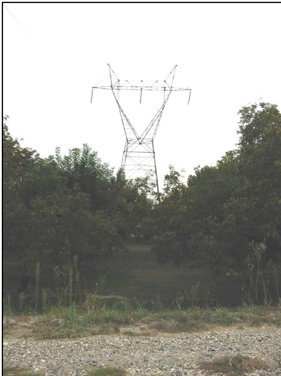
Figure 1-5. Example of Single-Circuit Tower
