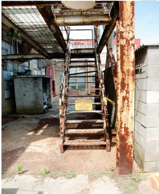
Figure 1-7. Unsafe and Unusable Emergency Stairs
