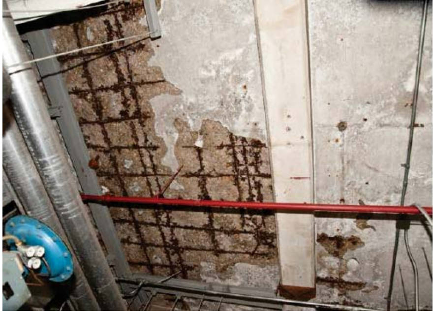
Figure 1-6. Spalling Ceiling of Fan Room 1
