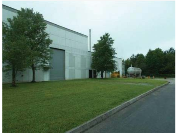
Figure 3-9. Access drive with high bay and Aboveground Storage Tank
