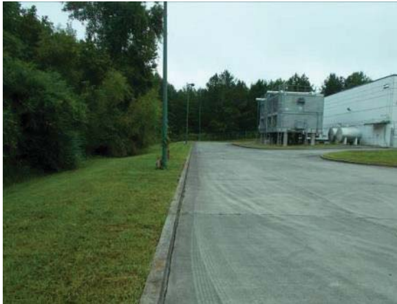
Figure 3-8. Western access drive with cooling towers and Aboveground Storage Tanks
