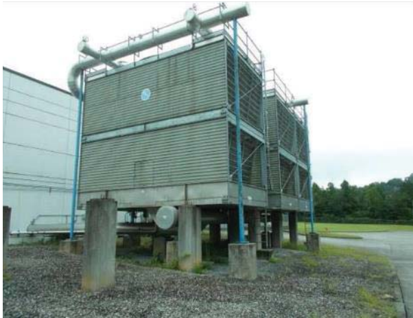
Figure 3-25. Cooling Towers
