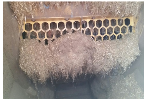
Plugged screen in a grinder [2]
