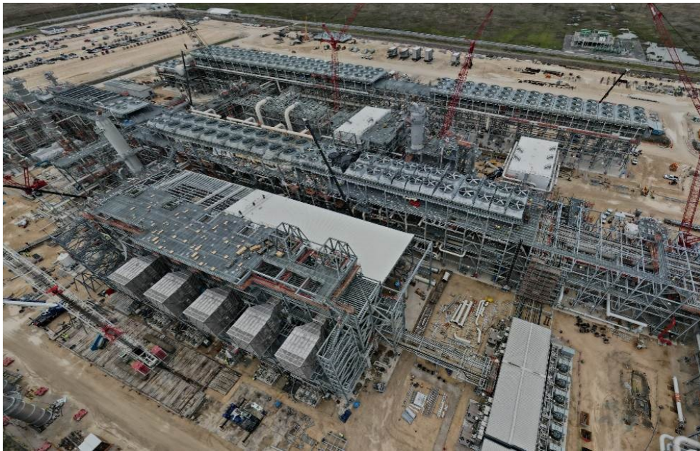
Progress at Train 6 facing Northeast
