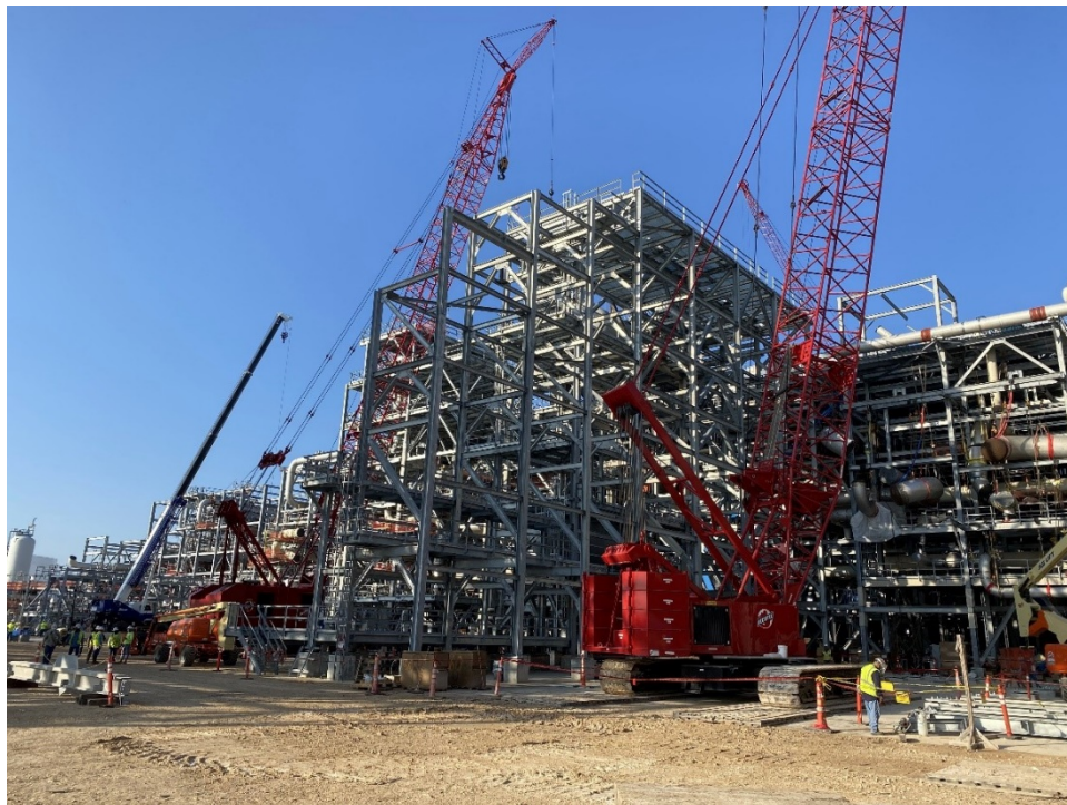
Steel Erection in advance of setting Ethylene Cold Box
