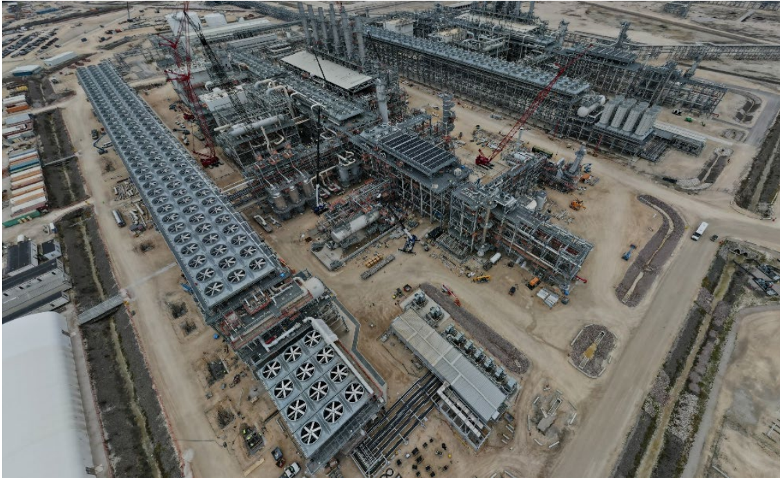
Progress at Train 6 facing South
