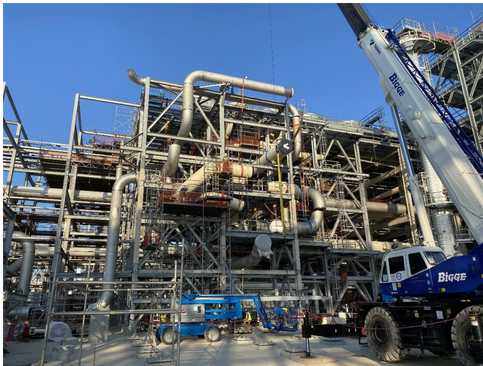
Pipe Installation prior to setting of Methane Cold Box
