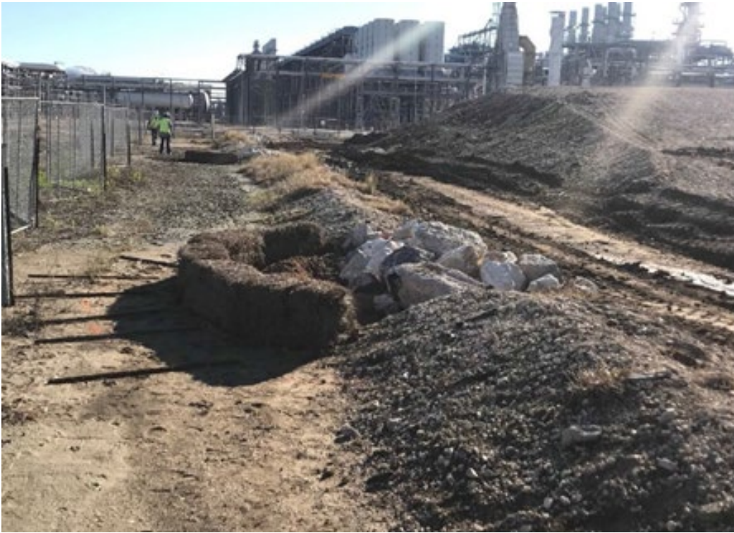
Installation of additional sediment controls (hay bales) in Laydown 14
