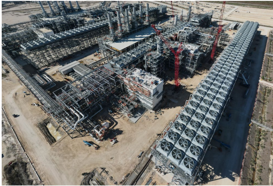
Progress at Train 6 facing North
