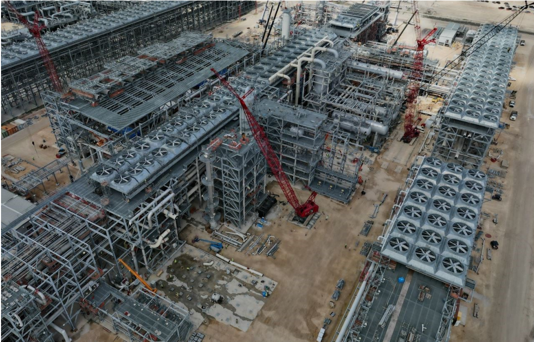
Progress at Train 6 facing North
