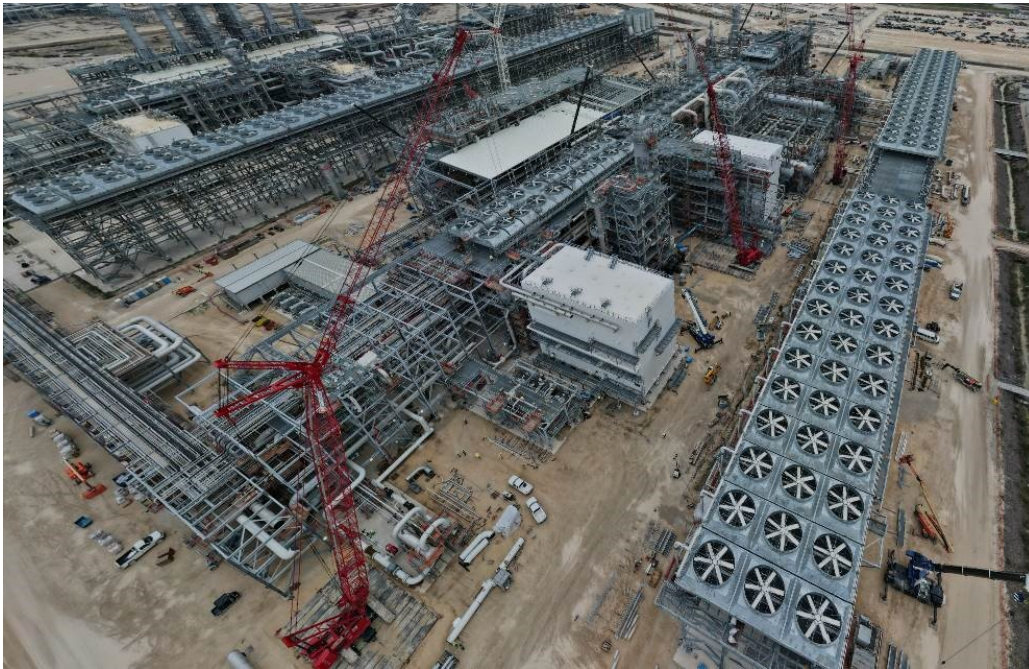
Progress at Train 6 facing North
