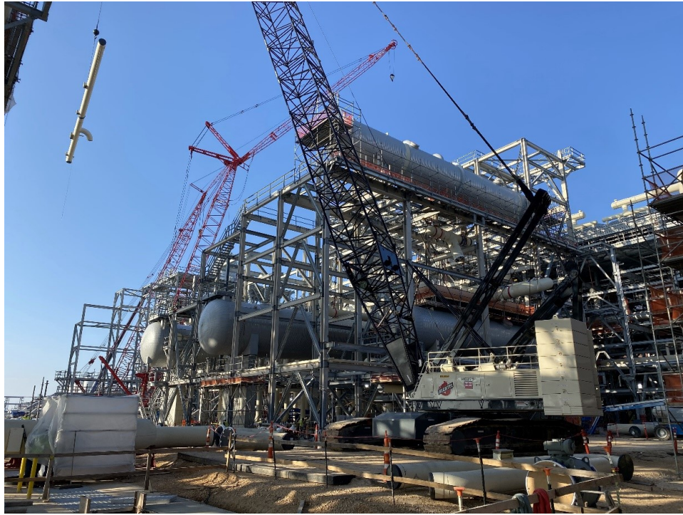
Progress at Propane Refrigeration Area
