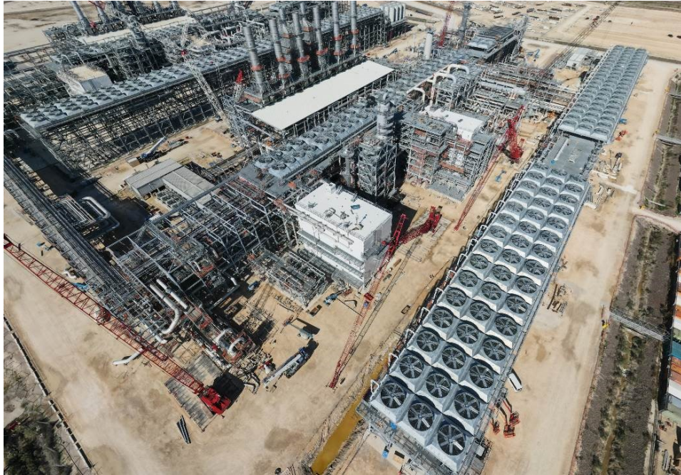
Progress at Train 6 facing North
