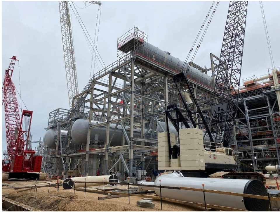
Progress at Propane Refrigeration Area
