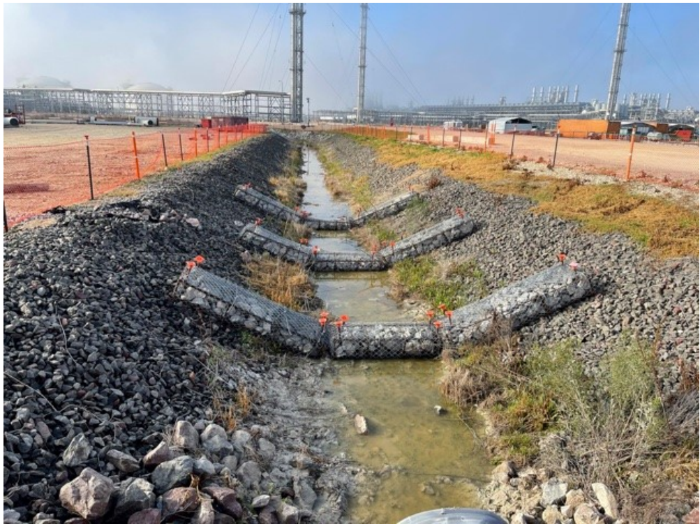
Gabion baskets installed in Outfall 004 drainage at Laydown 18
