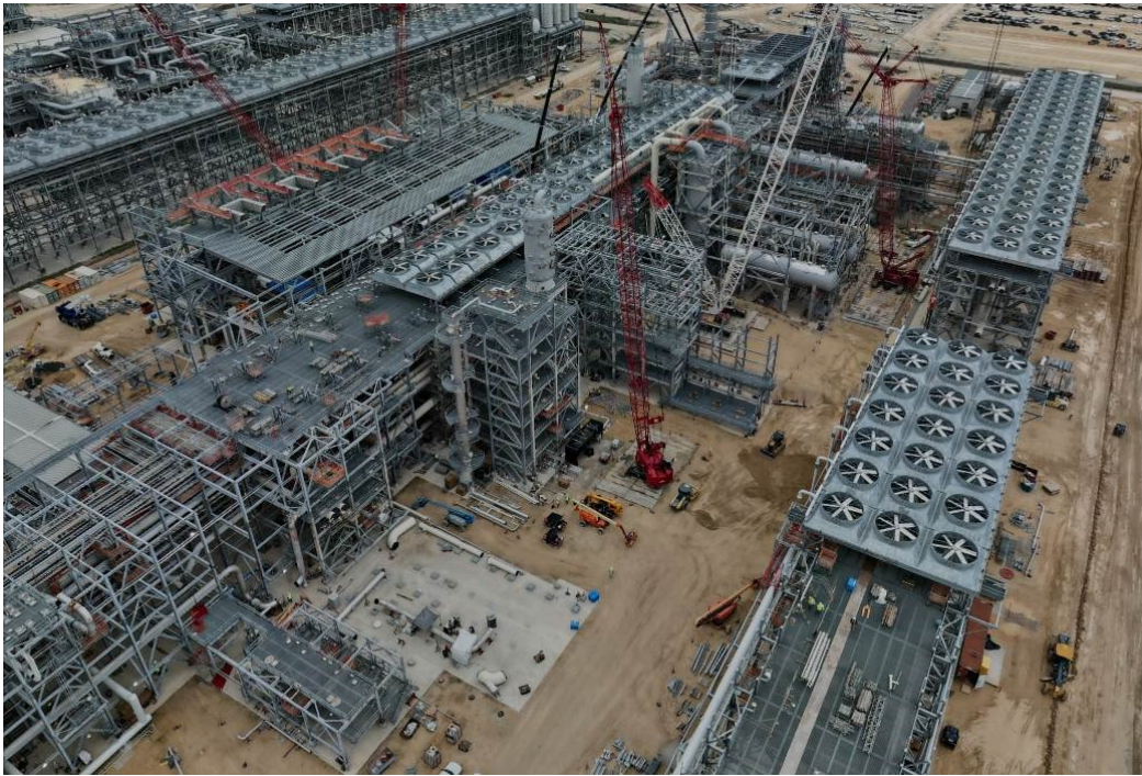
Progress at Train 6 facing North
