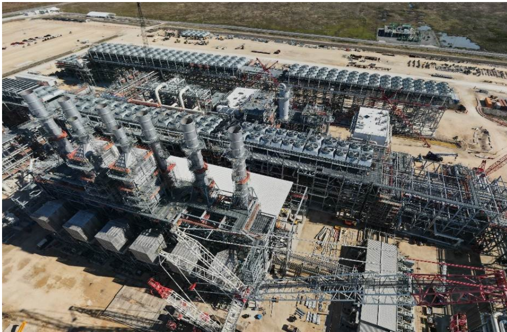
Progress at Train 6 facing Northeast
