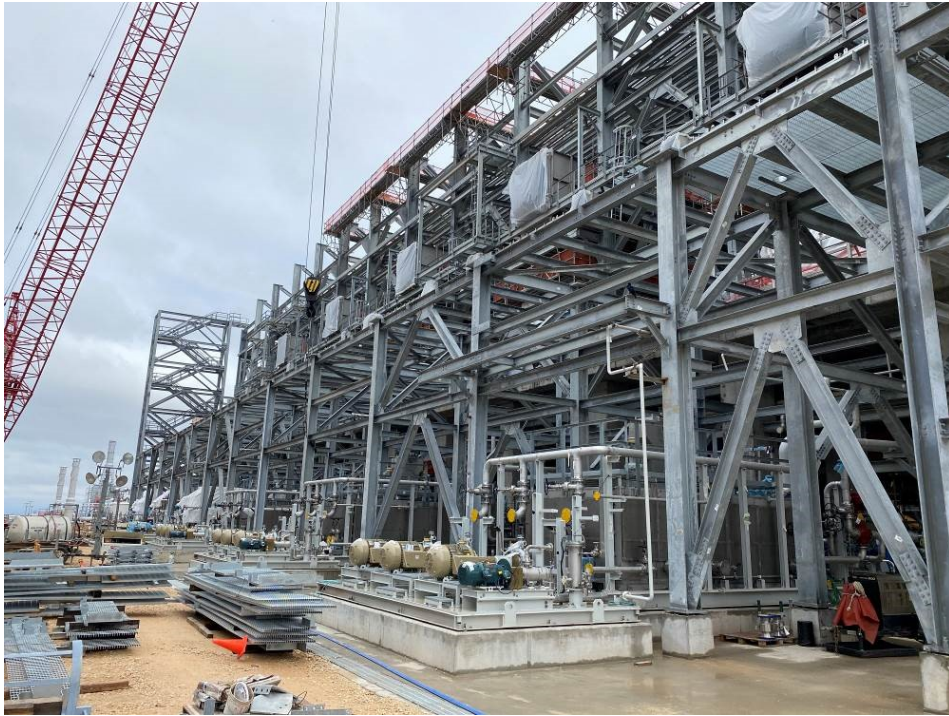
Progress on Filter House Steel at Compressor area
