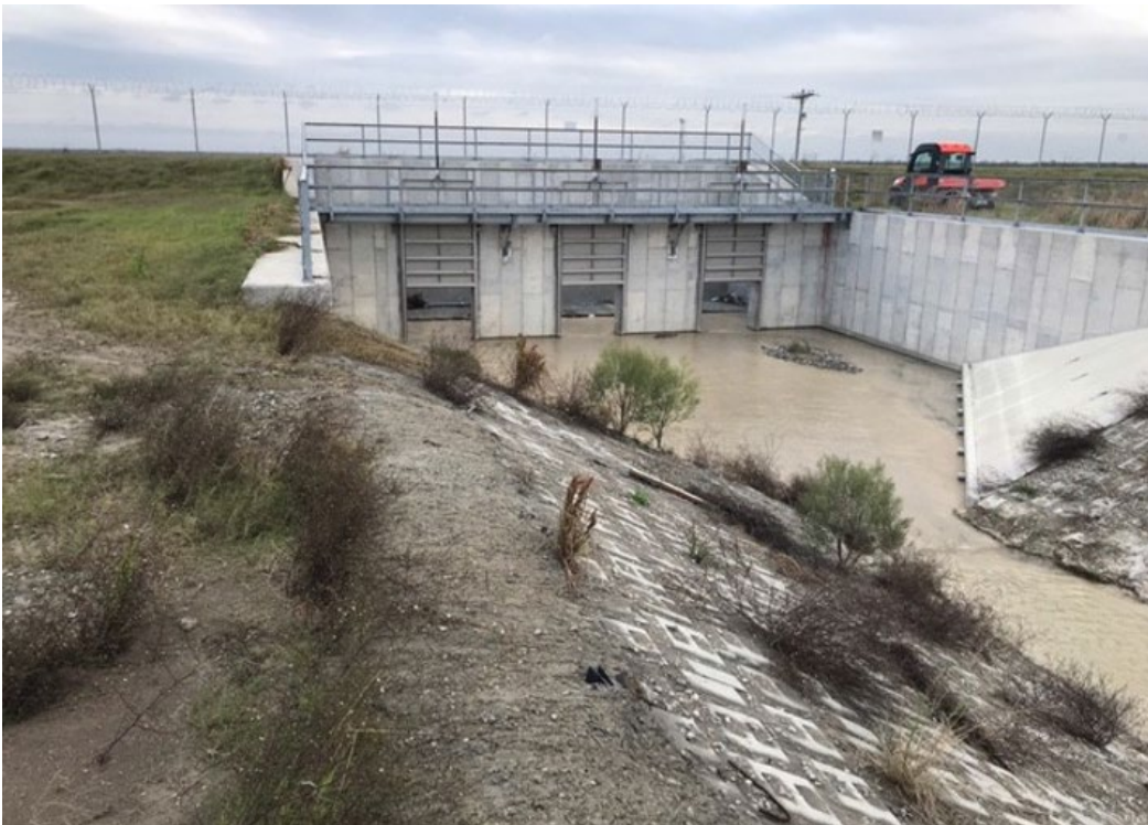
Observation at Outfall 004 during virtual construction inspection
