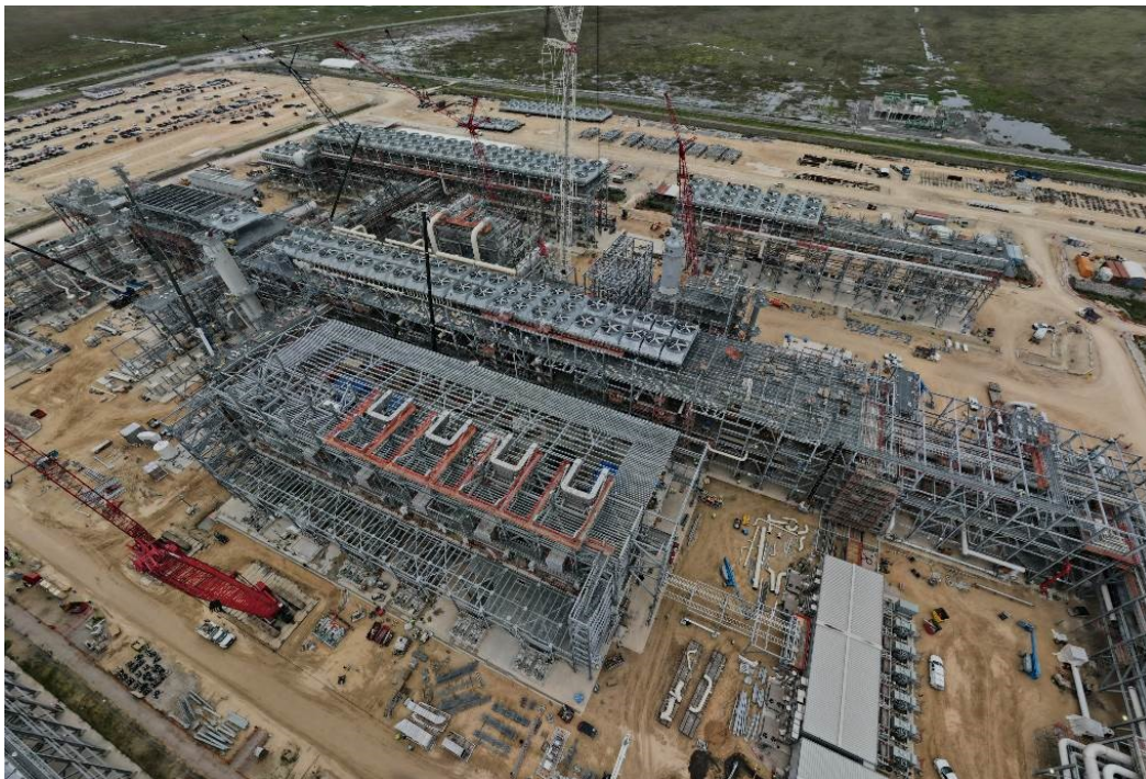
Progress at Train 6 facing Northeast
