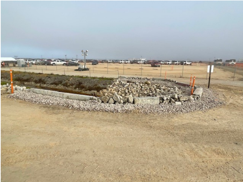
Rock check dams installed around storm water drainage in Laydown 18
