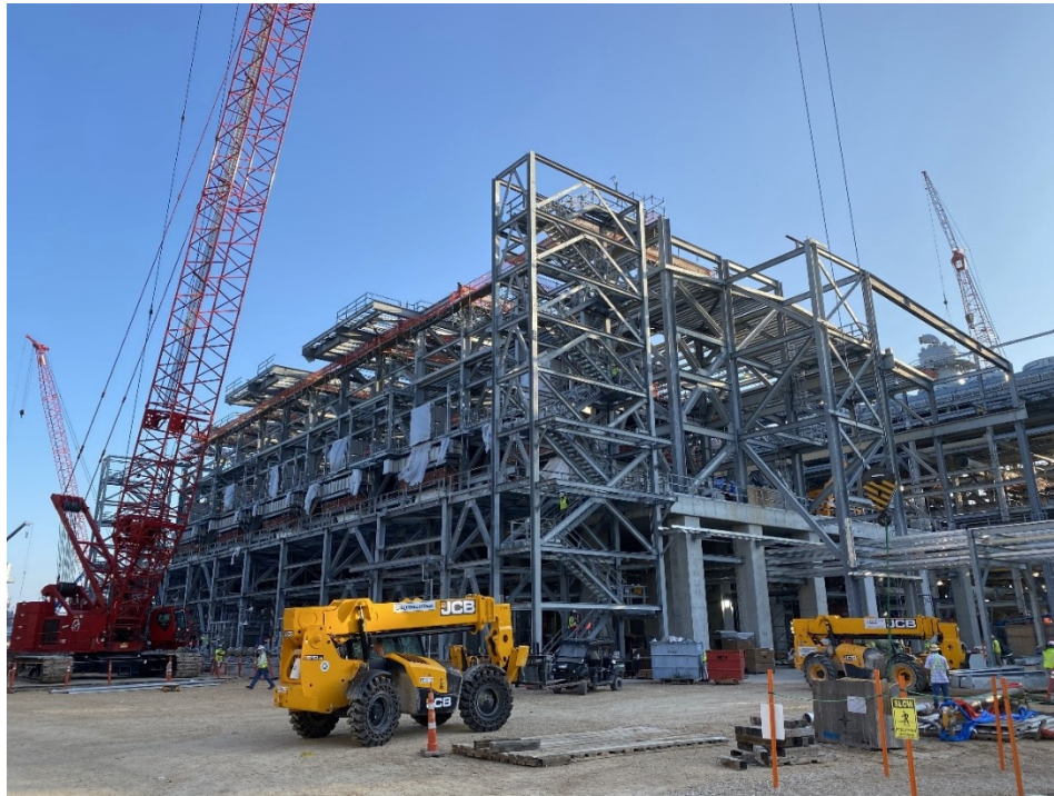
Upper Floor Steel Placement at Compressor Area
