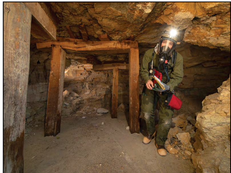
Aaron Sidder from Bat Conservation International passes cap and post timbers en route to the mine portal. (Photo by Bill Hatcher/BCI.)
