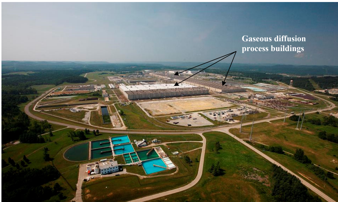
Figure 1.1 The Portsmouth Gaseous Diffusion Plant. (looking from the north-northeast towards the south-southwest)
